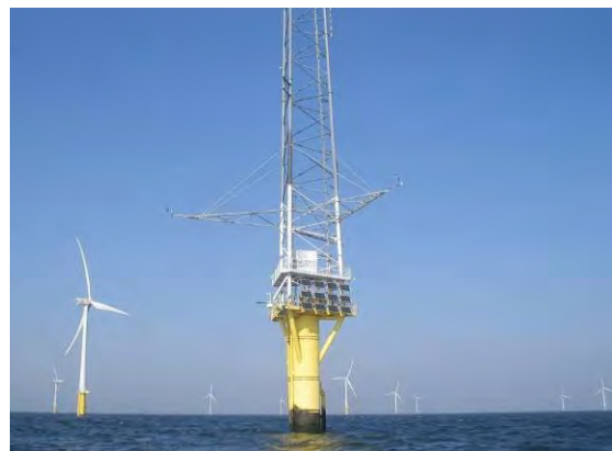
The MERLIN system was re-installed on a Monopole in 2006 as an avian monitoring system for the windfarm
