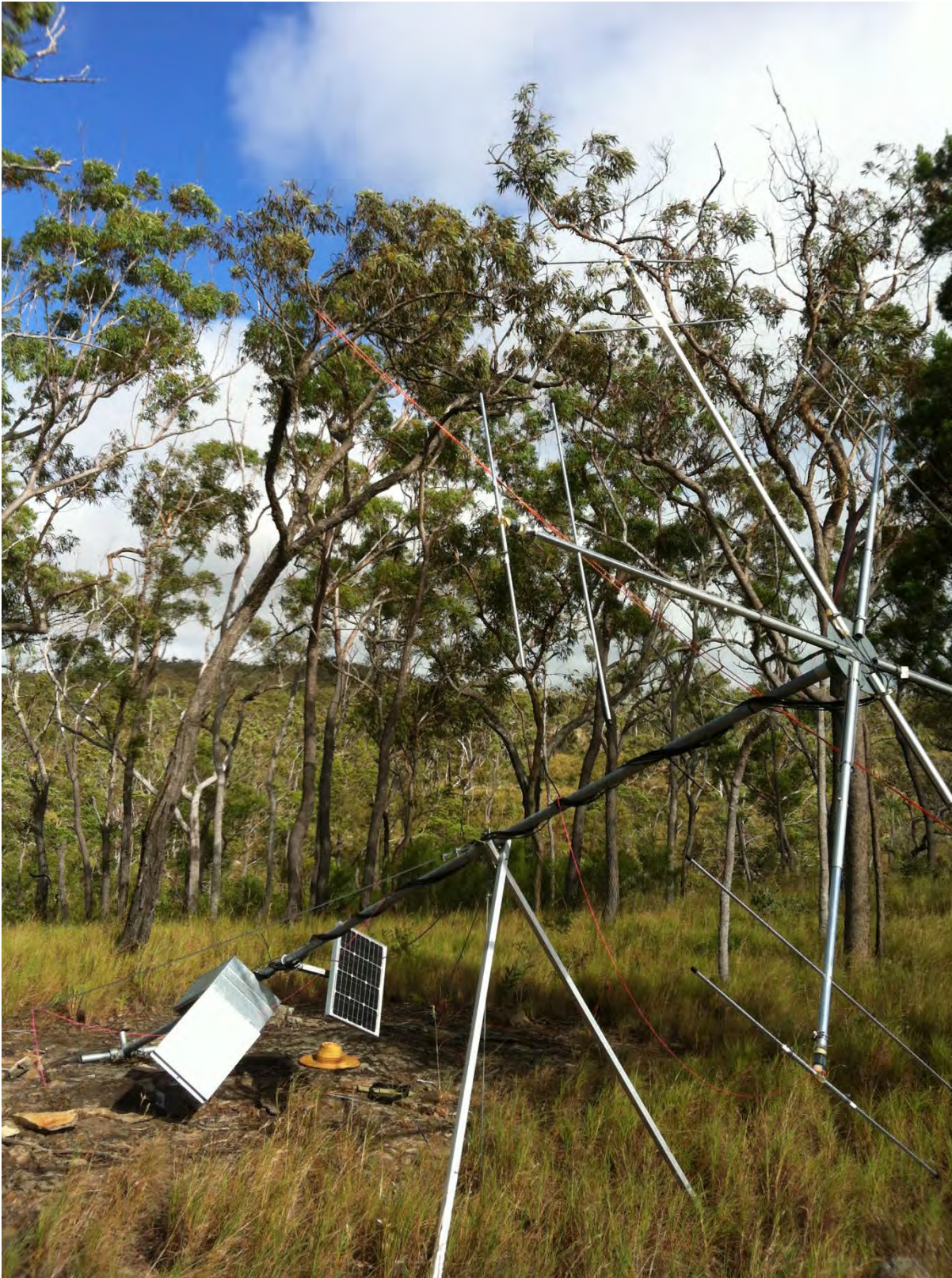
Plate 1 ARTS Tower Prior to Erection
