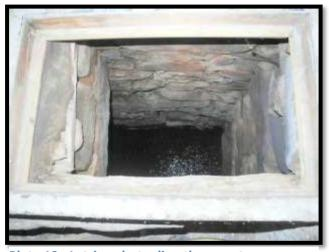
Plate 19 - Latrine chute directly over stream.
