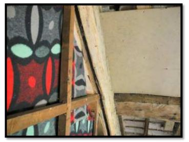
Plate 35 - mortise on principal rafter truss 2
