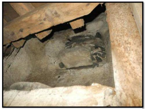
Plate 22 - Blocked cross passage door. This doorway appears to have been reduced in size leaving a small window, which can be see has been filled in roughly with stones.
