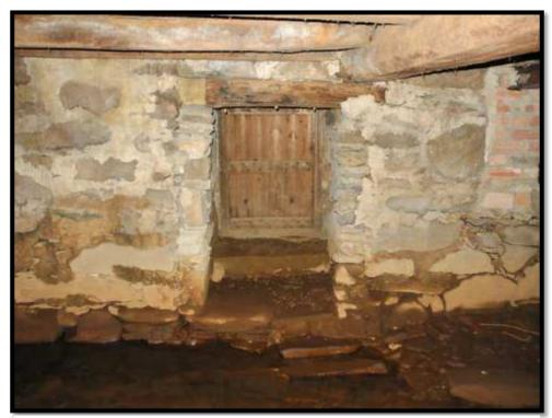
Plate 20 - Basement - external door, remodelled doorway south gable
