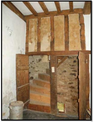
Plate 26 - Timber framed partition with doors to stairs.
