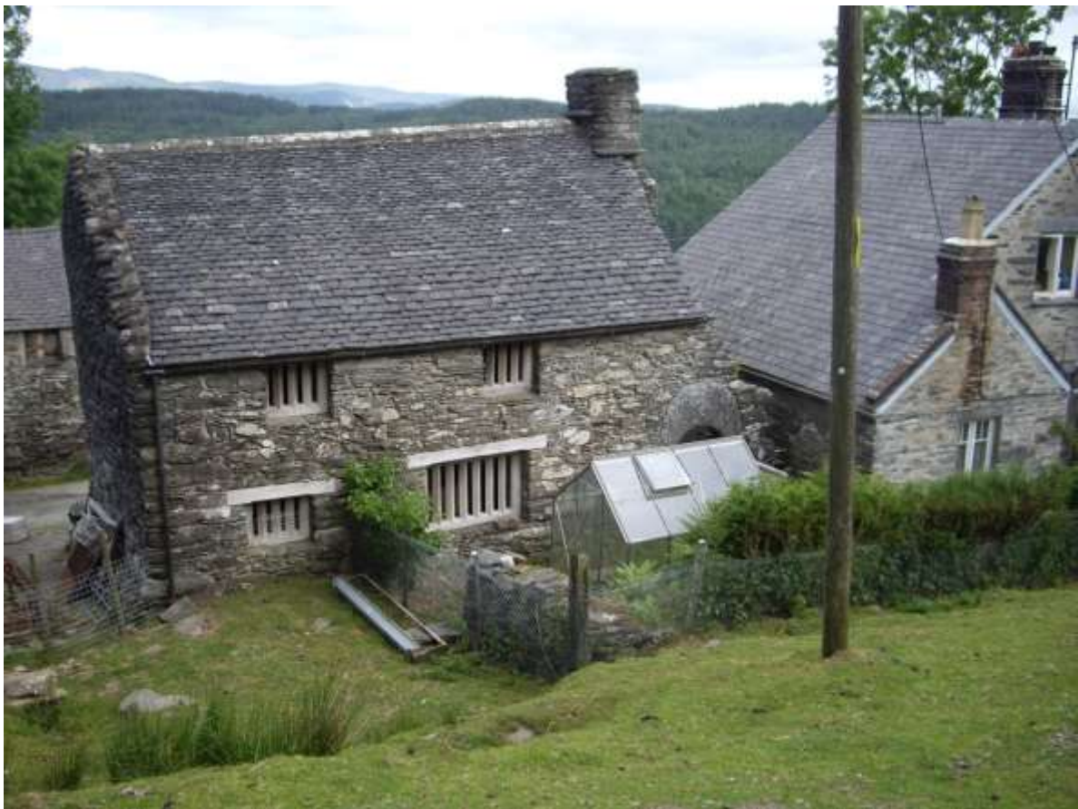
Fedw Deg from rear showing restored windows & doorway (just above greenhouse)
