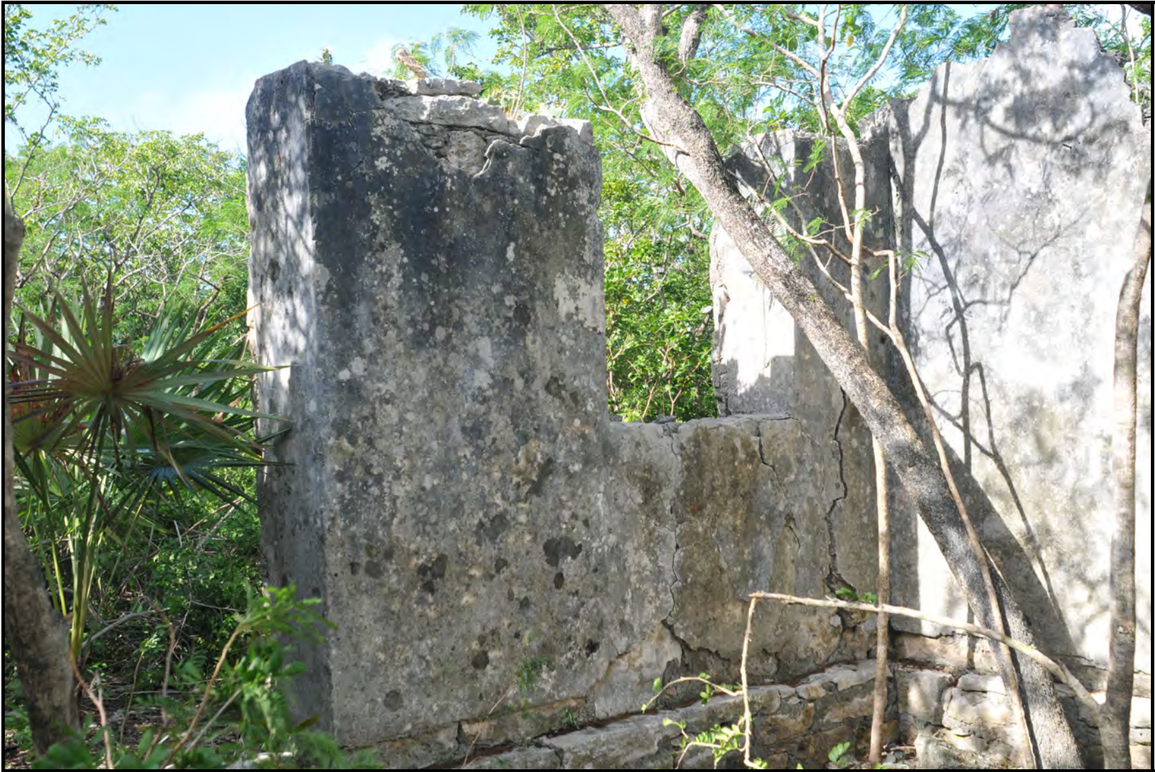
Plate 16. Structure 6(a). View, interior southwest corner.
