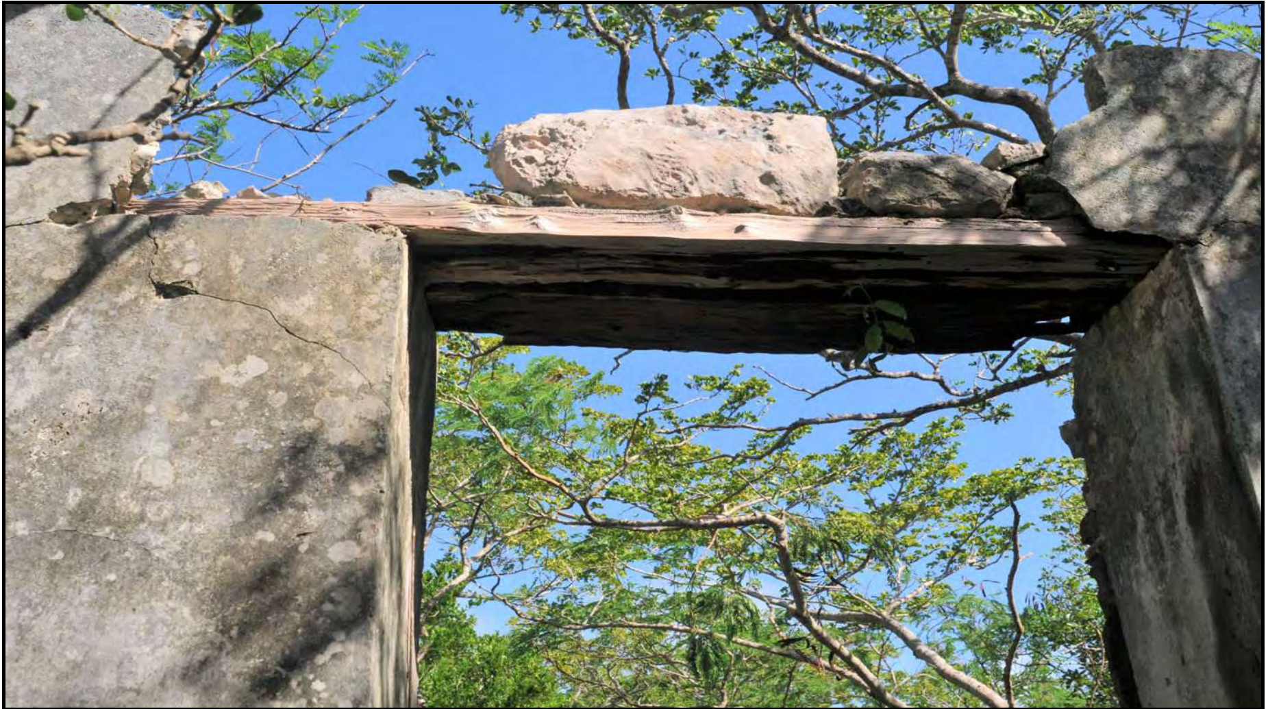
Plate 18. Structure 6(a). East facade, detail of lignum vitae lintel over window opening, interior view showing bearing.
