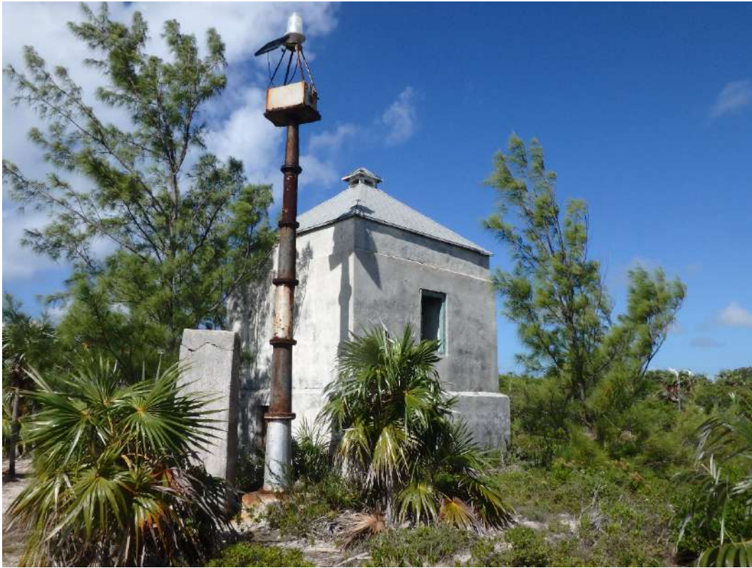
Existing Lighthouse Structures
