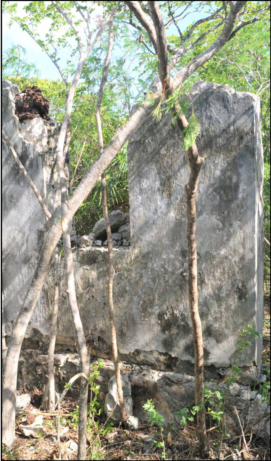
Plate 13. Structure 6(a). Detail of northeast exterior corner.
