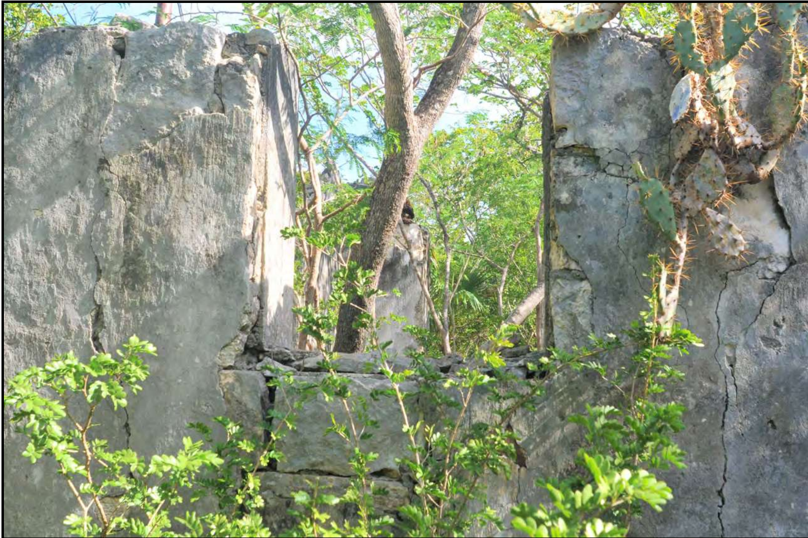
Plate 15. Structure 6 (a). Detail of west facade showing cut stone masonry around window opening.
