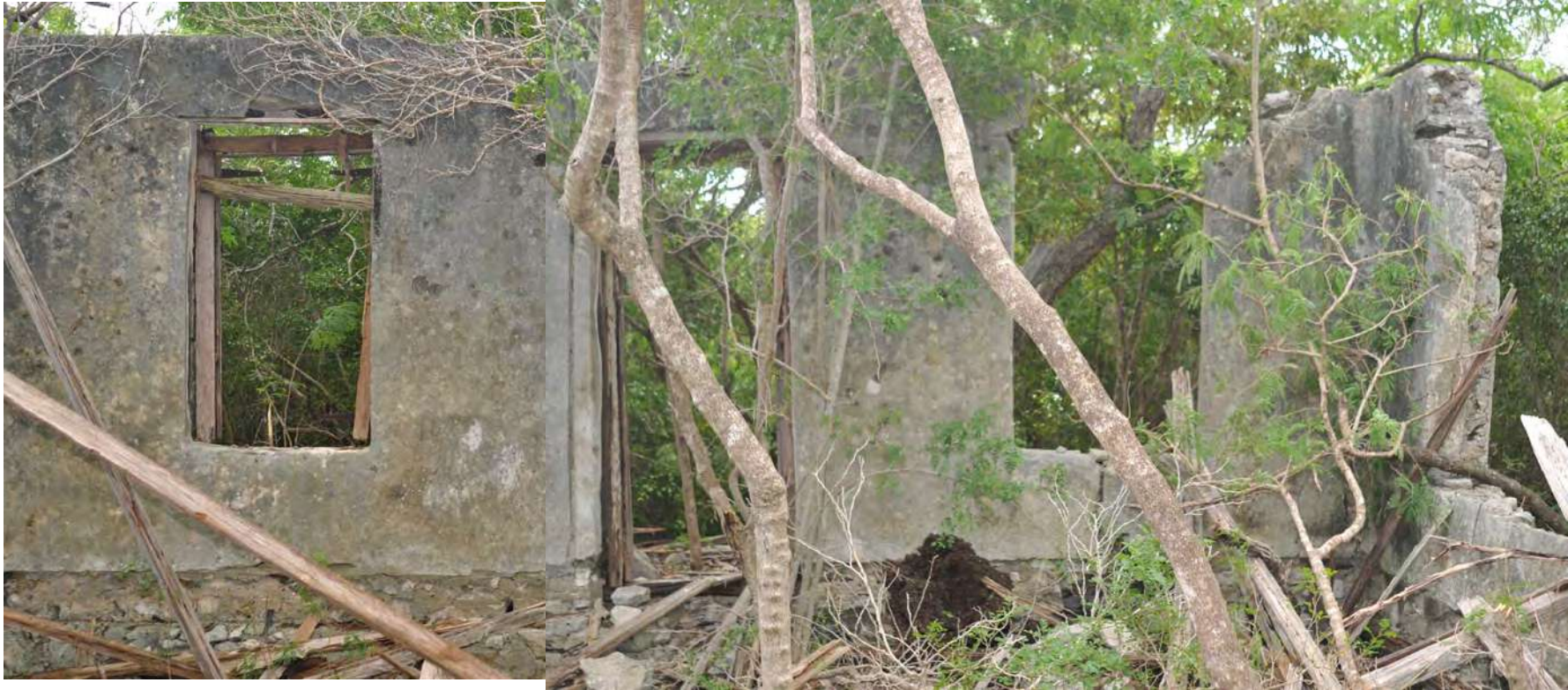
Plate 9. Structure 5. South facade, interior view (composite).
