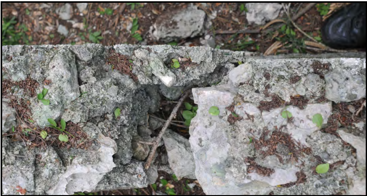
Plate 4b. Structure 2, south facade, plan view showing tabby and rectangular post hole.
