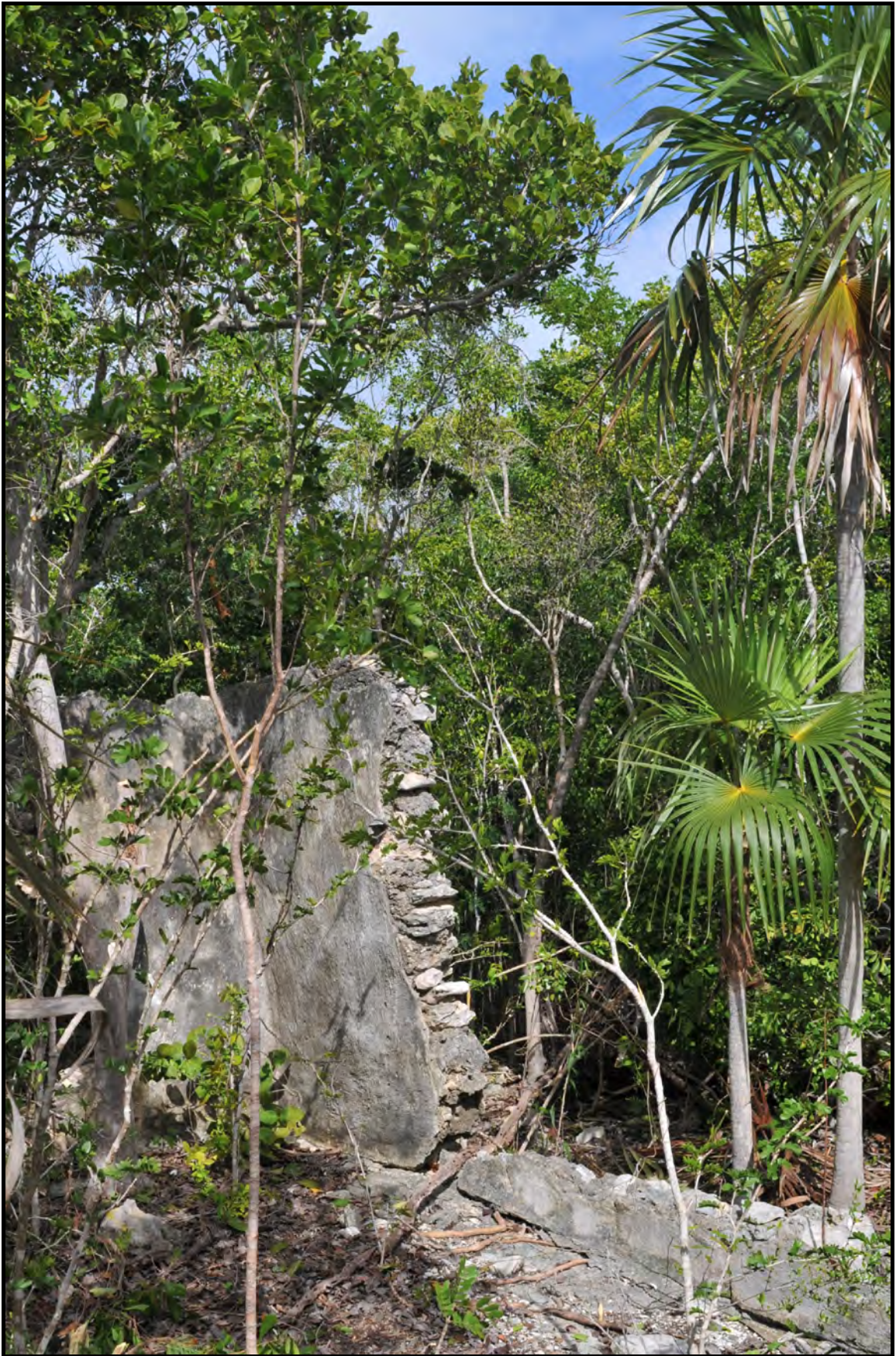
Plate 8. Structure 4. Detail of northeast corner, interior view.
