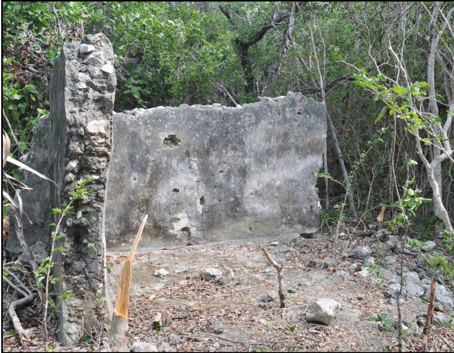
Plate 7. Structure 4. Interior view looking north showing cross wall (left) and mortar floor.
