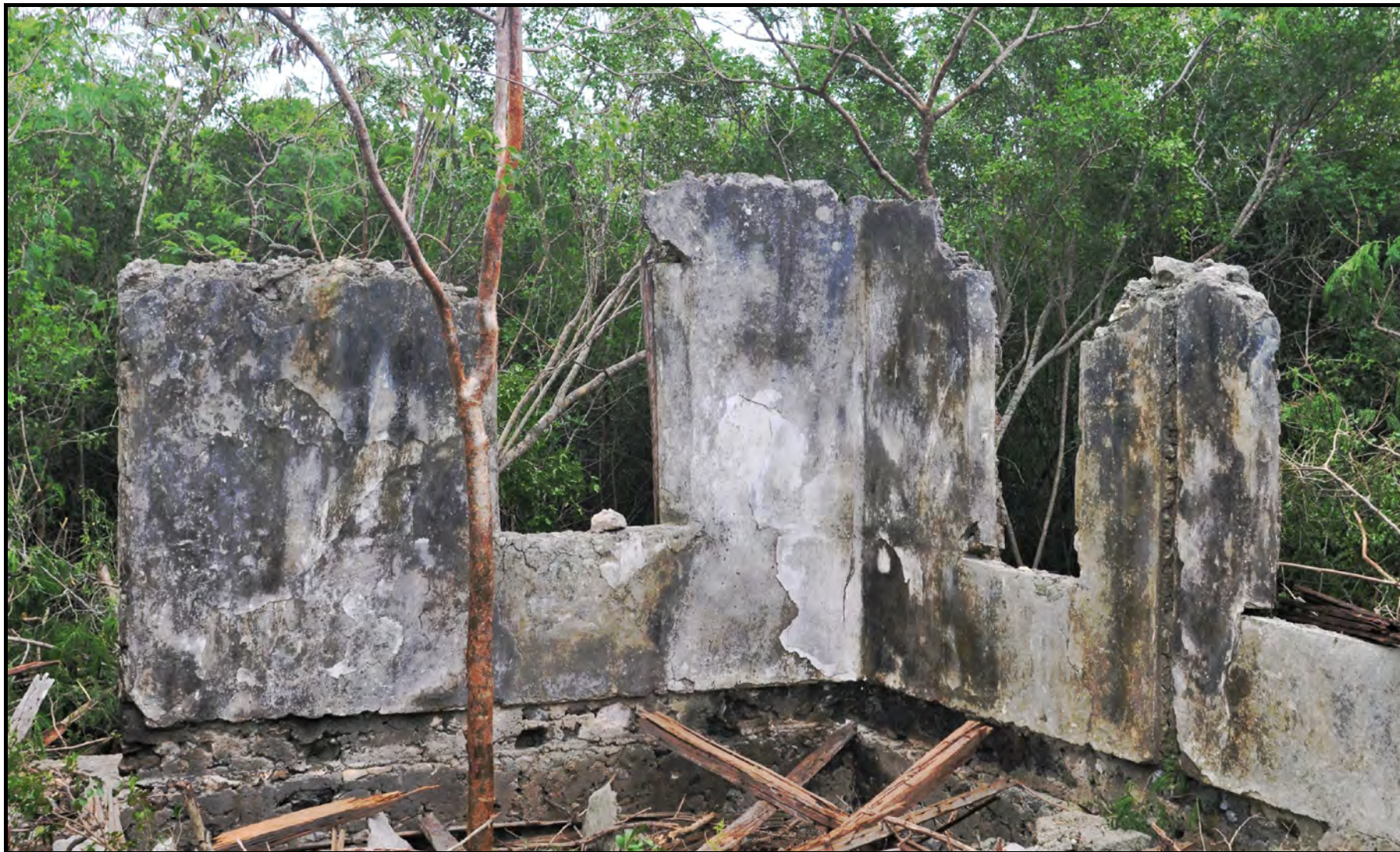
Plate 2. Structure 1, view of interior southeast corner.
