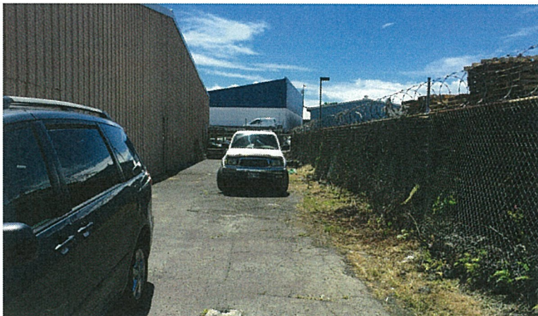
REAR OF BUILDING #2
