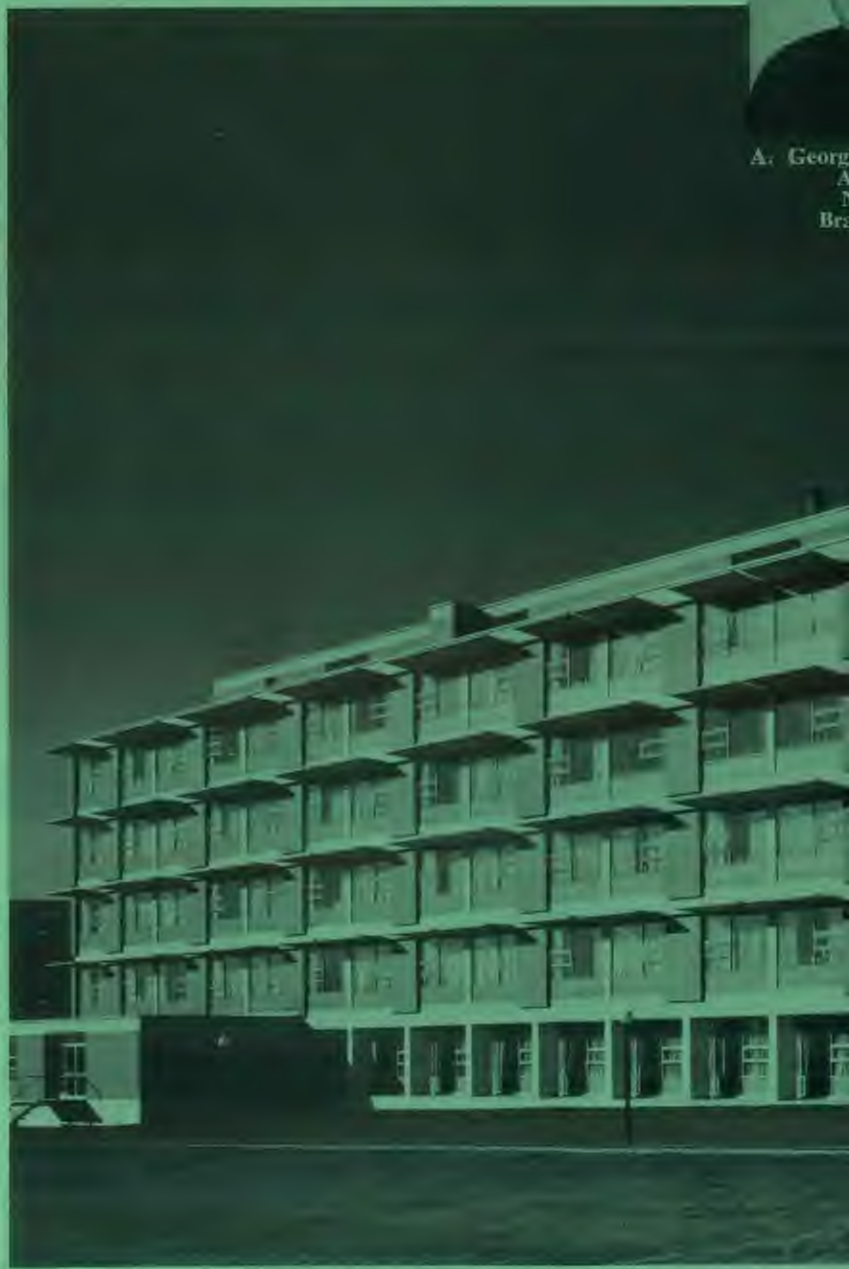
Extended view of eastern elevation housing surgical, medical, and other departments of the Branson Hospital.
