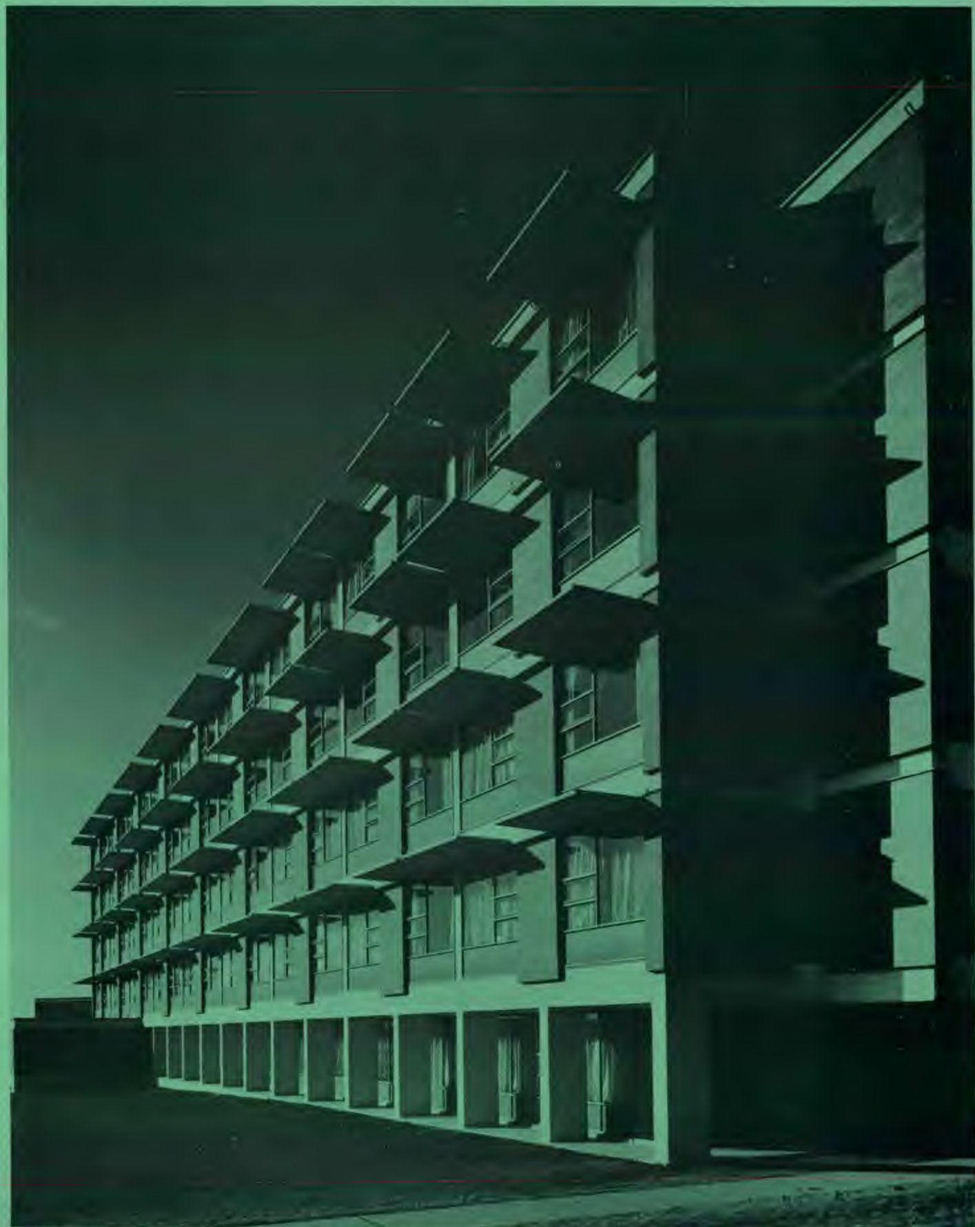
The east elevation showing Branson's new 335-bed wing. Architectural originality is seen implicit in the ornamental cantilever canopies which deflect heat and reduce sun glare.
