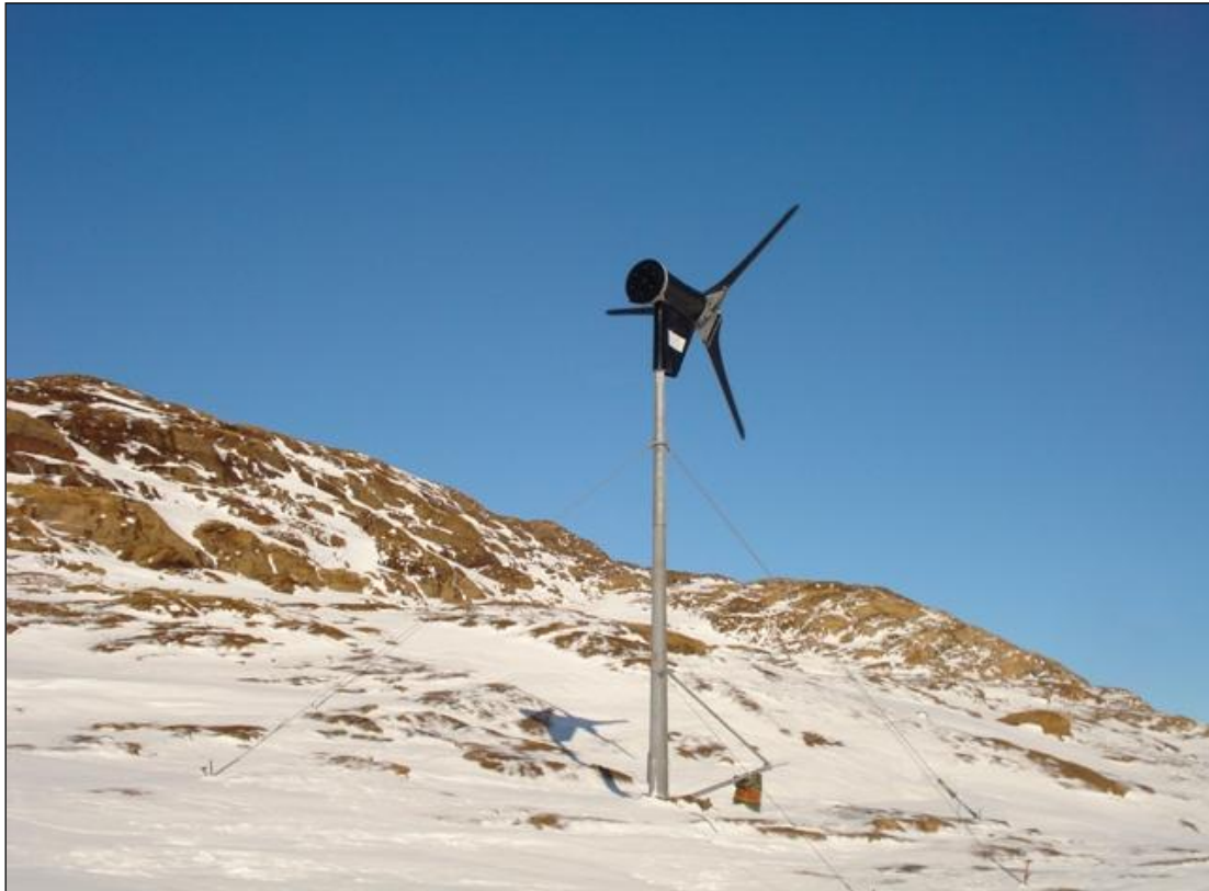
FIGURE 13 : WIND ENERGY GENERATOR (6KW) INSTALLED AT SITE
