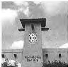
Examples of Building-Concealed Wireless Communication Facilities
