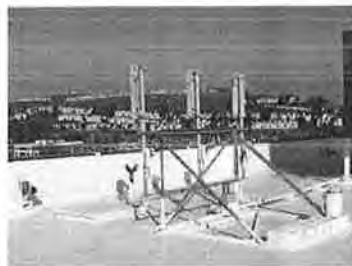
Examples of Roof-Mounted Wireless Communication Facilities
