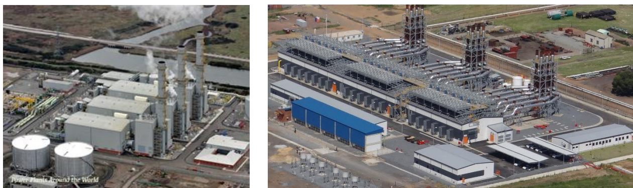
Figure 2: Examples of gas to power plant sites (source: www.industcards.com and www.wartsila.com )
