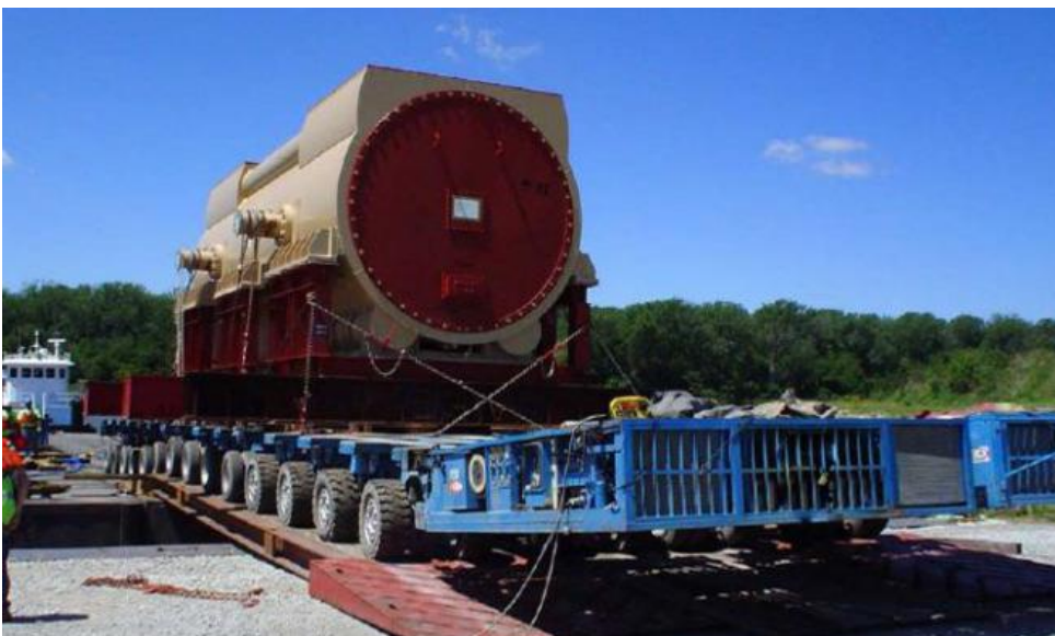
Figure 5: Example of large equipment being offloaded from a barge. Note the levels of the ramp, the barge and the jetty (source: SUBTECH)
