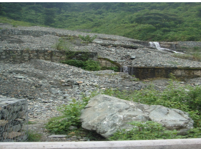
Debris deposited on check dam
