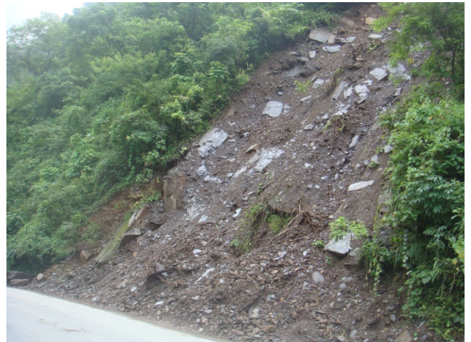
Landslide along the road.
