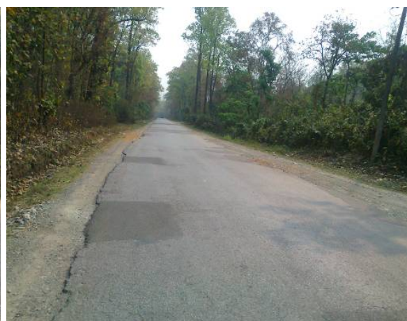
Wildlife crossing area at Ch 7+600
