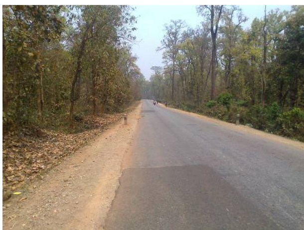
Wildlife crossing area at Ch 3+550
