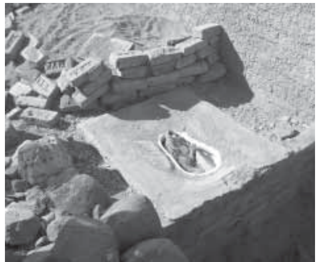
Abandoned demonstration toilet, Watephal
