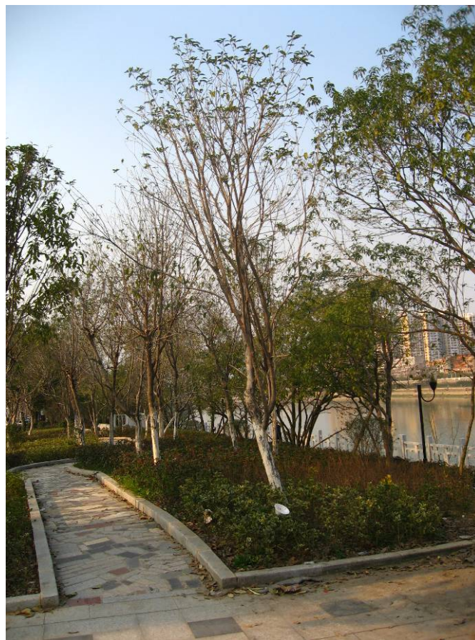
Figure 15: Current Situation of Constructed Section of Jingdezhen Flood Control Project (near Zhushan Bridge)
