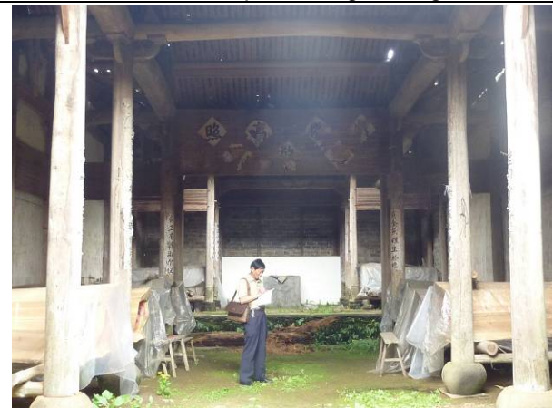
General Ancestral Temple of Yu's Ancestral Temple in Qingxi Village – Cultural-relic and Historic-building Specialist Working on Site
