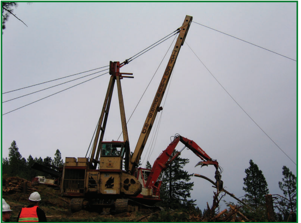
Figure 8.15. Yarder extracting whole trees or processed logs on steep ground (>35 percent slope).
