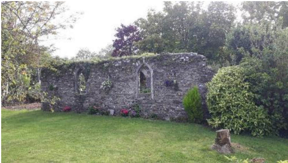
Photograph 78: South wall of St Patricks Chapel Garrafrauns
