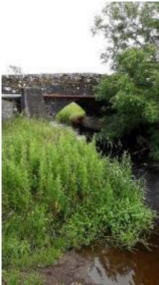
Photograph 167: Killuney/Addergoole More Bridge
