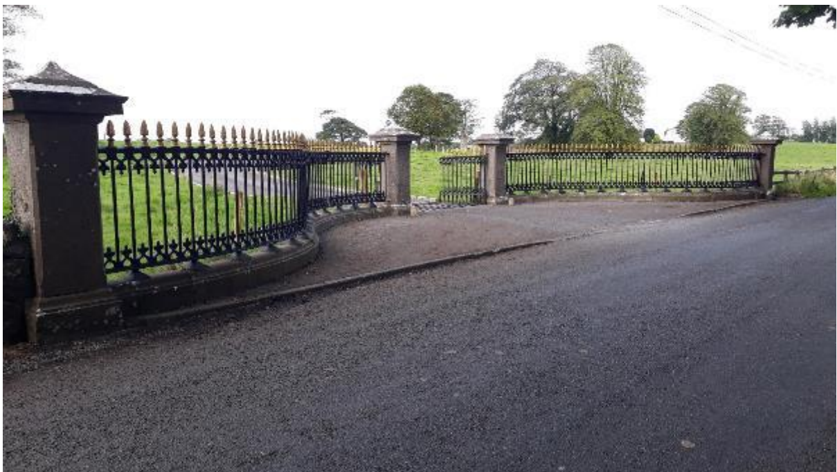
Photograph 120: Gates to former Joycegrove House
