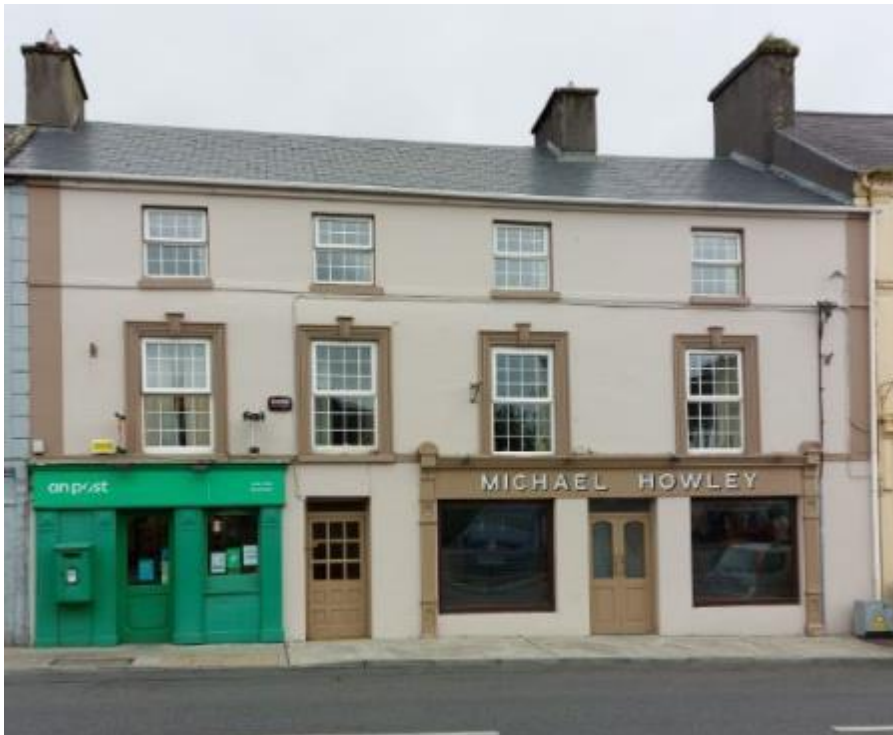
Photograph 146: Traditional shopfront with hand painted name plate and modern post office shopfront set into ground floor of house. Second floor windows with decorative channelled architrave with central pediment.
