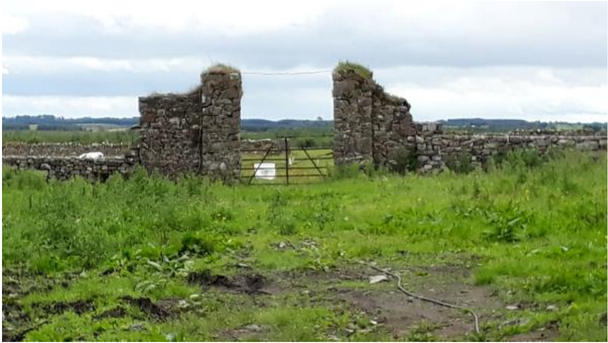
Photograph 116: Remains of boundary walls and gateway at former Woodfield House.
