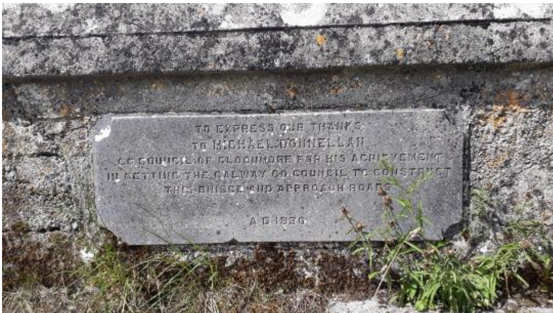
Photograph 172: Dedication stone on the Cloonmore-Slieve Bridge dated 1930
