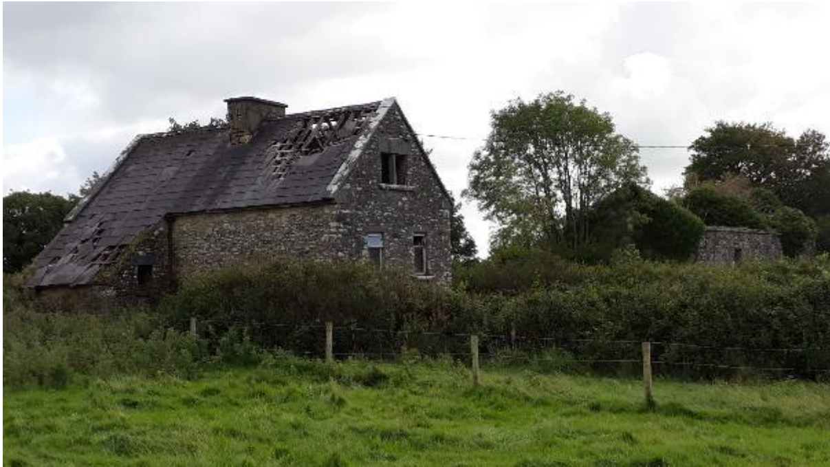
Photograph 121: House and stable block at Curraghaun
