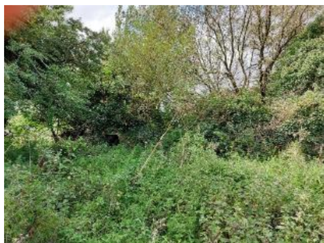
Photograph 150: Ruins of Millers House at Garrafrauns mill site
