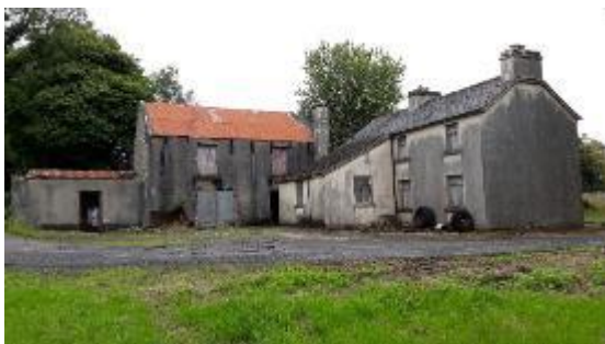
Photograph 160: Remaining two storey storage shed at Gortaganny Mill
