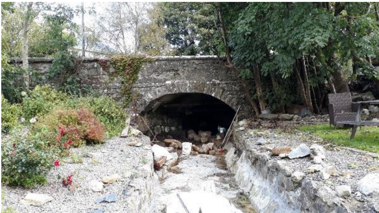
Photograph 169: Clooneen Mill Race Bridge
