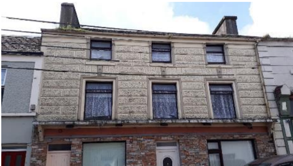
Photograph 149: Plaster decoration on lined and rendered façade of upper floors of house in Castle St. with remains of fascia of a traditional shopfront over ground floor.
