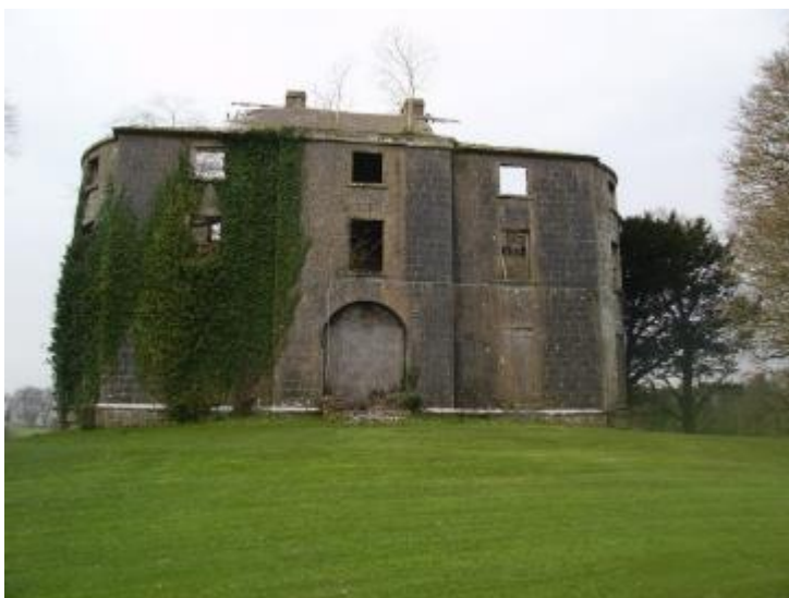
Photograph 118: Dunmore House today
