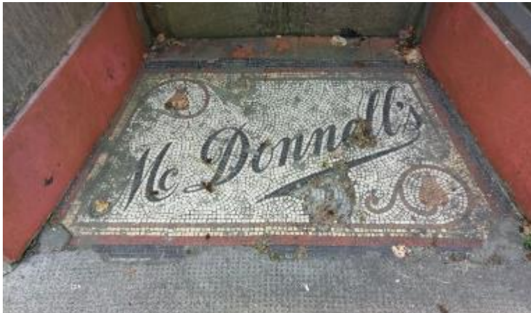
Photograph 143: Mosaic tiled entrance door step Bridge St., Dunmore
