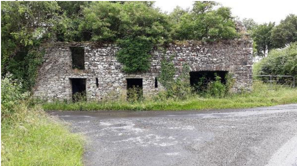
Photograph 158: Attiflynn Mill store
