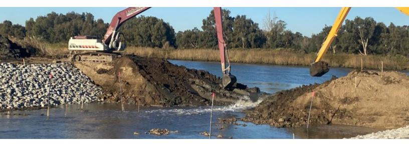
Levee breach in the Montezuma wetlands restoration project. Photo courtesy of the Montezuma wetlands project.
