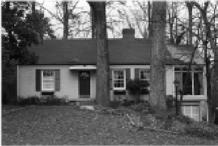
Example from Druid Hills Heights with basement garage.
