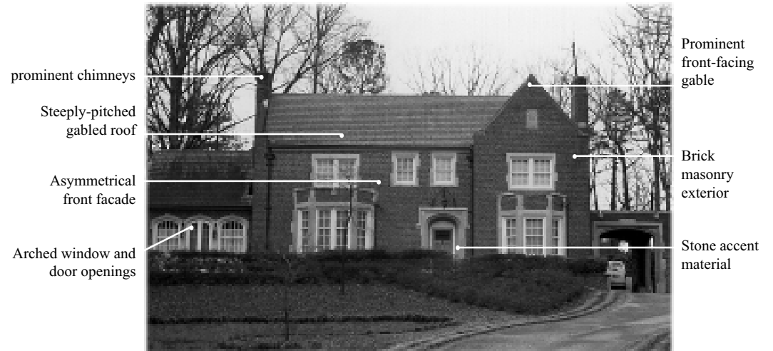
High style example of the English Vernacular Revival style with principal features keyed.
