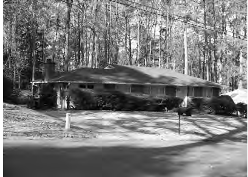
Example of Ranch House type with a low pitched hip roof, Chelsea Circle
