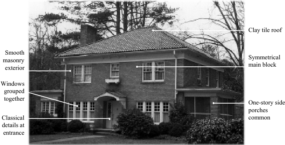
Typical example of the Italian Renaissance Revival style with principal features keyed.
