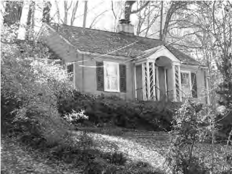
Example of Minimal-Traditional House type with a moderate pitched side gable roof, Chelsea Circle
