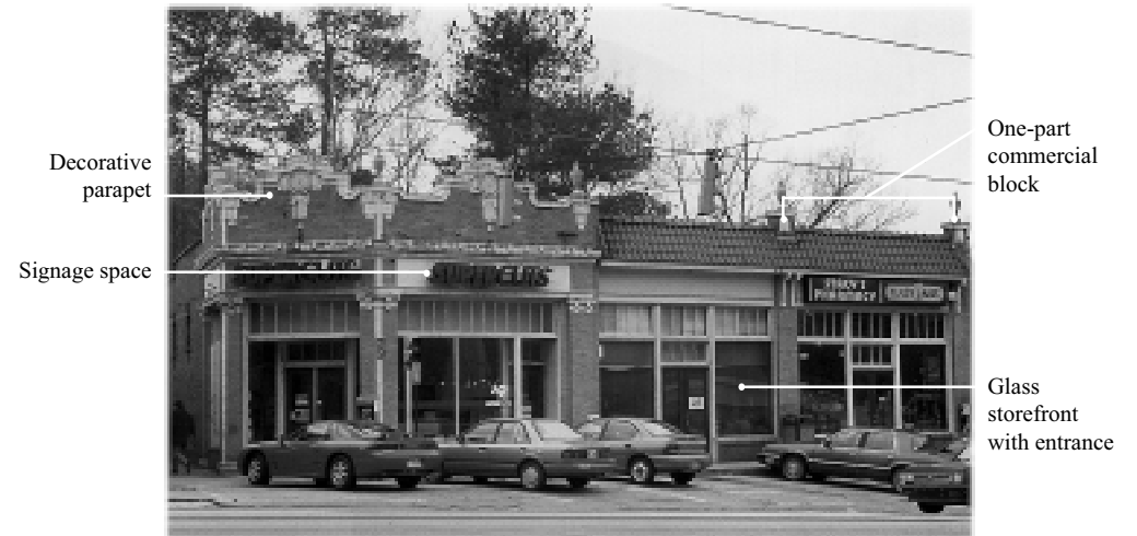
Historic commercial building in Emory Village with principal architectural features keyed.
