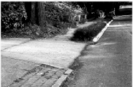
Example of historic granite curb in foreground and nonhistoric concrete curb in background. Note intrusive character of "white-colored concrete" when compared to subtle shades of granite.
