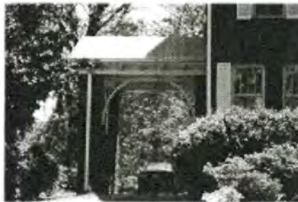
THE OPEN CHARACTER OF THIS PORTE COCHERE IS AN IMPORTANT FEATURE THAT SHOULD BE RETAINED
