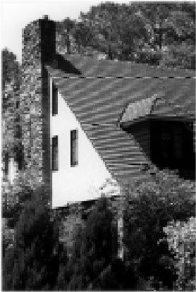
The random-stone masonry of this chimney is unusual in Druid Hills and should be properly maintained.
