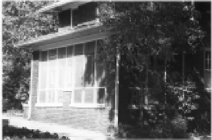
This side porch has been enclosed with screen, helping to maintain its original open character.
