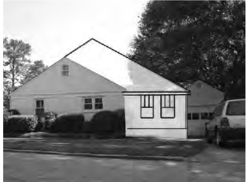
Poorly conceived addition that would mask the homes original proportions and character.
