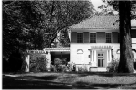
The open pergola design of this entrance porch, side porch, and porte cochere is a significant stylistic feature of this house and should be maintained.
