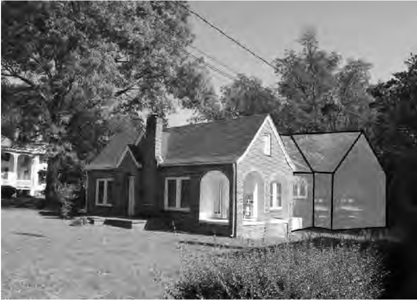
Well conceived addition that would substantially increase the size of the home while minimizing the appearance of the mass of the home. Breaking buildings into smaller architectural components avoids the perception of monumental façade.
