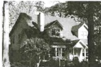
LARGE REAR ADDITION MADE TO THIS HOUSE OUT OF SCALE WITH ORIGINAL BUILDING
