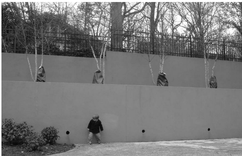
Large retaining wall on new construction that is out of scale with the built environment of Chelsea Heights.
