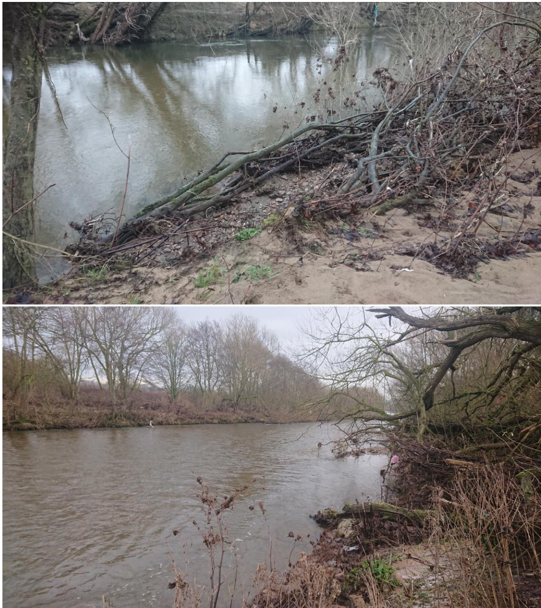
Fig 19. Mature willow specimens on the LB created some deeper water and cover around their roots. Small crack and goat willow specimens at the bank toe were providing the only other physical structure and cover within the channel but the extent of this was generally limited to within a metre or so from the bank. These images indicate how the complex of roots and branches trapped debris and caused the deposition of finer sediments (sand and gravel). Unfortunately, a combination of livestock trampling and Japanese knotweed had prevented further stabilisation of these sediments.
