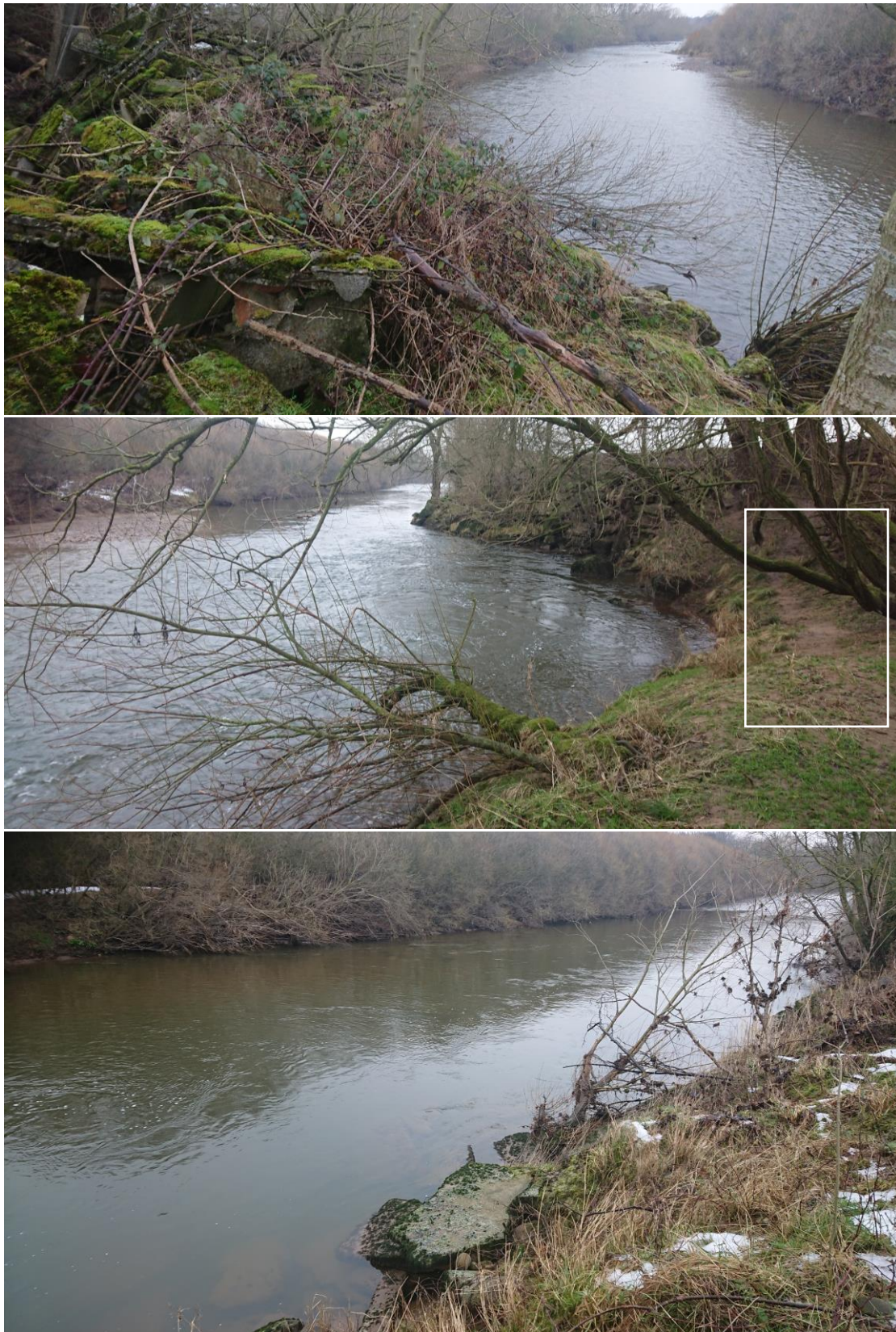
Fig 15. Various example towards the u/s limit where the RB top and face was predominantly concrete slabs dumped on the bank as 'protection'. Willow and bramble had managed to eke out a niche and establish some cover, but where sheep had easy access (eg middle image, white rectangle highlighting path), the cover was reduced and desire lines indicated weakening of the bank structural integrity.
