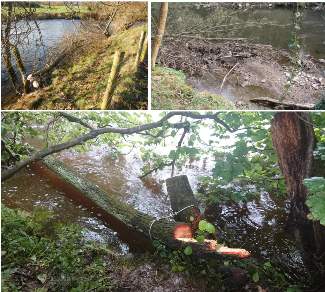
Fig 24 LH upper - hinged trees laid into the margins; RH upper- the impact of the crown of a tree kicker encouraging deposition in the lee and providing complex refuge habitat; Lower - felled alder and cabled back to living stump.
