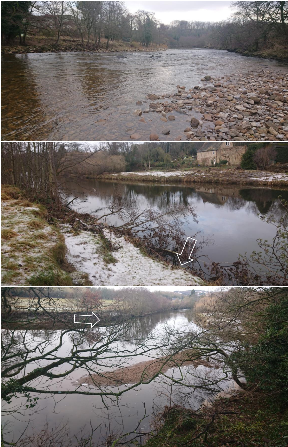
Fig 7. The straightened reach of Easby water looking d/s from Sand Beck (upper), a mid point of deeper glide (mid), and looking back u/s from the bend at Abbey Wood (lower). The unnatural course has left the river pinned to the LB at Abbey Wood where it is forced abruptly right over a bedrock seam. This has left the river with impounded characters u/s of the bend and much steeper d/s (see Fig 8). White arrows on mid and lower panel indicate the same point on the RB where erosion is evident on the inside of the bend.
