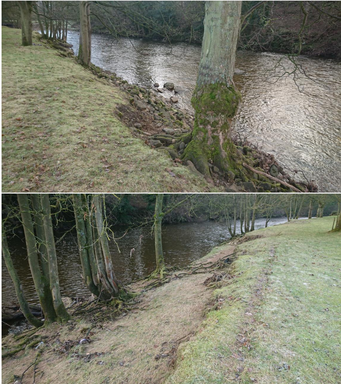
Fig 12. The channel was pinned against the right-hand side of the valley for much of the Red House Farm water. The LB had a sparse fringe of more mature trees along the channel that were all suffering from exposure of their root systems due to livestock grazing and trampling. Eventually, these will be lost and, again due to the livestock, there was no self-set regeneration to replace them.
