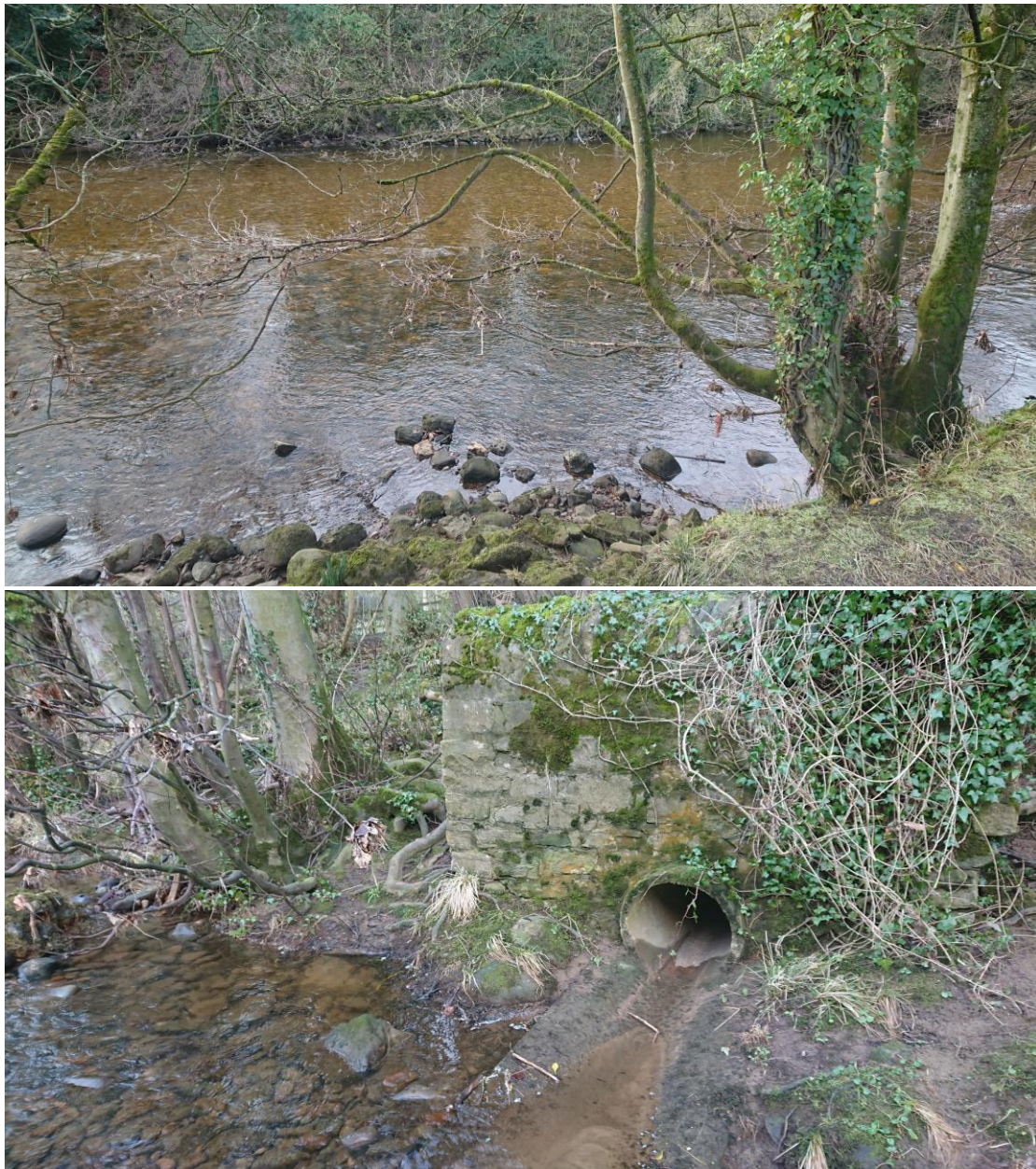
Fig 4. For at least ~500m (see Fig 1 from Mercury Br), the substrate toward the LB appeared markedly darker in colouration, despite changes in depth, flow path, shade / angle incident light etc. Various pipes were noted and the majority of Richmond infrastructure lies to the LB so this could reflect chronic inputs of nutrient from multiple sources.
