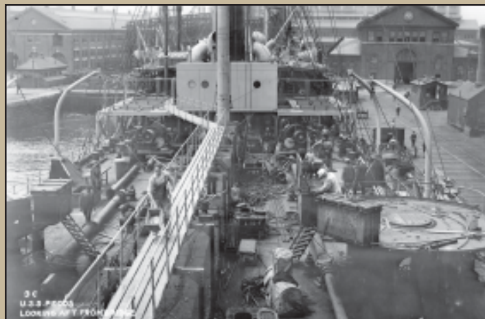
Following launching, much work remained to be done. On July 13, 1921, workers swarm over USS Pecos , berthed at Pier 7 West, even as USS Whitney (AD-4) begins to rise on the Shipways. Commissioned on Aug. 21, 1921, USS Pecos would be sunk by the Japanese on Mar. 1, 1942.
