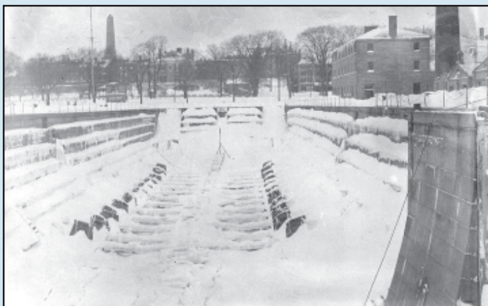
This view looks north along the center line of the Dry Dock. The Dry Dock Engine House (Building 22) is to the right at the head of the dock. Barely visible in the background is the Marine Barracks. The Bunker Hill Monument can be seen in the left background. BOSTS-14957
