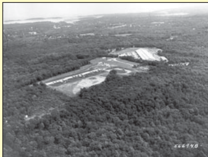
This aerial photograph taken on Aug. 12, 1959, shows the Cohasset Nike Site (BO-38). This facility, designated as Battery A, 3rd Missile Battalion, 52nd Artillery, was one of a series of anti-aircraft missile sites located around Boston. U.S. Army Signal Corps 566948
