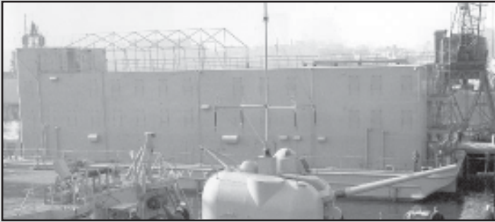
BERTHING BARGE — Berthing barges provided living space for sailors in shipyards while their vessels were undergoing repairs. This view shows Repair, Berthing, and Messing Barge YRBM-26 on Oct. 31, 1970, three weeks after delivery to the Navy from her builder, Marinette Marine of Marinette, Wisc. The Boston Naval Shipyard served as the facility for the delivery of naval vessels and craft built on the Great Lakes as well as along the northern New England coast. BOSTS-10868
