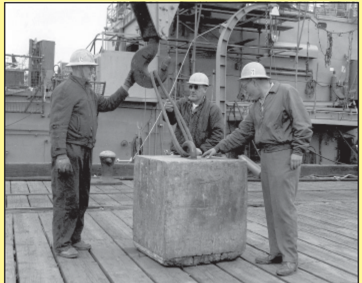
RIGGER — The term “rigger” encompassed more than one occupation. While the term is most often associated with the individuals who fabricate items out of rope, it also applied to men who were involved in the operation of cranes and other heavy lifting equipment. Here Foreman (Leadingman) Rigger Horace Grosshandler (center) supervises Riggers Jacob K. Mulley (left) and John Carr in lifting a 5-ton test weight onto the destroyer USS Fiske (DD-842) in Dec. 1967. BOSTS-7740
