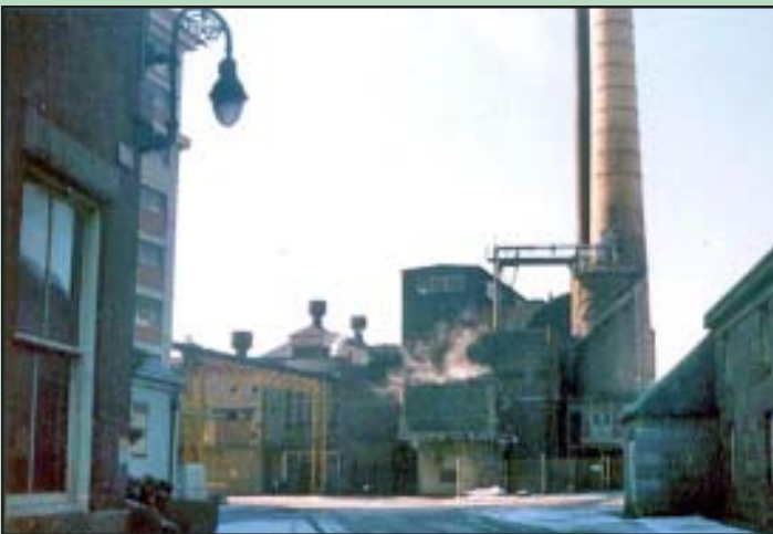
Building 108, Cooling Tower 264, Ash Silo 268
