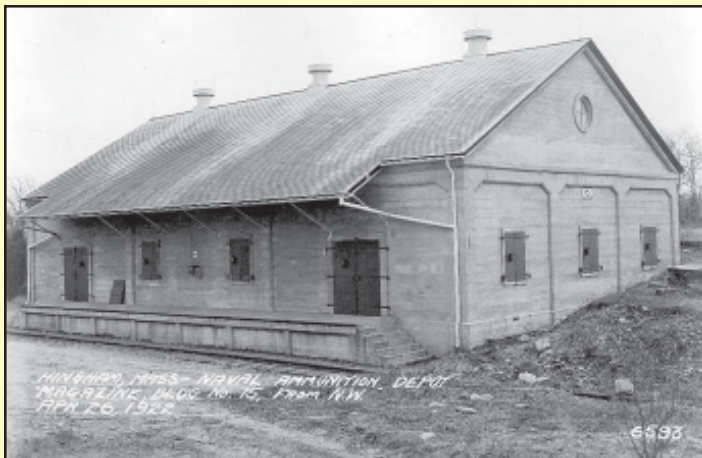
The individual storage buildings at the NAD Hingham were fairly small in size and constructed of concrete to reduce danger of explosion and fire. This Apr. 26, 1922, photograph of Building 15, one of the site's many Magazines, is part of an early 1920s project to document the facilities of the First Naval District. BOSTS-8079
