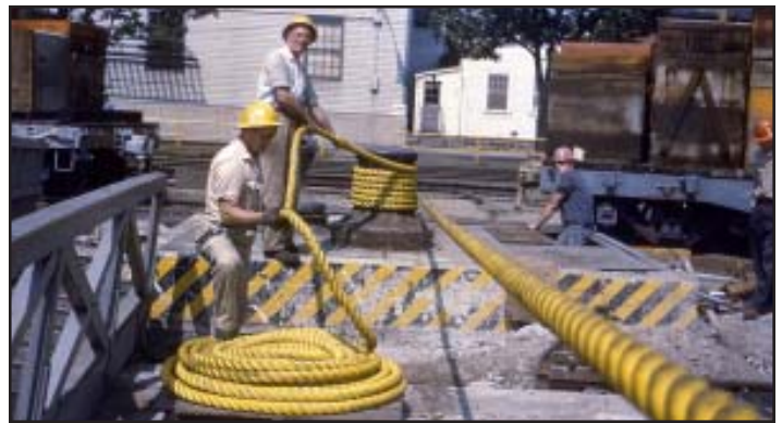
CAPSTAN — The Navy Yard utilized electric capstans to assist maneuvering ships in its dry docks. Here workers play out nylon rope being wound around the capstan at the head of Dry Dock 2 in the early or mid-1960s.
