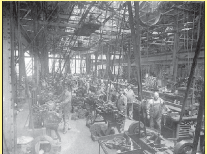
MACHINIST — Machinists fabricated numerous components for ships using a variety of machines such as lathes, drills, and presses. This June 13, 1913, view of the Machine Shop (Building 42) shows the numerous belts which ran the machines from overhead shafts prior to the introduction of individual electric motors for each machine. BOSTS-9433
