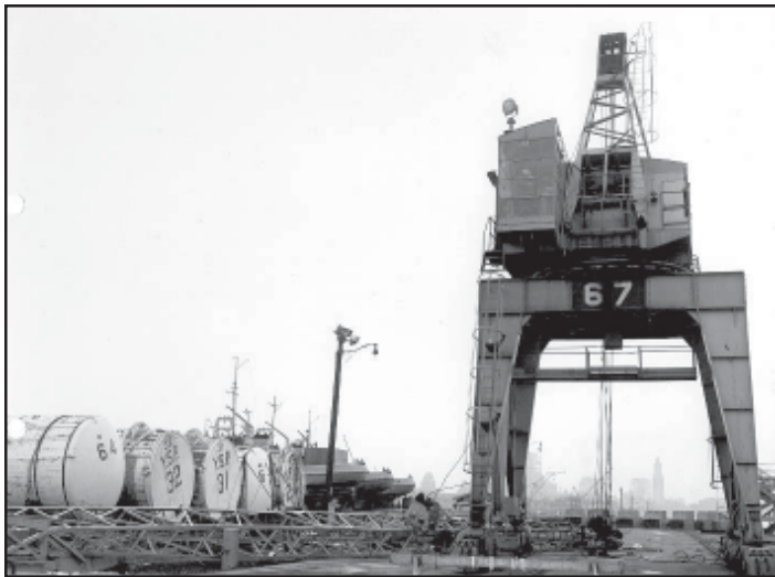
Shipyards operations were always hazardous, and yard photographers were called out to document major accidents. (Left) On the afternoon of Feb. 17, 1965, the boom of Portal Crane 67 collapsed during a load test, which had proceeded despite the crane operator's report that the crane was not operating properly. Fortunately, no one was injured in the accident, which took place on the North Jetty at the South Boston Annex. Note the salvage pontoons at left. (Right) Three and a half months later, on June 1, 1965, the boom of Portal Crane 21 collapsed. In that accident, which occurred on Pier 6, the driver of a passing truck was killed. Note floating crane YD-77 (YD-77) at right being used to lift the broken boom. BOSTS-13347
