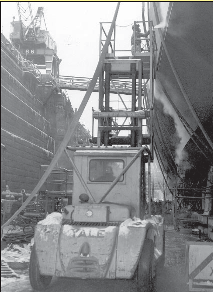
PAINTER — Shipyard painters often worked under difficult conditions. On Dec. 16, 1970, a painter sprays the hull of USS Little Rock (CLG-4) in Dry Dock 3 from scaffolding supported by a forklift. BOSTS-11814
