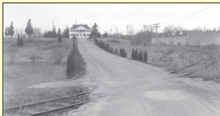
As with other military facilities in the area, the NAD benefited from WPA projects in the 1930s. This Dec. 2, 1937, view shows the widened roadway leading to the Administration Building (Building 114). Note the railroad tracks which provided for internal movement of munitions. One of the many concrete Storehouses (Building 100) is seen at right. BOSTS-8167
