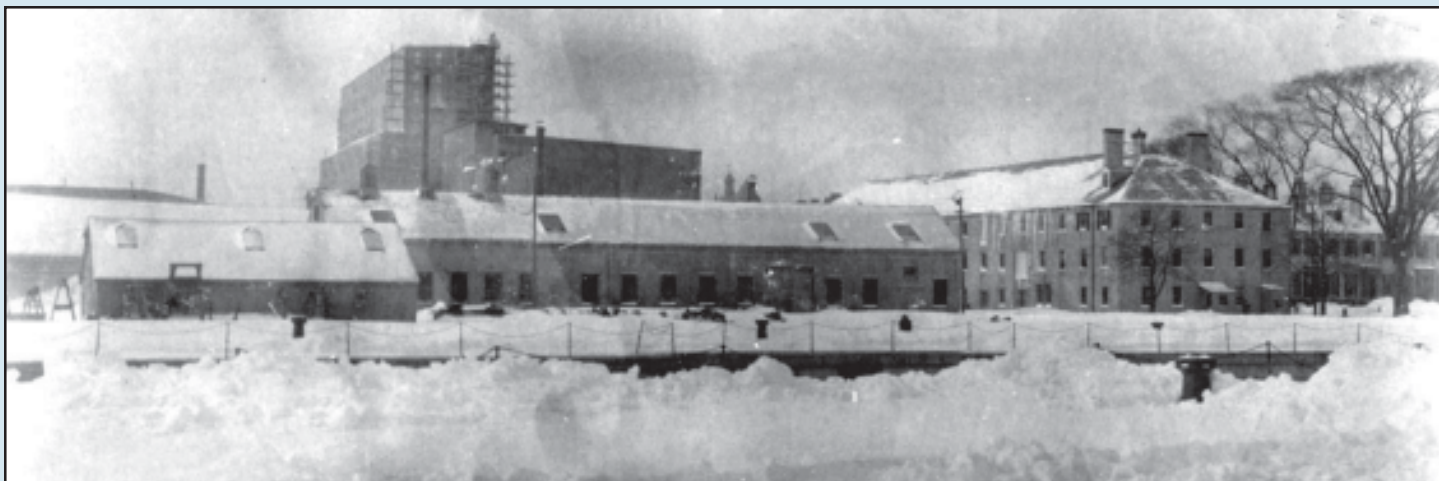
This view looks west across the Dry Dock. From left to right are the Boat House (Building 94); the Foundry (Building 16); the Store House (Building 5), then housing a variety of activities including the pay office, dispensary, labor board, museum, and paint shop; and Quarters B-F. Rising above the roof of the Foundry are the Hoosac Docks Grain Elevator and Hoosac Stores No. 1 & 2. BOSTS-14957
