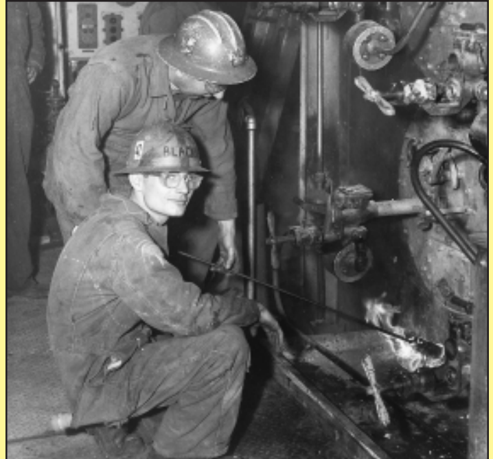
BOILERMAKER — Boilermakers dealt with the main propulsion systems of steamships. Here, Boilermaker Philip A. Ruggiero holds the torch to “light off” the boilers on USS Decatur (DDG-31) in Jan. 1967. In the foreground is Helper Boilermaker Richard E. Black.
