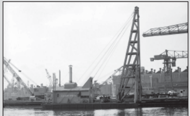
FLOATING PILE DRIVER (YPD) — Floating pile drivers were used in the maintenance of the Navy Yard's waterfront facilities. Acquired in 1942, YPD-24 sits at Pier 8 on Lincoln's Birthday, 1960. BOSTS-14883
