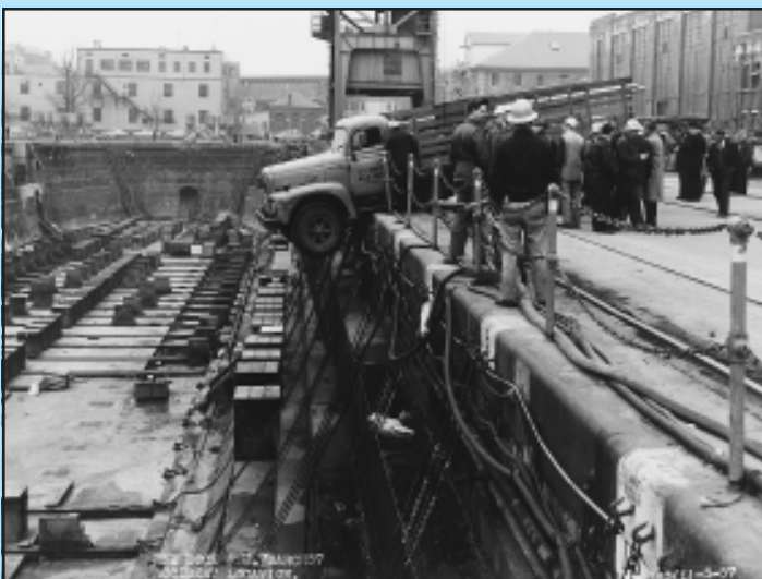
Yard photographers were called out to document accidents which happened in the yard. Image 863-57 was taken on Mar. 7, 1957, after Navy stakebody truck 97-07924 went through the railing surrounding Dry Dock 2. BOSTS-15698
