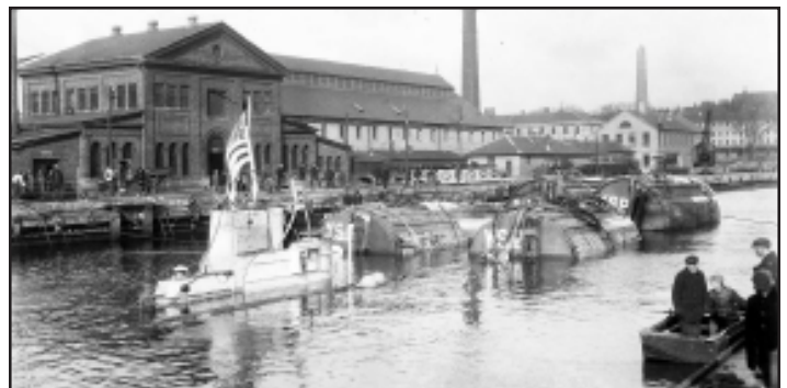
PONTOON — The Navy used pontoons for salvage work. Four of the six salvage pontoons used to recover the sunken submarine USS S-4 (SS-109) are seen forward of the conning tower as the boat is maneuvered into Dry Dock 2 on Mar. 19, 1928. BOSTS-14138
