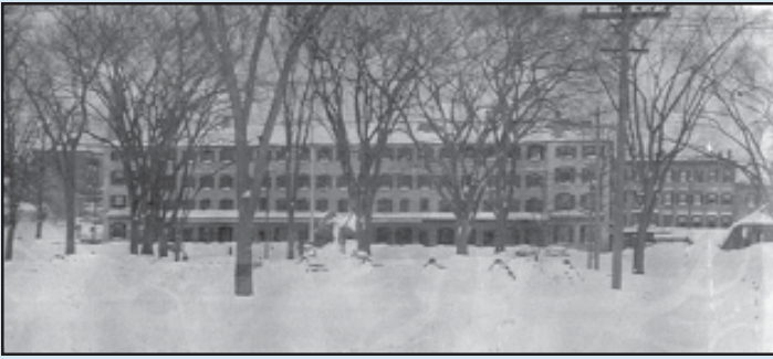
This view shows the Marine Barracks (Quarters H-I-K) looking across a depleted Shot Park. Note the USS Niagara figurehead in the center and the Marine Corps Officer of the Day Office (Building 30) at right.
