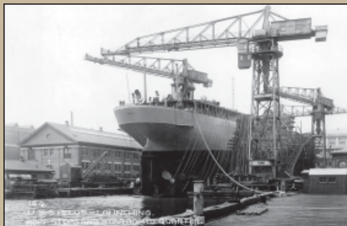
By April 22, 1921, all was in readiness for launching. Vessels were built so that the stern was the first part to enter the water.
