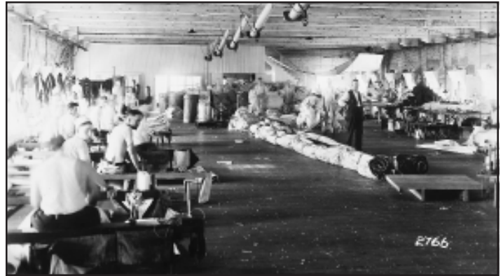
SAIL LOFT, YARD — The Navy Yard’s Sail Loft in Building 33 is seen in this photograph taken around August 1917. Note the suspended yards which allowed sails to be hung. BOSTS-9333
