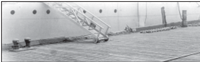
BITT, BOLLARD, BROW — This photograph of Pier 6 East from July 1923 shows, from left to right, a bitt , the brow providing access to the ship, and a bollard . BOSTS-15623
