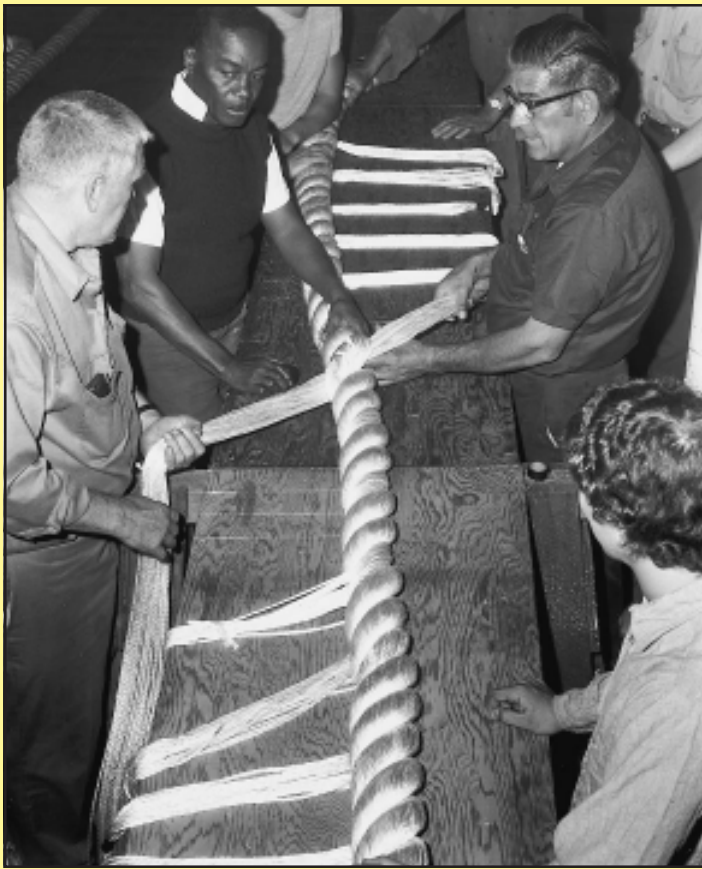
RIGGER — One of the oldest shipyard trades was that of rigger, responsible for the miles of rope used on sailing ships. Although used in far smaller quantities in the modern age, rope remains a critical item for naval vessels. Here riggers splice together a piece of nylon rope in Sept. 1970. BOSTS-9307
