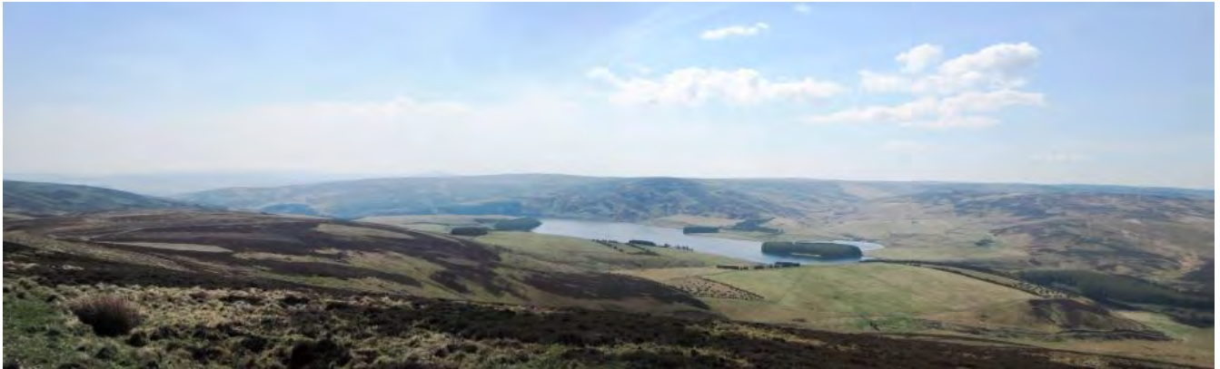
The Whiteadder reservoir surrounded by pastureland enclosed within the rising peaks of Priestlaw and Penshiel Hills viewed from Spartleton
