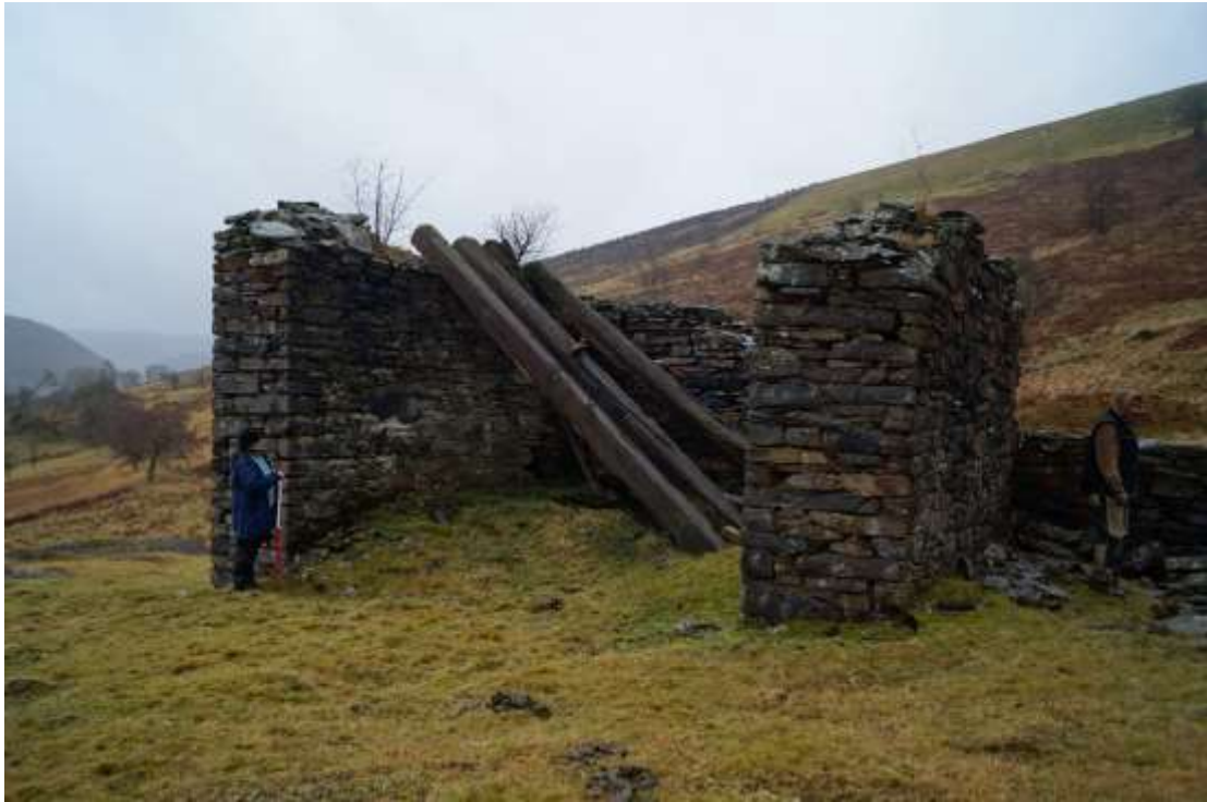
The remains of the crusher-house at the Cwm Elan Mine complex.
