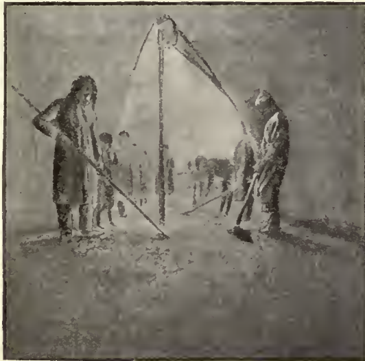
FIG. 4.—Breaking the earth under tent.
