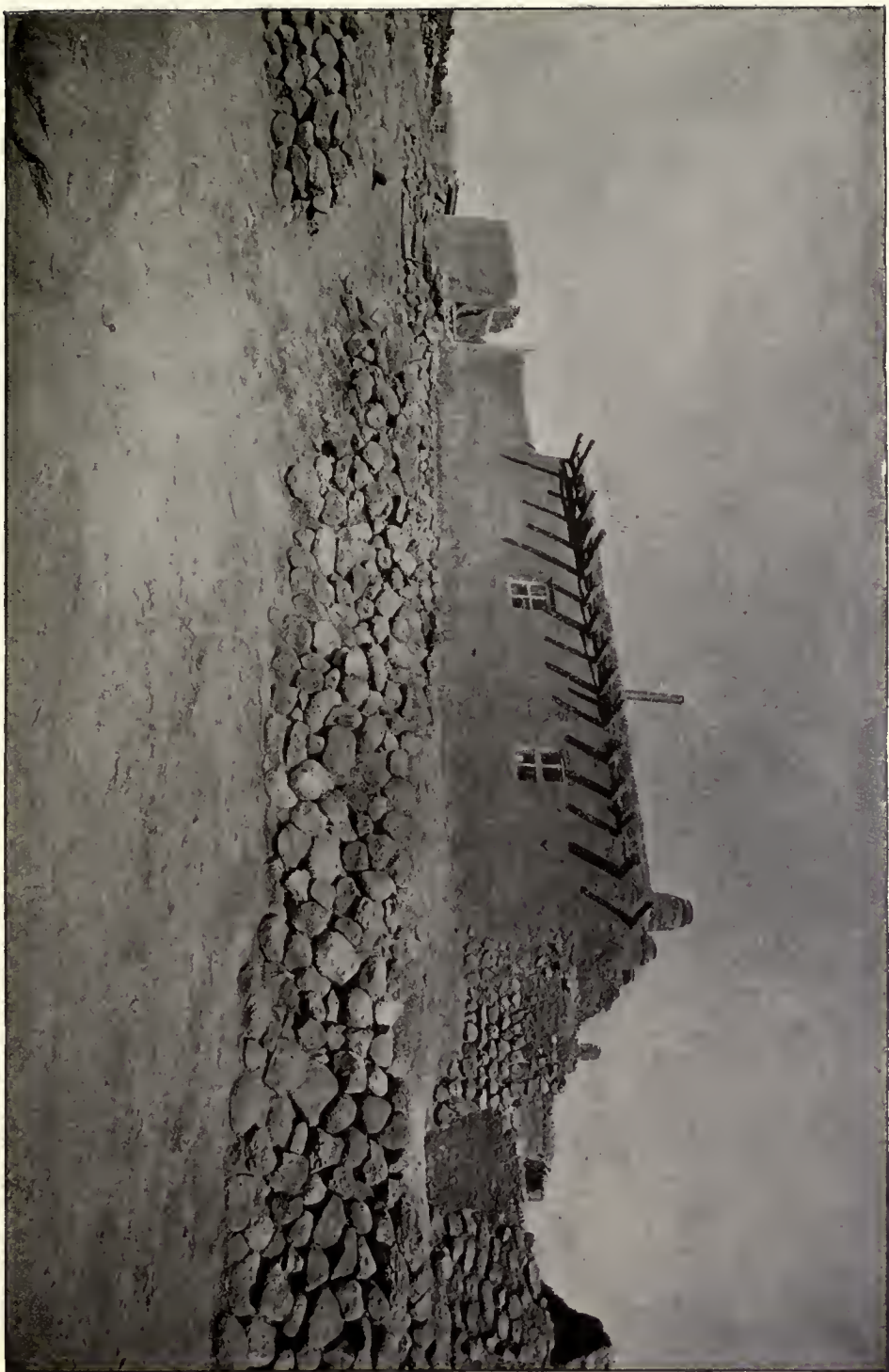
STONE HOUSE, SHOWING PLASTER ON EXTERIOR.
