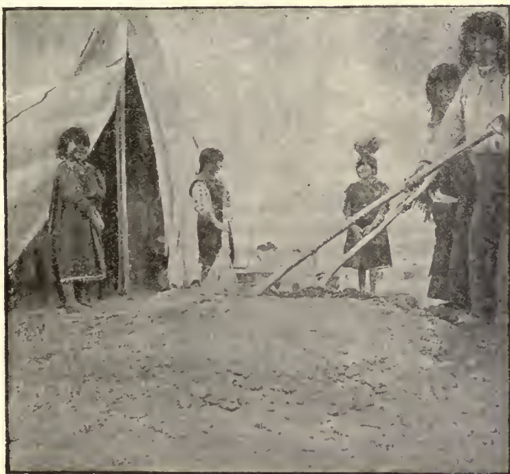
FIG. 12.—Mixing clay for plaster.
