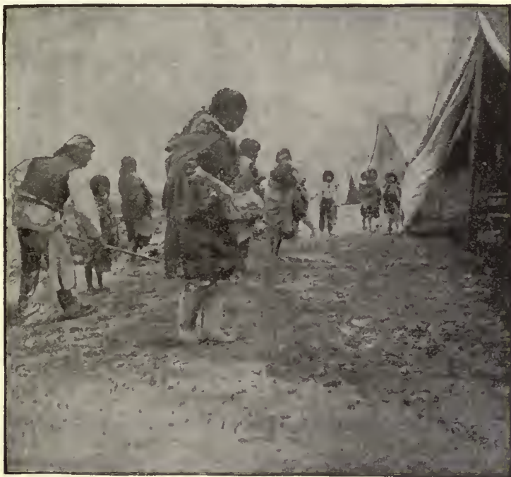
FIG. 10.—The process of leveling.
