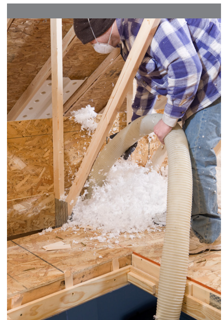
Insulation being blown into attic to increase heat retention in a home.
