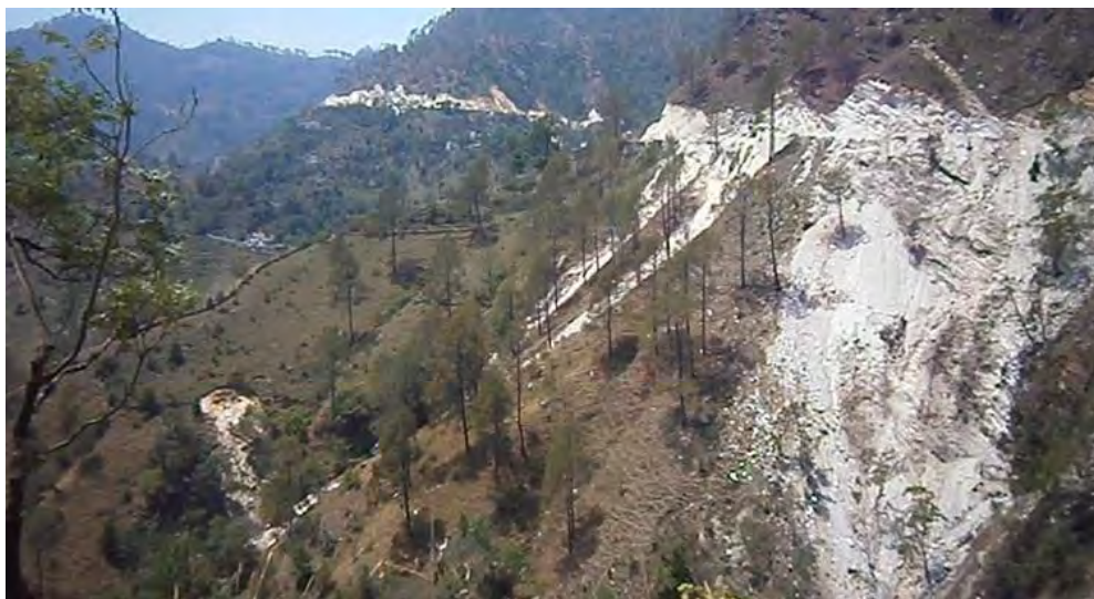
Enroute Askot, lots of debris flowing down the slope
