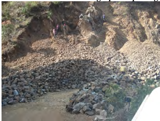
Road Cutting: A hill opened up for extracting material for road construction
