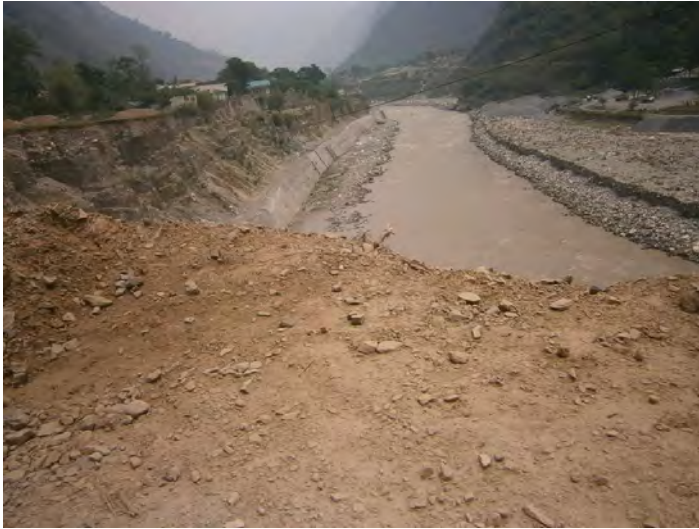
Washed off right terrace along Kali, road realigned later (see google map shown)
