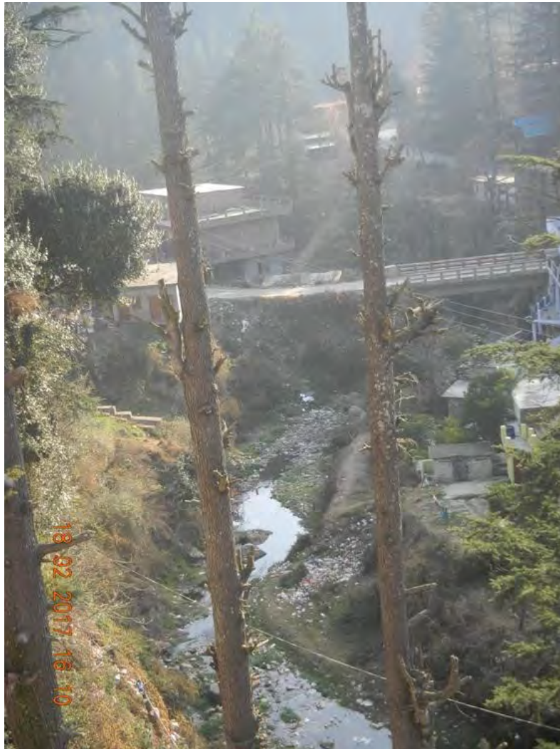
Lohawati flowing through Lohaghat; Salna lift scheme (below)
