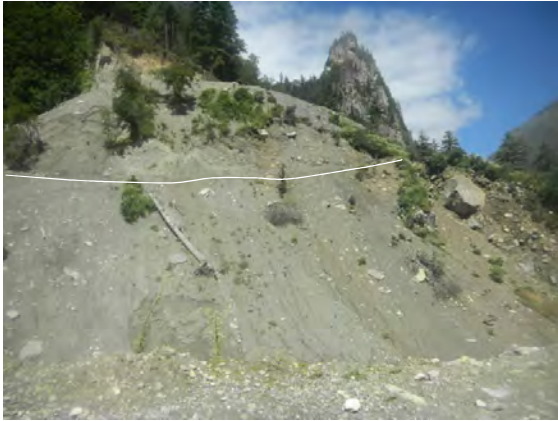
Huge debris flow due to hill side cutting for road en-route Darma (white line indicating road level)
