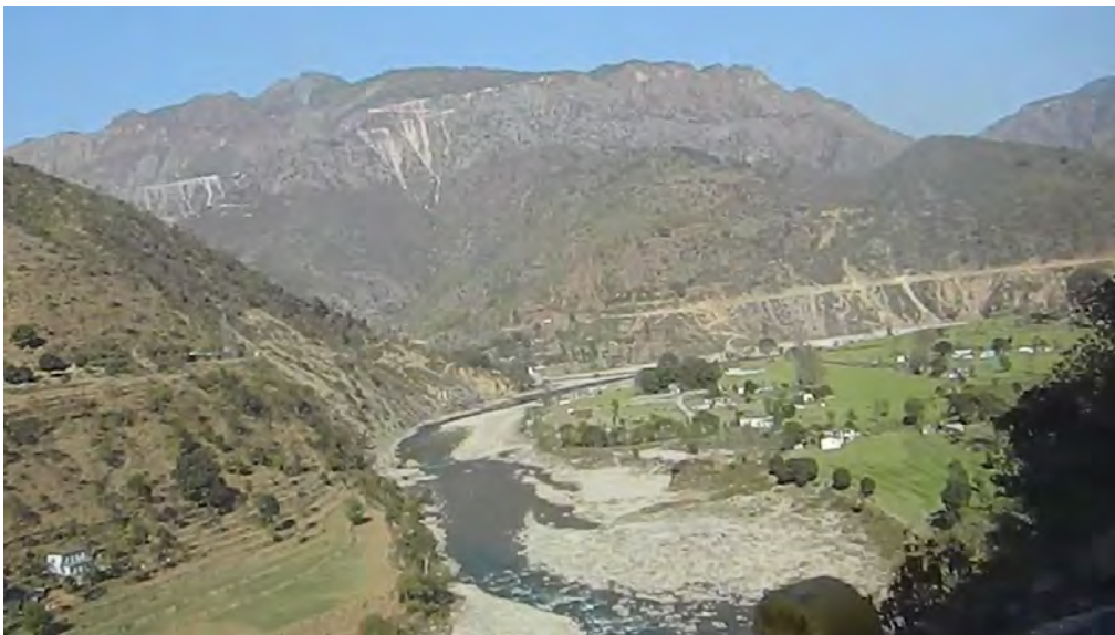
A view of Saryu Valley, road construction activity is easily noticed here
