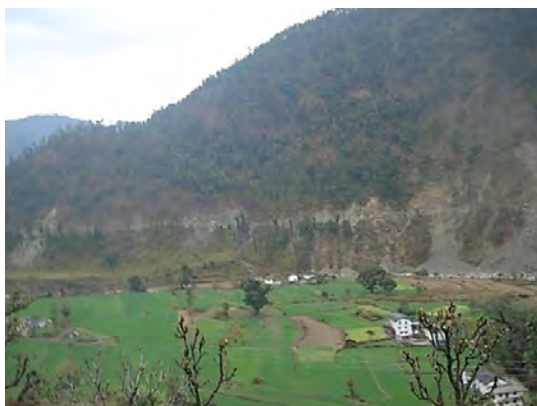
View of Road link to Amori across the River as seen from Macchiyar Road – One can see the disturbance and slides
