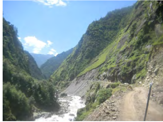
Road alignment along River Dhauli, sliding areas have increased
