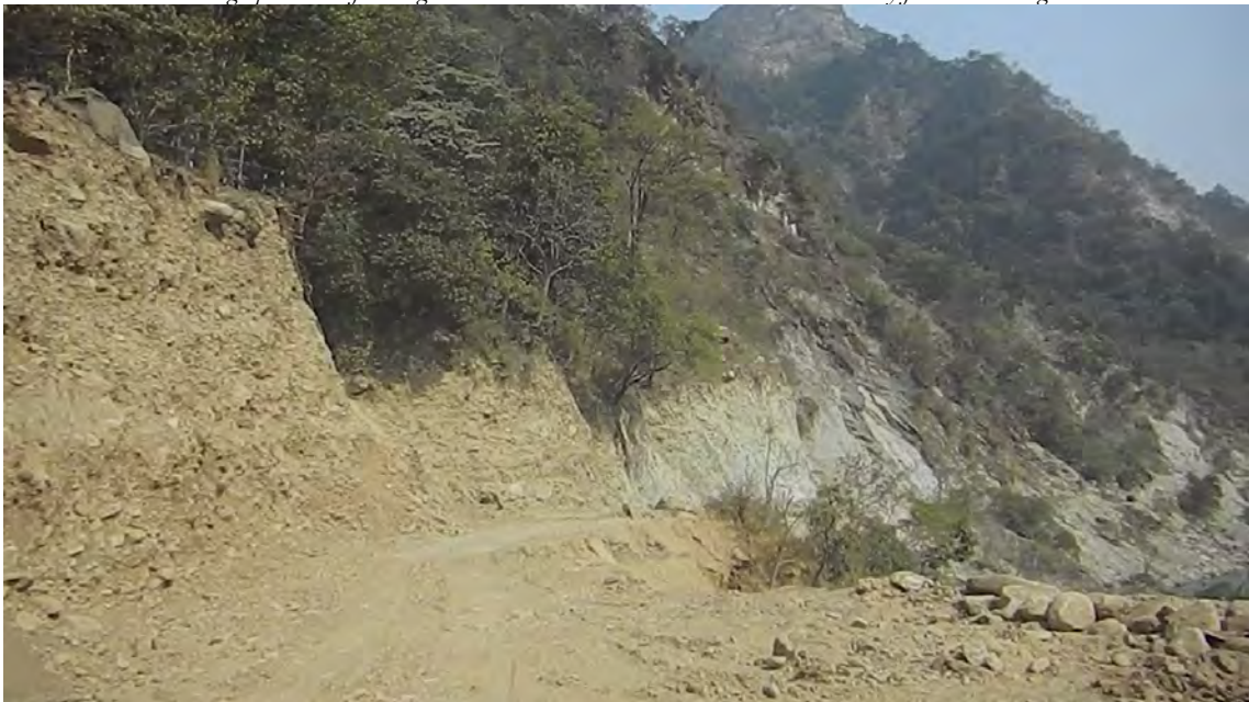
Road cutting for Thuligad-Rupaligad alignment underway, the hills constitute boulders, stones, soil and other aggregates having high potential of sliding
