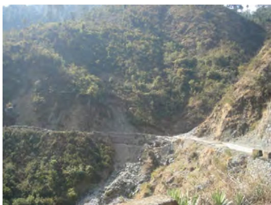
A rock slump – 600m from Saal en-route Taand
