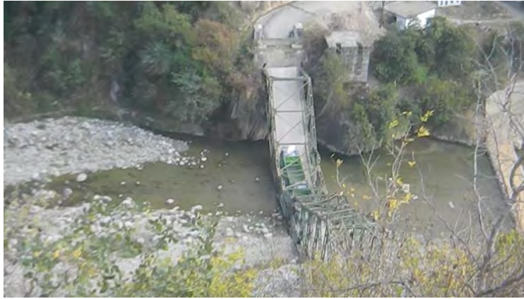
A bridge collapse on river Kulur, the bridge collapsed probably under the weight of truck which is seen stuck on the bridge
