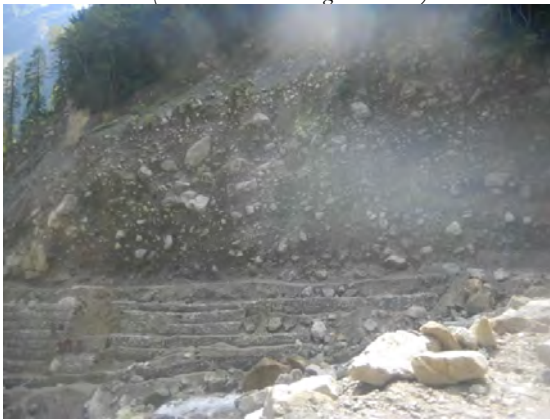
Slope protection work, Beyond Urthing
