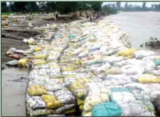
Right Bank of Mahakali River at Dhakanaghat
