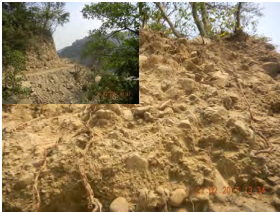
Road cutting for Thuligad-Rupaligad alignment underway, the hills constitute boulders, stones, soil and other aggregates having high potential of sliding
