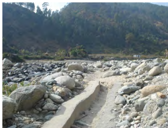
Typical inlet point for a gravity canal along the river bed (Champawat District)
