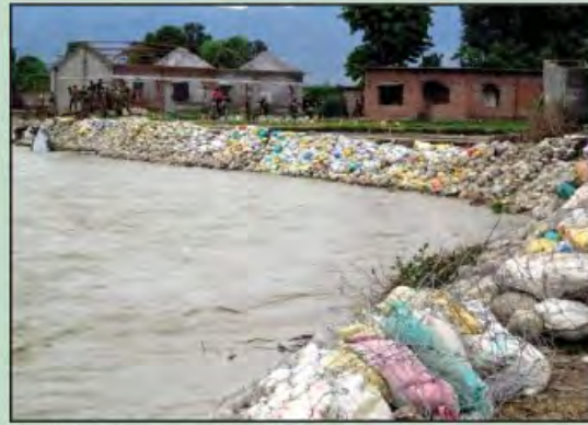
Right Bank of Mahakali River at Dhakanaghat
