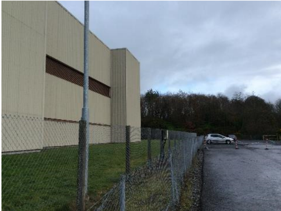
Figure 15.15 B 21 (SE elevation), looking ENE towards landscaped berm & Old Rectory (RPS 614).
