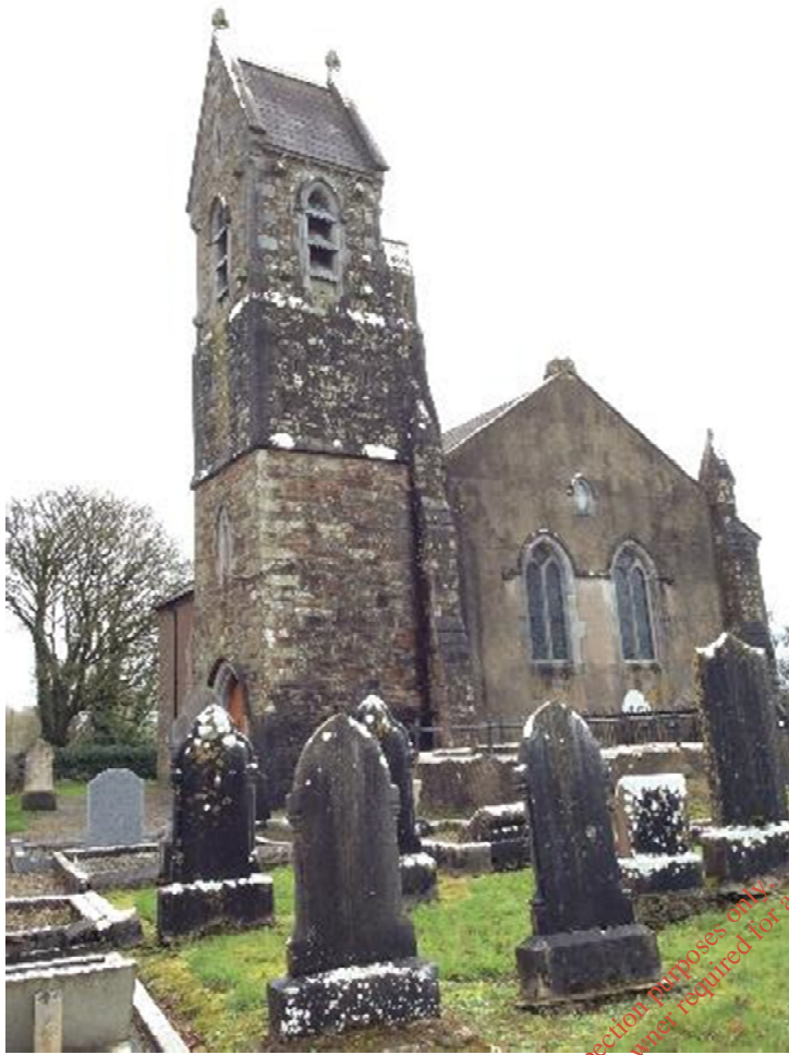
Figure 15.10 Church and graveyard CO096-069001 and 002, looking SE.
