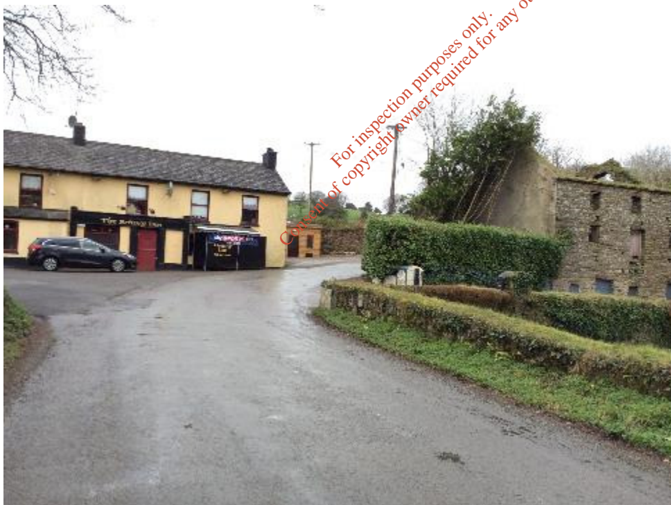
Figure 15.12 Rear of Corn mill CO096-055 on right of photo.
