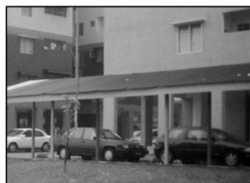
Car parking area
