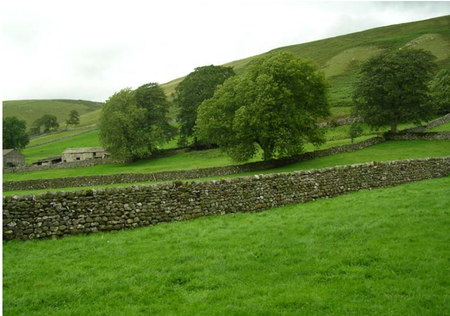
Plate 8: Restored wall at Sawyers Garth Farm
