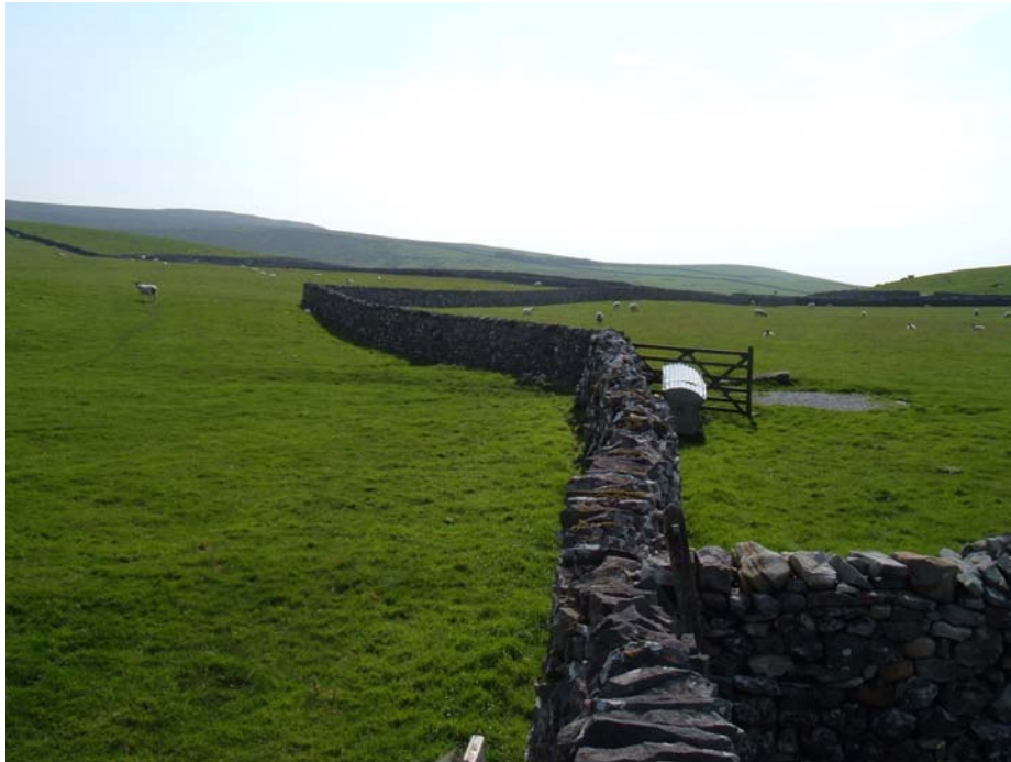
Plate 13: Long-distance views of restored walling in context of the Dales landscape
