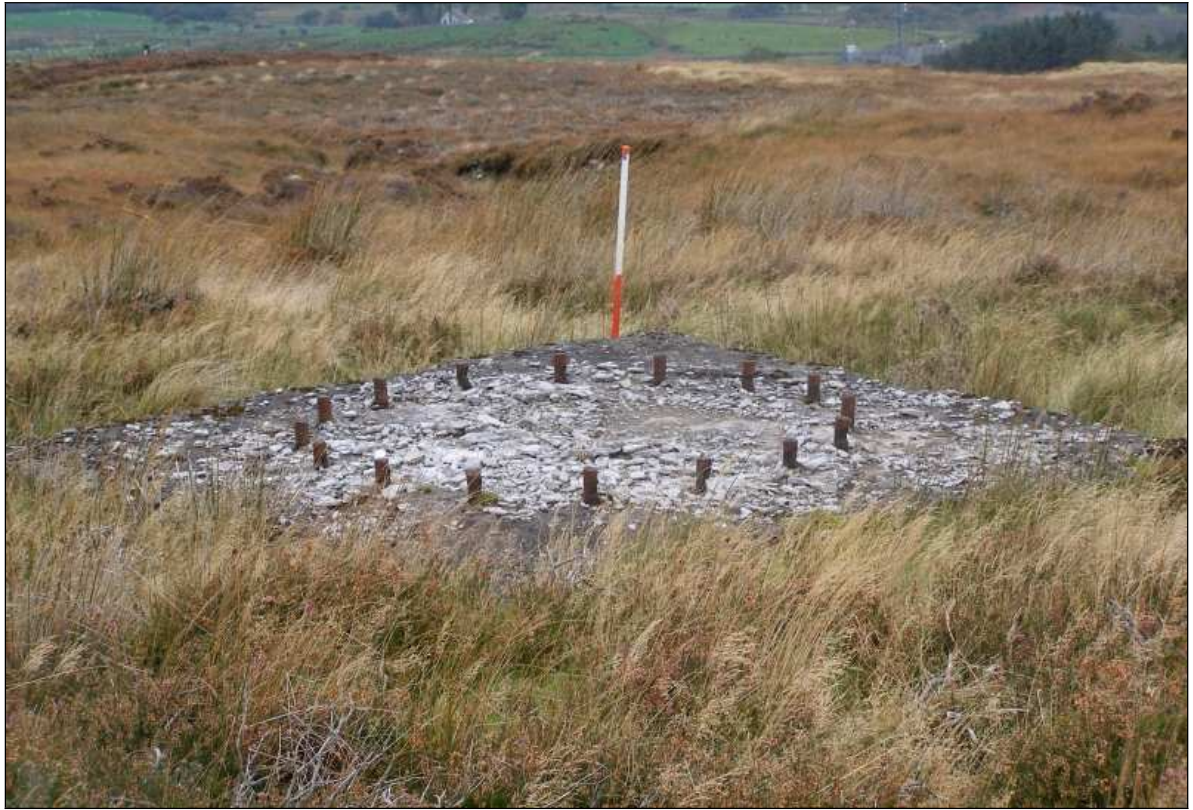
Plate 21: Current surviving example of a radio antennae mast base (NMR 270469)
