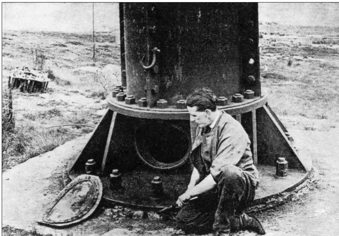
Plate 20: Early view of a radio antennae mast base at the Marconi Transatlantic Transmitting Station near Waunfawr (NMR 405838) (Waunfawr Radio Station Archive)
