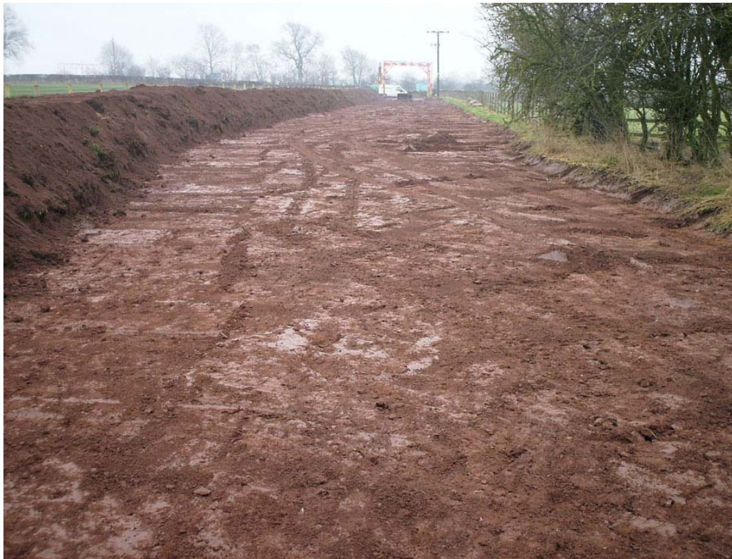
Plate 2: Easement north of Newton Road, Field 4, looking south
