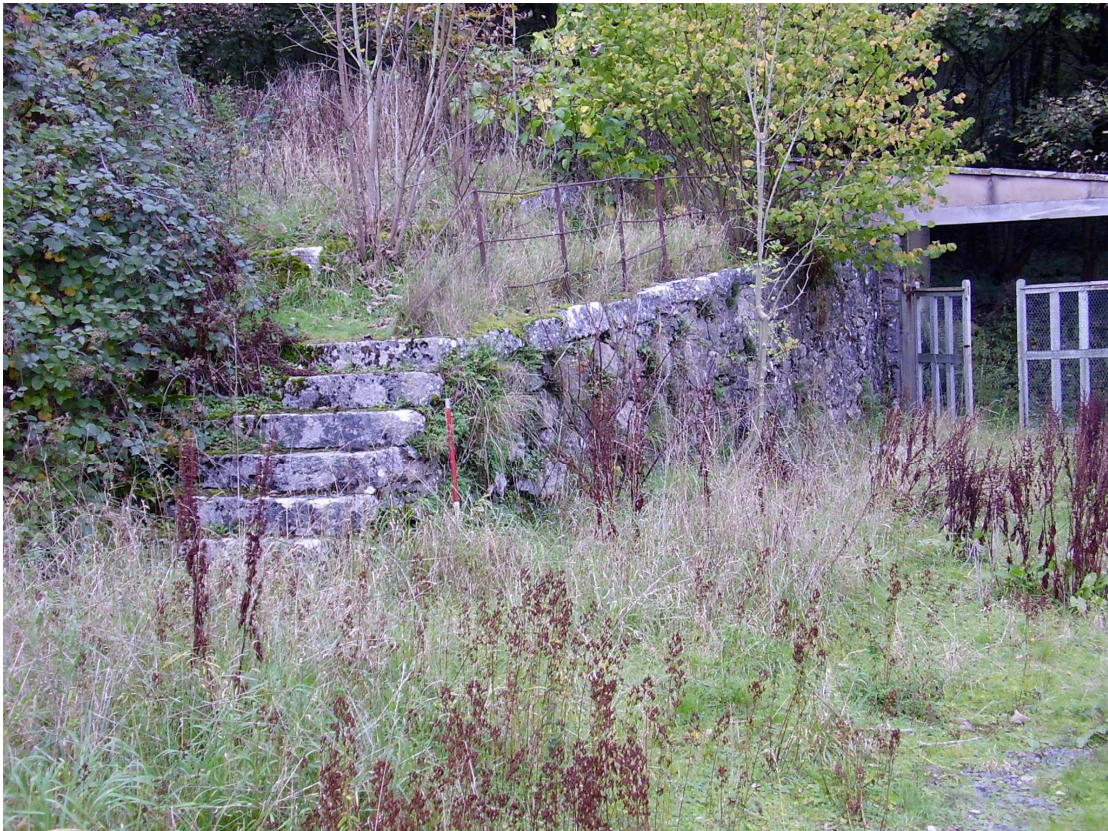
Plate 4: Terrace and steps within the walled garden (Site 21)
