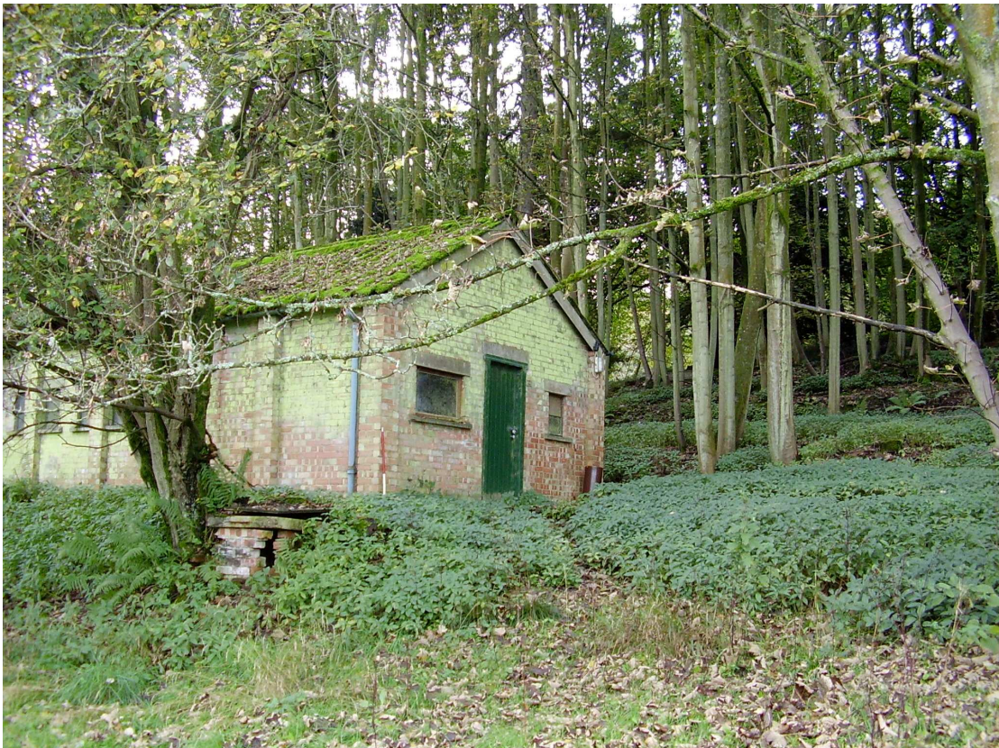
Plate 8: Another of the Site 30 World War Two structures
