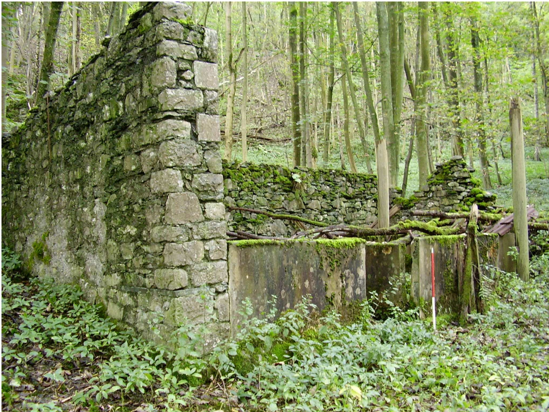
Plate 6: Derelict building (Site 24) to the north of Merlewood
