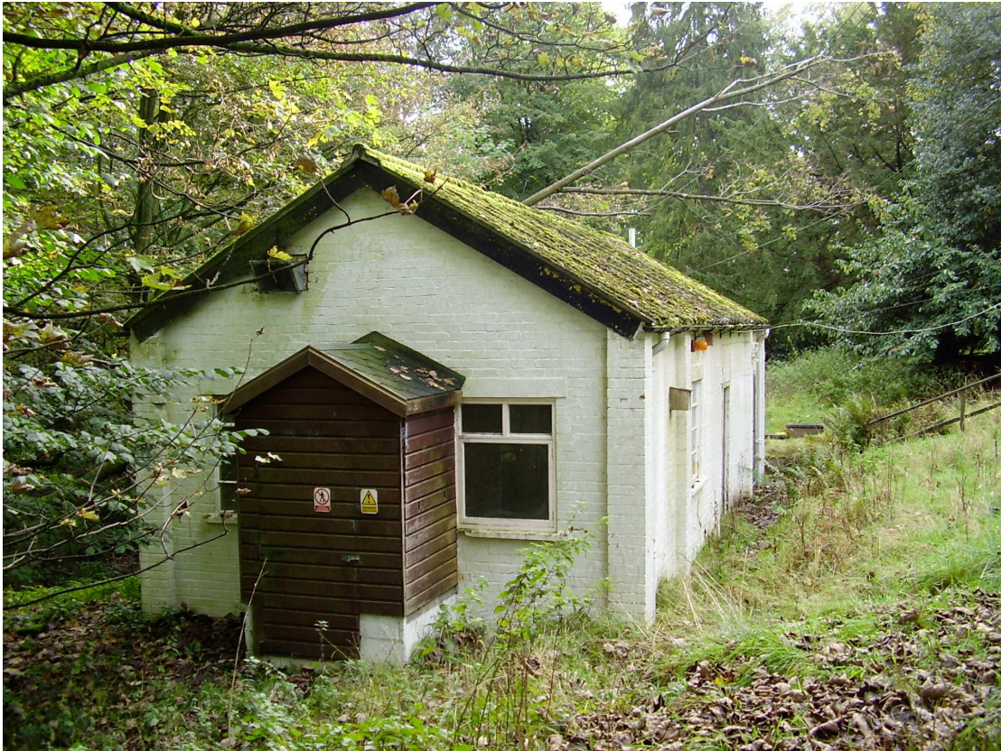
Plate 7: Brick-built structure (Site 30) likely to relate to the Second World War use of Merlewood
