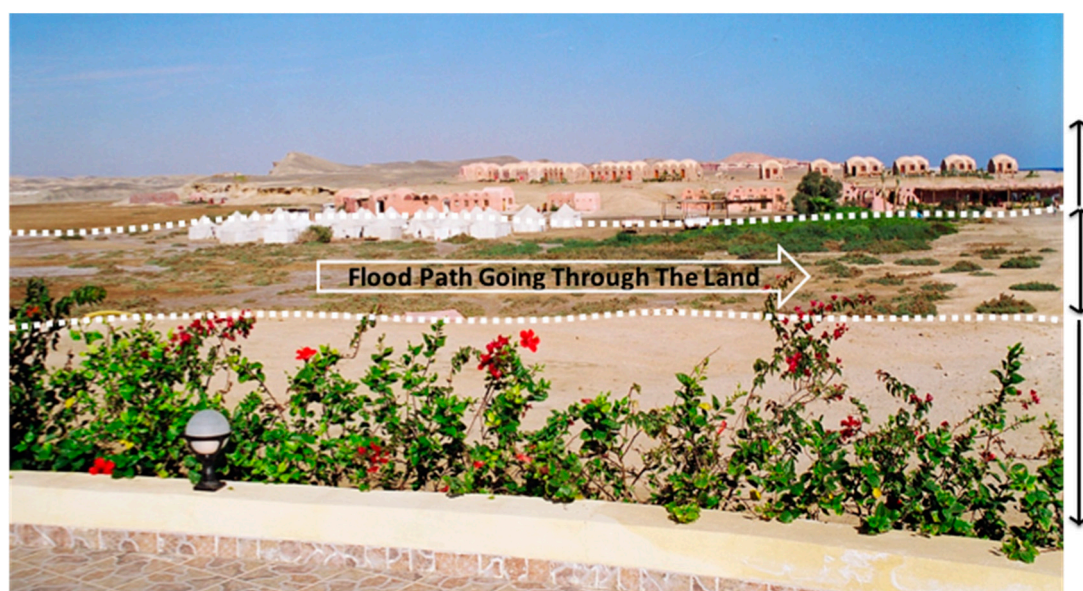
Figure 8. Example of resort that avoided construction on salt marshes (placing buildings on adjacent high land) even when the allocated parcel was primarily marsh. View of Shagra Eco-lodge, looking north across Wadi Shagra. (Photo by Gohar, January 2004).
