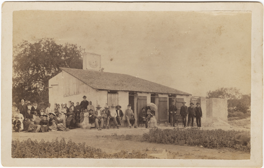
FIGURE 15. Topo Chico bathhouse, c. 1890. With permission of DeGolyer Library, Southern Methodist University, Dallas, Texas. AG1987; 0643.
