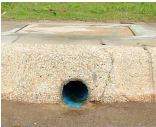
Stormwater draining to ocean
