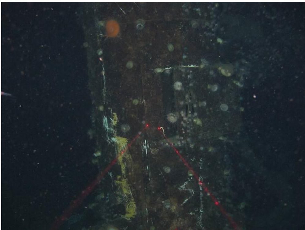
Figure 8-12. Light cnidarian encrustation with no L. pertusa on base of the abandoned test pile near the Zinc installation (within 5 m of the sea floor).
