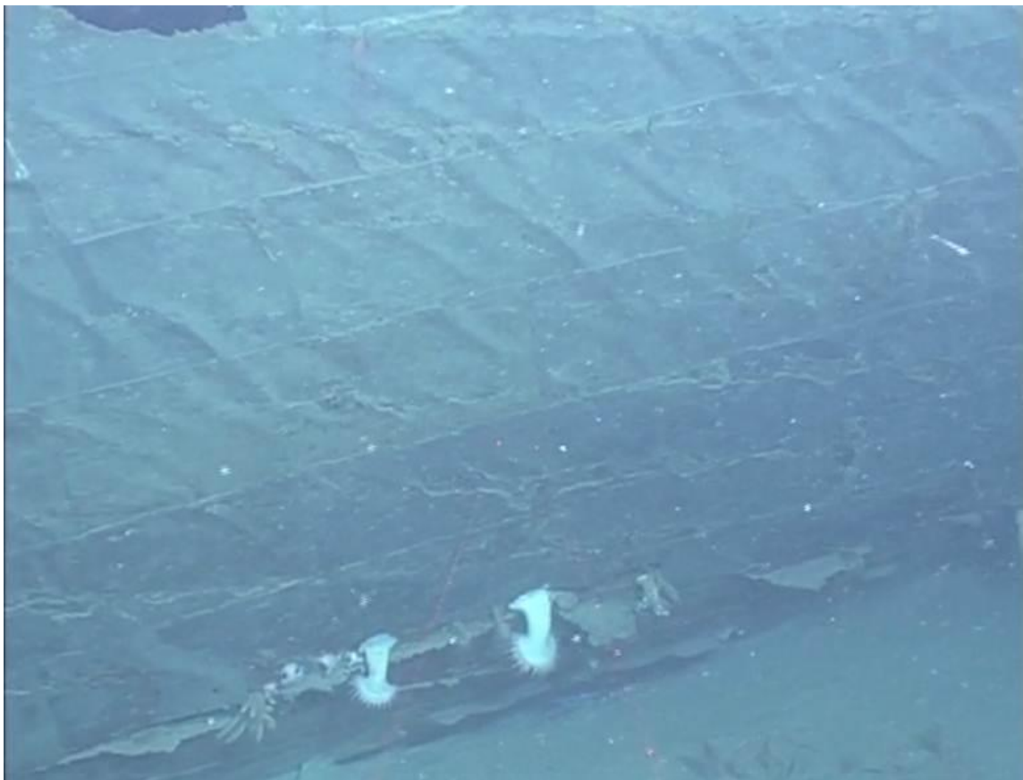
Figure 10-14. Diagonal foiling observed in sheathing (Starboard side).
