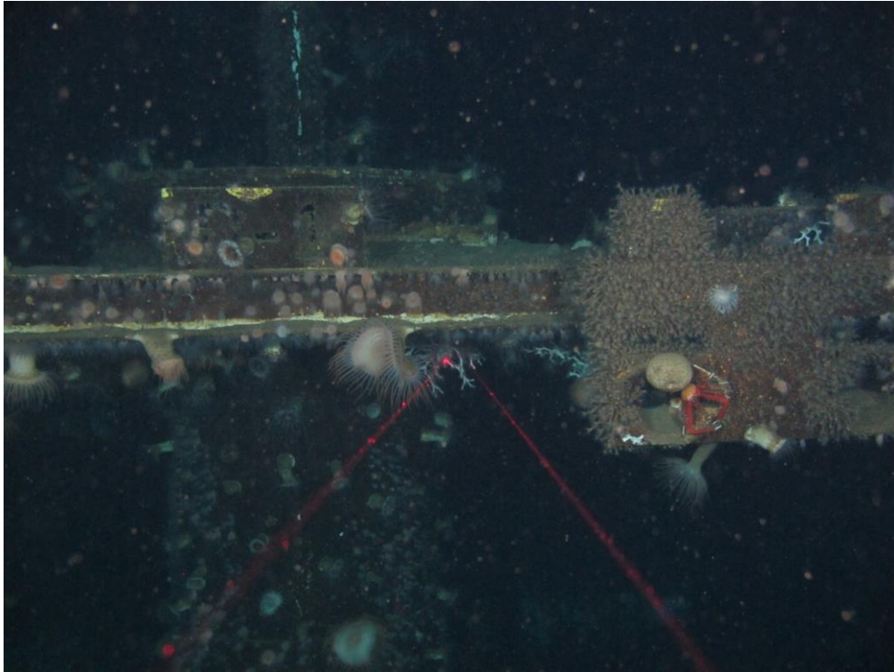
Figure 8-11. Fauna incrustated flow-tube connection about 7 m above the sea floor at the Zinc installation.
