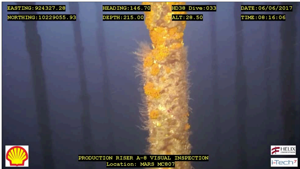
Figure 3. Part of the riser field below Shell's Mars (MC807A) platform.
