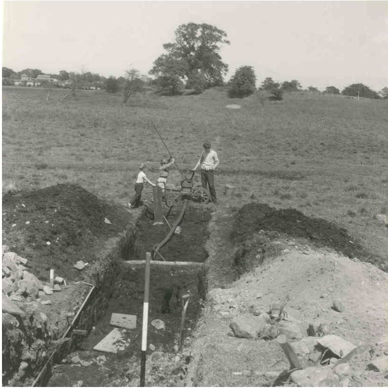
Fig. 3 Trench D (?) showing the need for a pump to remove ground water – looking east? (Gelling Collection - Shropshire Council Archive)
