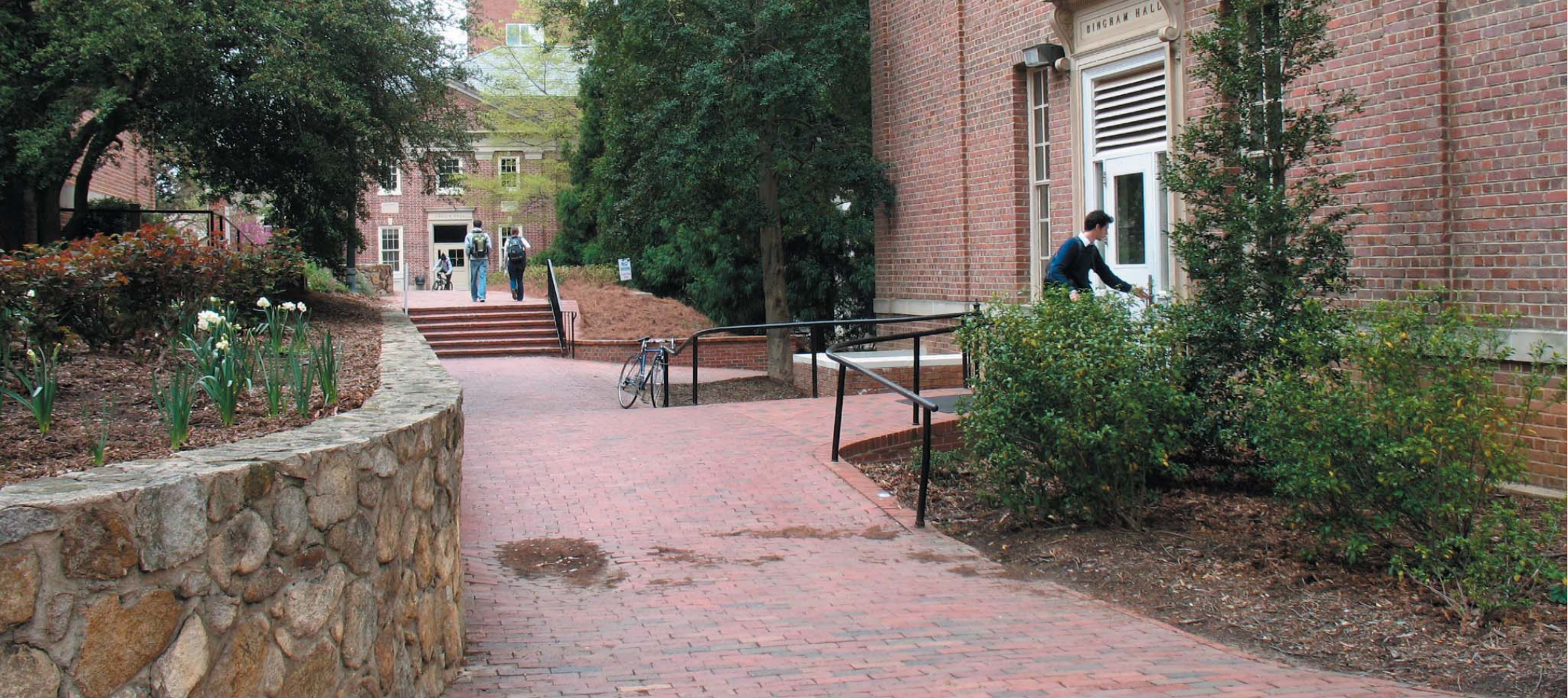
Polk Place existing condition at building envelope, 2008
