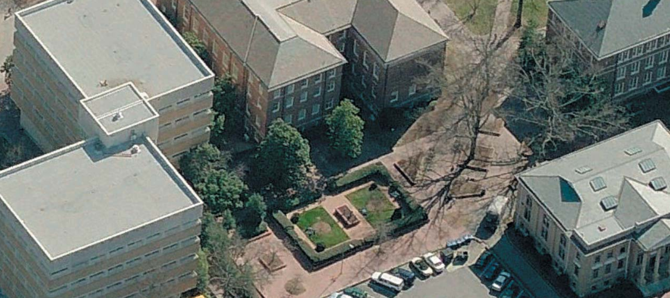
Bynum Hall quad, existing condition, 2008
