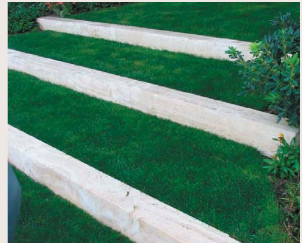
Example of limestone risers with turf treads
