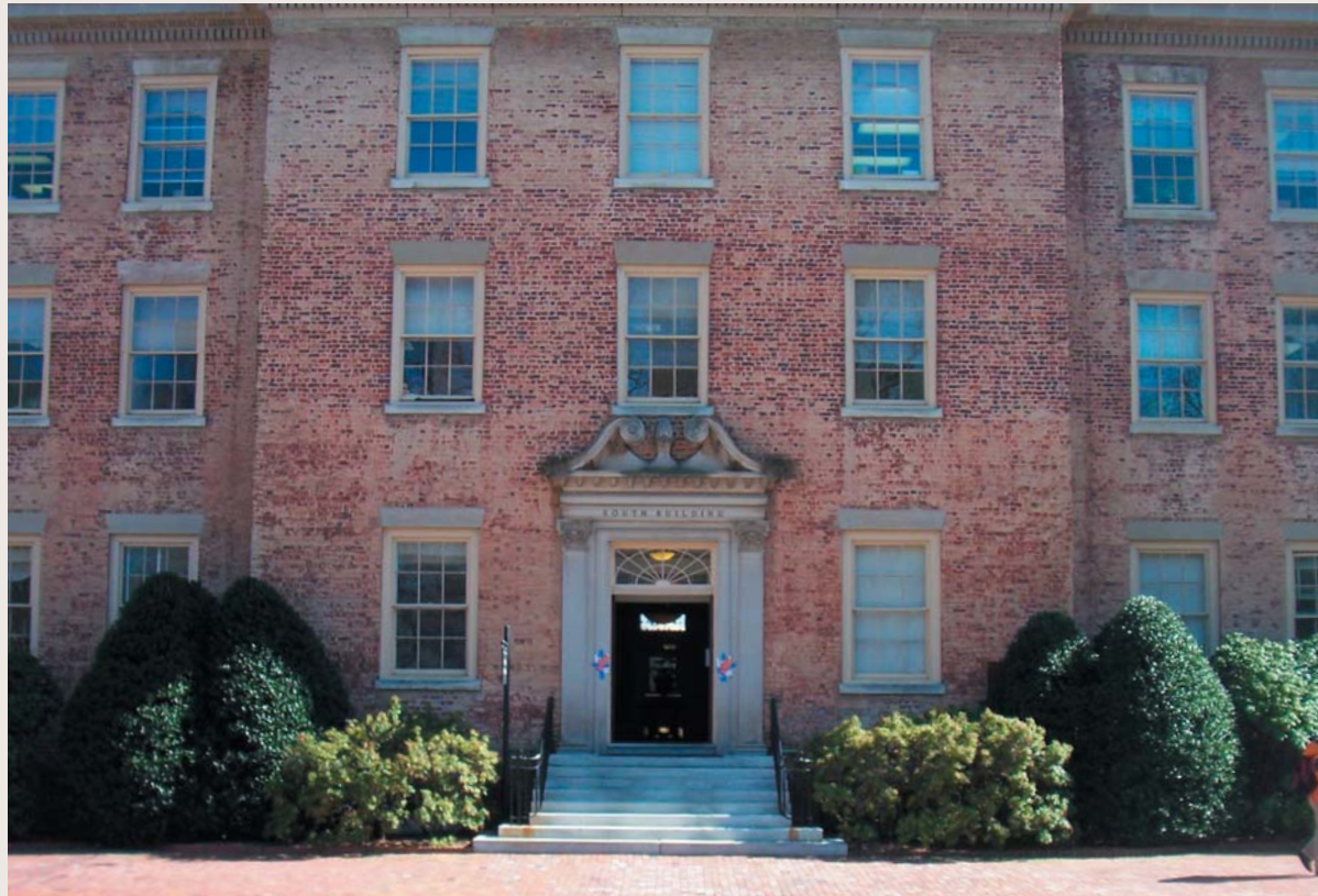
Foundation planting examples: Top: South Building, UNC Campus Bottom: Old West Building, UNC Campus
