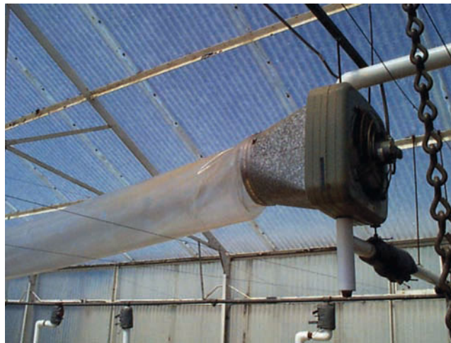
FIGURE 19-13. Use of a convection tube ensures even distribution of heated air through the greenhouse. (Delmar/Cengage Learning. Photo by Steven Newman.)
