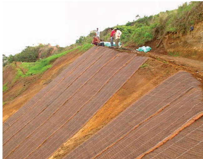
FIGURE 13-11. Erosion netting and mulch permit this newly seeded slope to develop a strong turf planting. Without the mulch and netting, the seed would wash away before becoming established. ( Courtesy United States Department of Agriculture )
