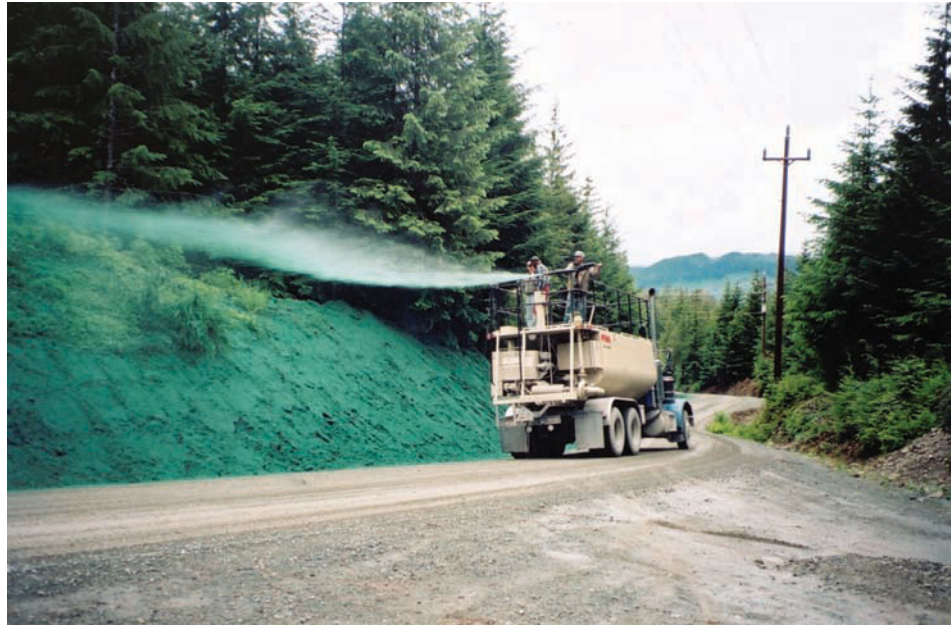
FIGURE 13-4. Use of the Hydroseeder gives rapid stabilization to this steep embankment. (Courtesy United States Department of Agriculture)
