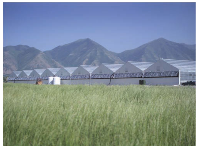
FIGURE 19–2. A typical ridge and furrow, A-frame, truss greenhouse range (Delmar/Cengage Learning. Photo by Steven Newman.)
