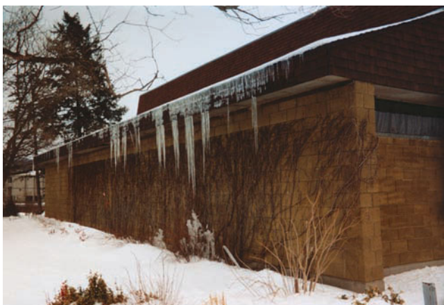
FIGURE 11–20. Falling ice can split and break shrubs planted beneath the overhang of a roof. (Delmar/Cengage Learning)
