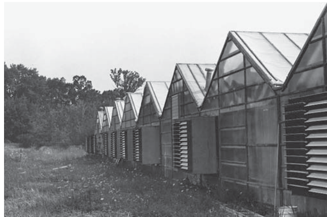
FIGURE 19–16B. These fans at the opposite end of the greenhouses pull the outside air through the pads. (Delmar/Cengage Learning. Photo by Jack Ingels.)
