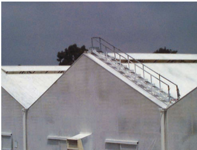
FIGURE 19–14. Shading is applied to lower the temperature. Sections can be left unshaded for crops requiring high light intensity. ( Delmar/Cengage Learning )
