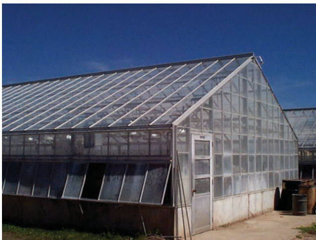
FIGURE 19–1. A detached A-frame truss greenhouse (Delmar/Cengage Learning. Photo by Steven Newman.)
