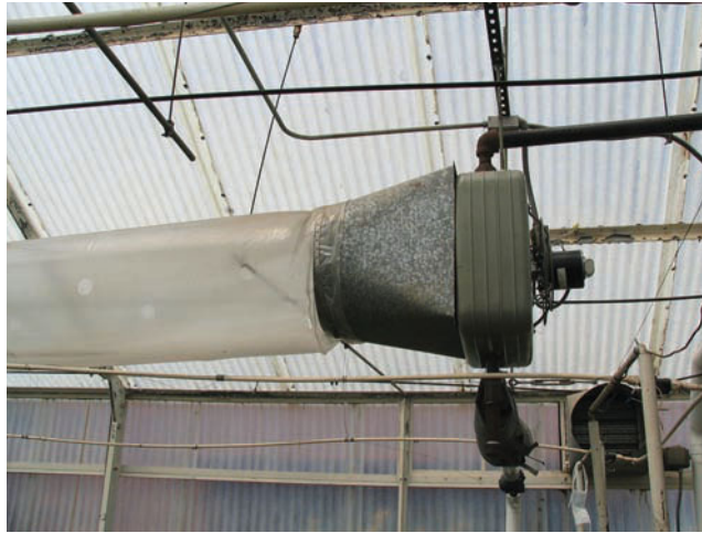
FIGURE 19–10. Fan jet ventilation and heating unit blows hot air toward the central circulation fan (Delmar/Cengage Learning. Photo by Steven Newman.)
