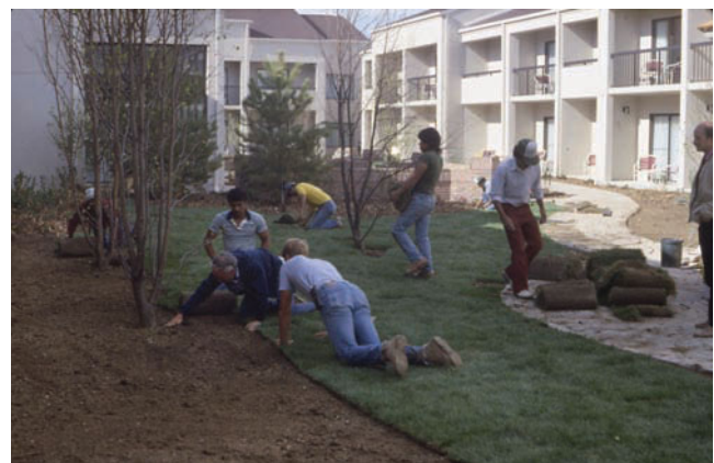
FIGURE 13-6. After careful preparation of the soil, the sod is unrolled at the site of the new lawn. (Delmar/Cengage Learning)
