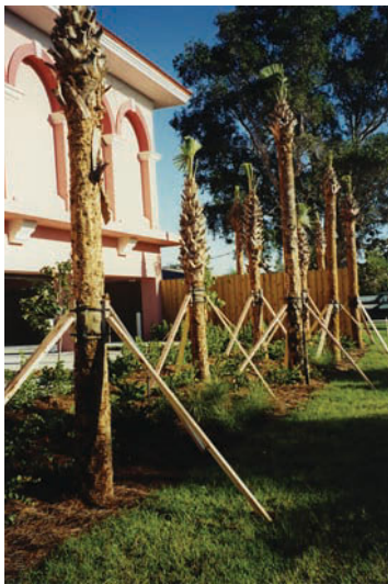
FIGURE 10-17. Exterior bracing supports the palms. Protective banding prevents injury where braces meet the trunks. (Delmar/Cengage Learning. Photo by Jack Ingels.)
