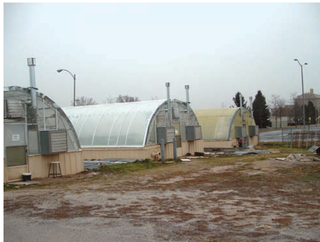
FIGURE 19–3. A quonset-style greenhouse (Delmar/Cengage Learning. Photo by Steven Newman.)
