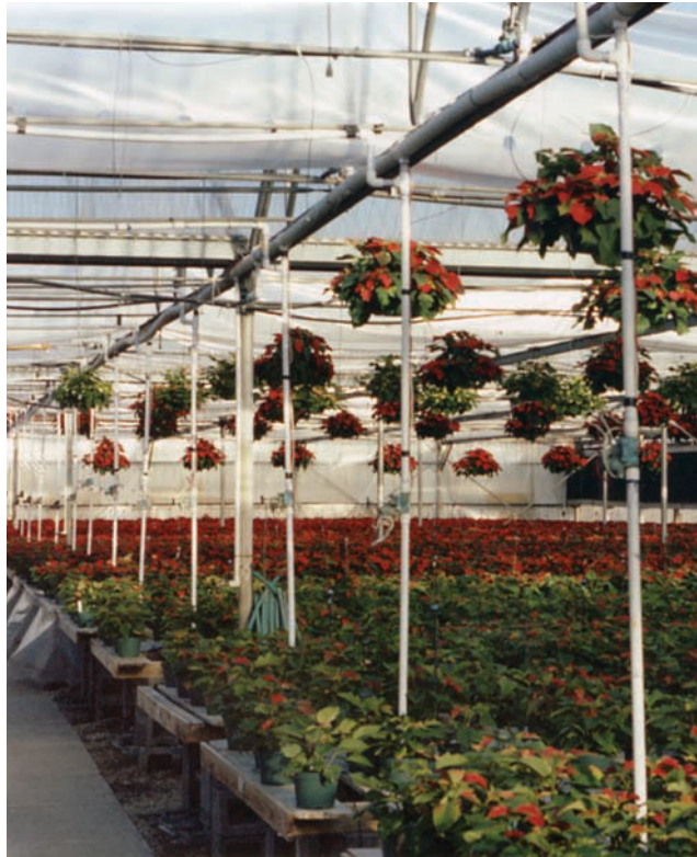
FIGURE 19–20. This photo illustrates the pipe frame. (Delmar/Cengage Learning. Photo by Jack Ingels.)
