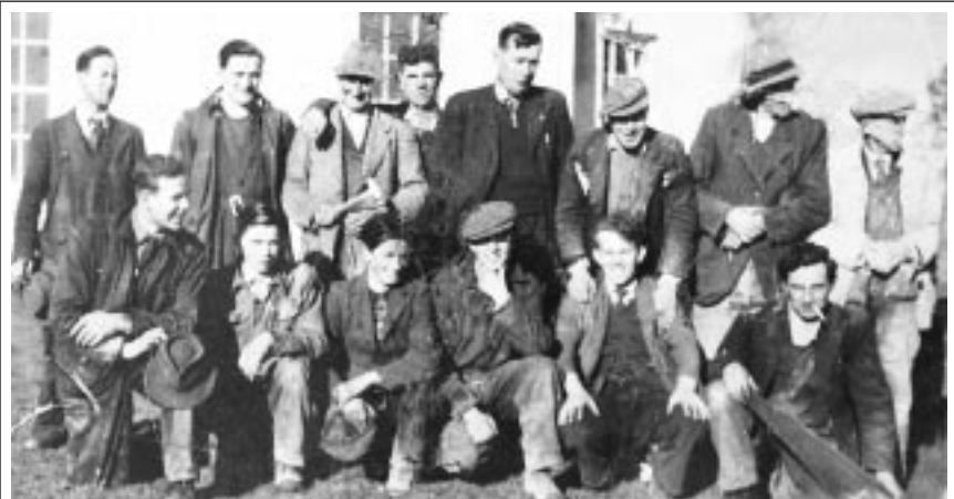
Ardsallagh House c.1951, renovations of house by contractor Laurence Kenny, The Green. Front: Mattie Kavanagh (Clonmel), Dick Fitzgerald, Tom McCormack (Annsgift), Mick McCormack (Annsgift), Johnny Jacobs (Waterford), Johnny Littleton. Back: Dick (Reidy) Power, Tom Burke (Coolmoyne), Tommy Kenny (Baptistgrange), Paddy Fitzgerald, Employee of Jacobs (Waterford), Bill 'Uncle' Connors, Dan McCarthy (Coolmoyne), Tom Finn (Burke Street).
