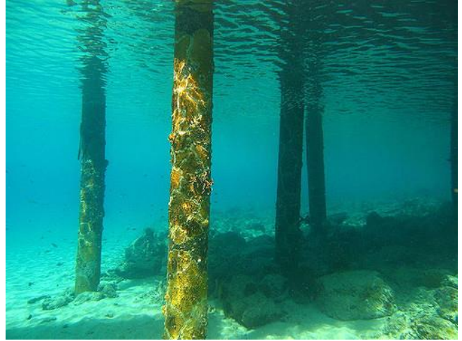
Coastal waters – under pier
