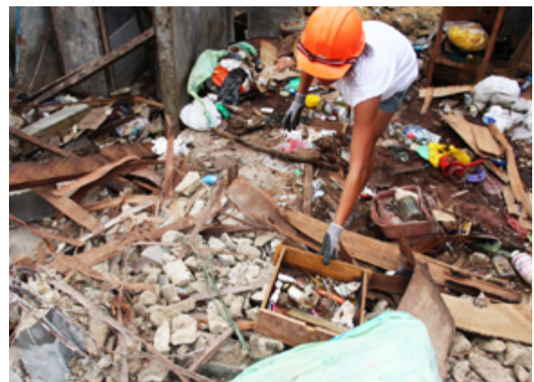
Debris and mess created by the earthquake Flickr / All Hands Volunteers Photobank
