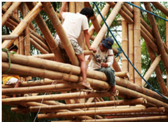
Filipinos working at the construction site Flickr / Andrea Fitrianto
