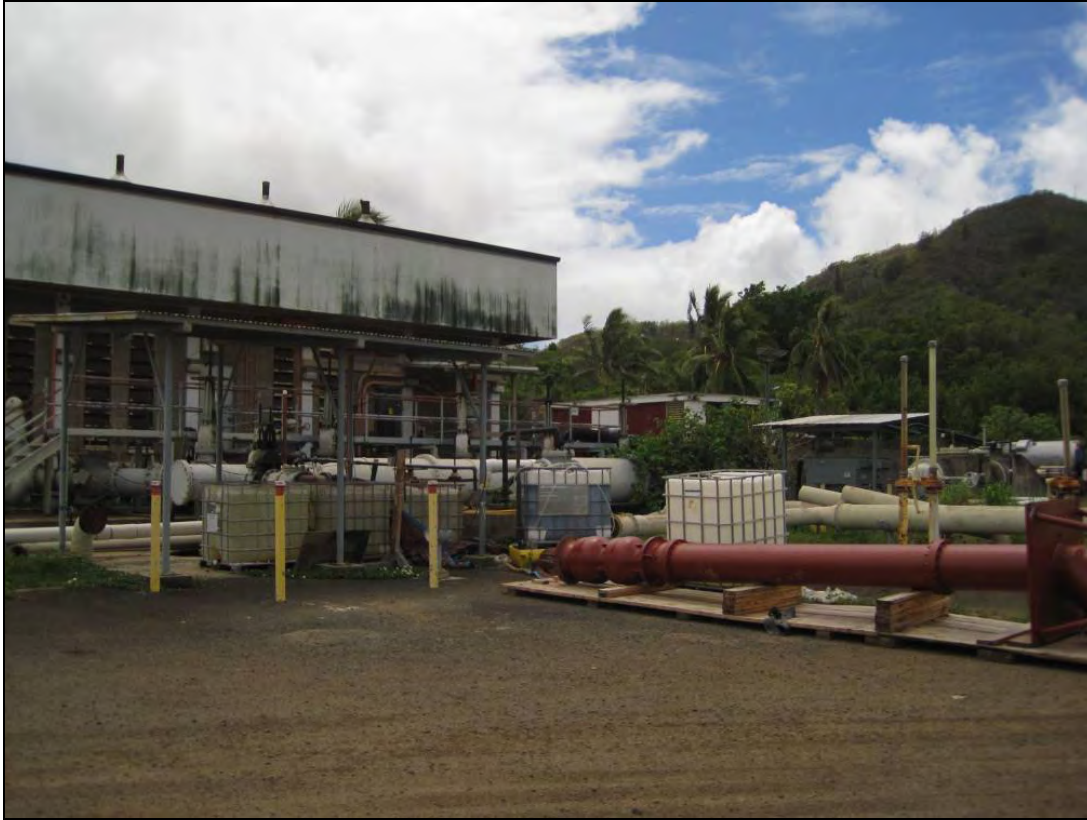
Figure 30. Buildings and piping within eastern portion of WWPTF, view to southeast
