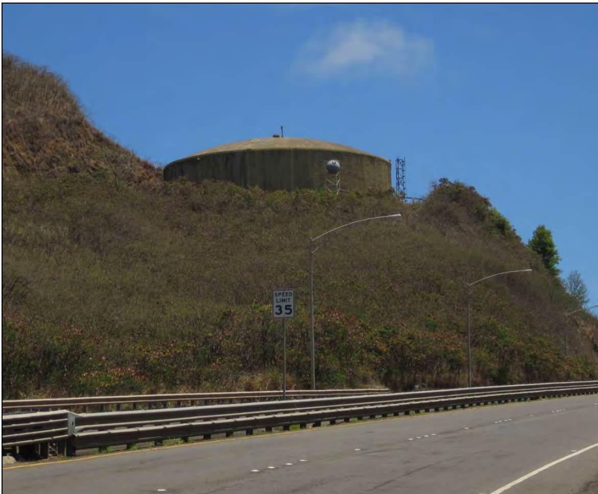
Figure 49. Photograph showing location of water tank within the BWS property and location of proposed intermediate tunnel access shaft, Mōkapu Saddle Road in foreground, view to north
