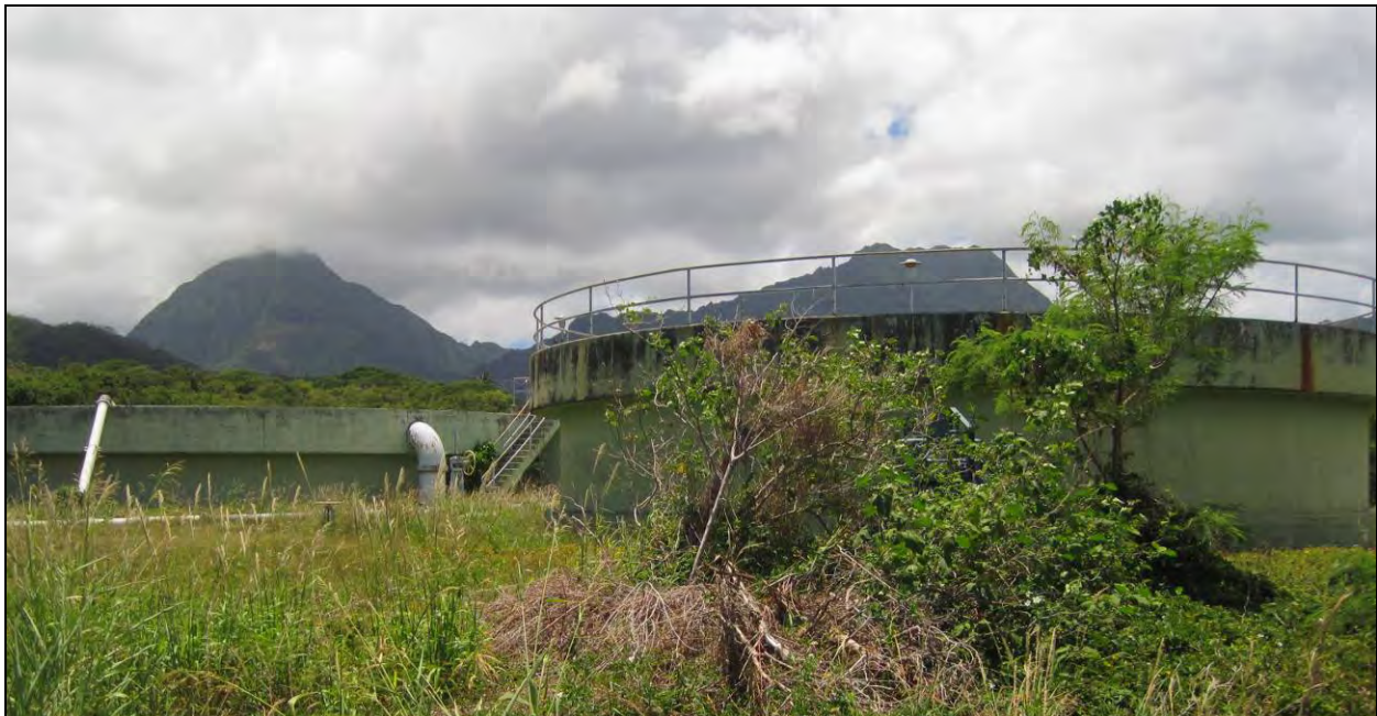
Figure 27. Photograph showing large holding tanks where improvements are planned in south central portion of the Kāneʻohe WWPTF, view to southeast
