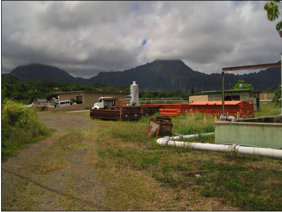
Figure 32. Photograph showing development in eastern portion of WWPTF, view to southeast
