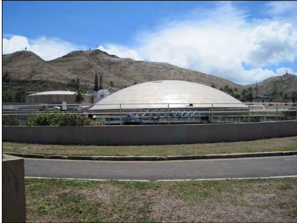
Figure 47. Overview showing location of “Facility 7” at the Kailua WWTP, view to southwest This is also the most likely location of the dewatering facility.
