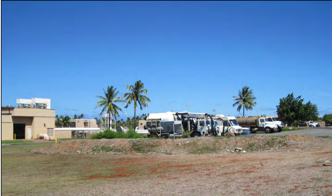
Figure 37. Overview showing proposed location of flow equalization basin at the Kailua WWTP, view to southeast (also shown on aerial, Figure 33 and a second photograph Figure 43)
