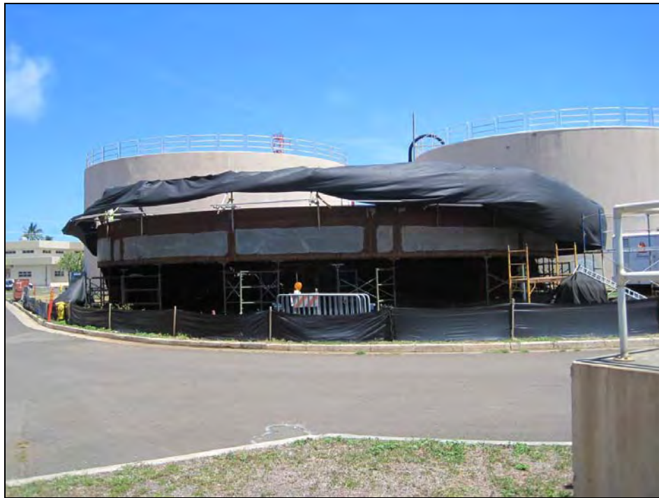
Figure 40. Site location Alternative C at the Kailua WWTP, view to east
