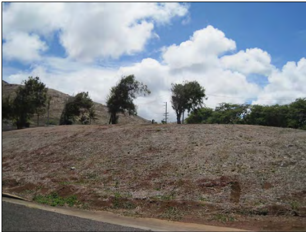
Figure 42. Overview showing location of “Facility 2” at the Kailua WWTP, view to west
