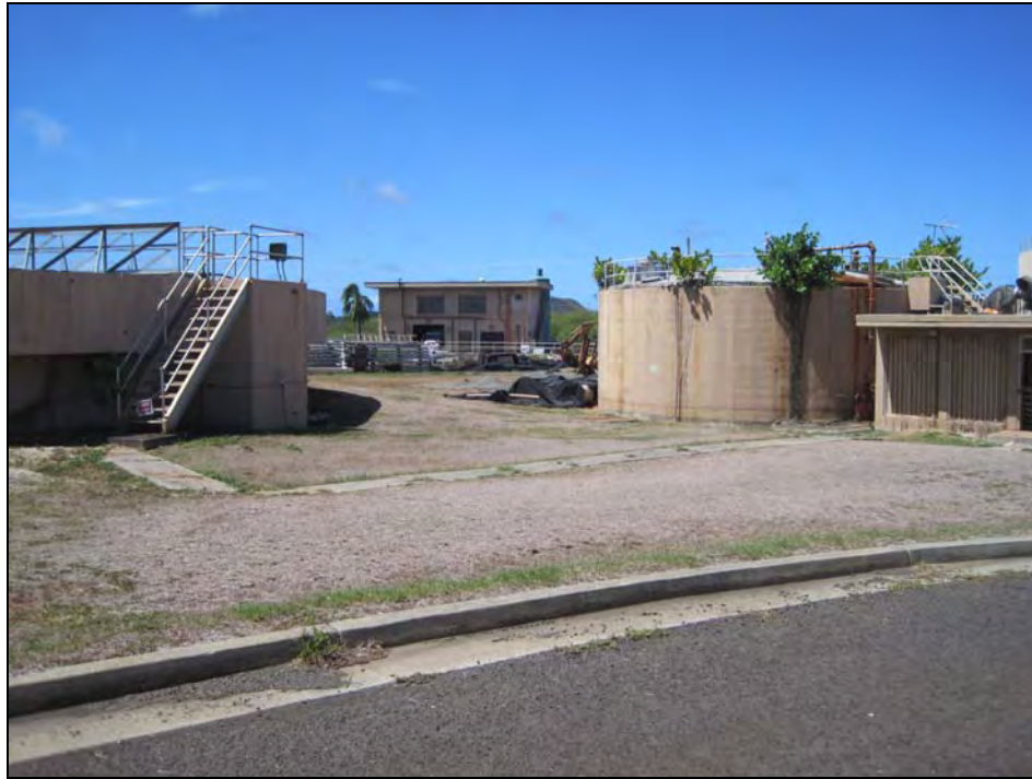
Figure 45. Overview showing location of “Facility 5” at the Kailua WWTP, view to northwest
