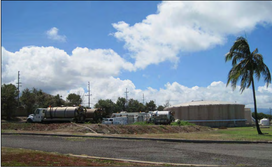
Figure 43. Overview showing location of “Facility 3” at the Kailua WWTP, view to southwest. Note that mounded area consists of compacted soil and debris. This location is also proposed for the equalization basin (see Figure 33).
