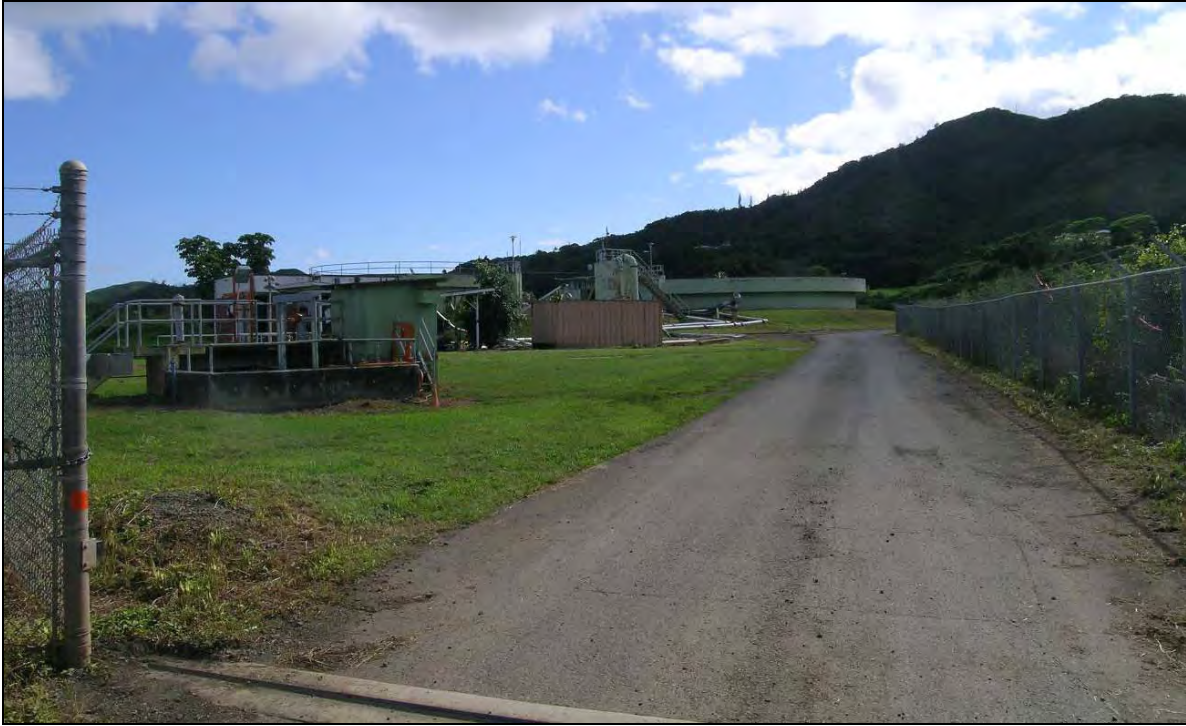
Figure 24. Entrance to the Kāneʻohe WWPTF, showing chain link fencing along southern boundary to right and existing tanks where improvements are planned to left of asphalt paved roadway, view to southeast
