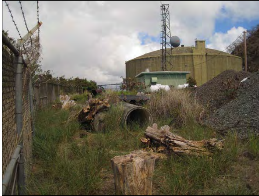
Figure 50. Photograph showing existing water tank, southern fenced boundary of parcel, BWS property at Mōkapu Saddle Road, showing construction debris, piping and gravel, view to west
