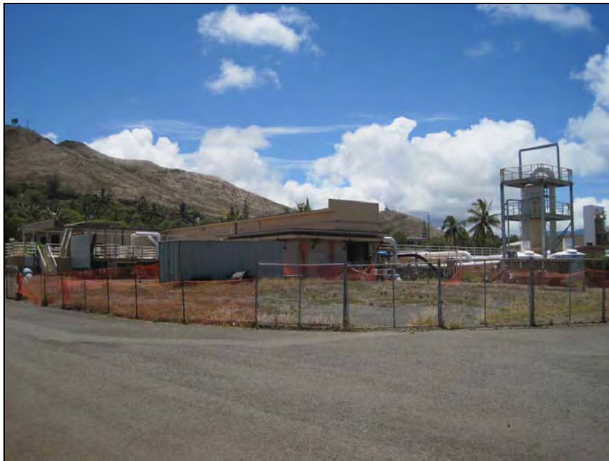
Figure 48. Overview showing location of “Facility 8” at the Kailua WWTP, view to southwest
