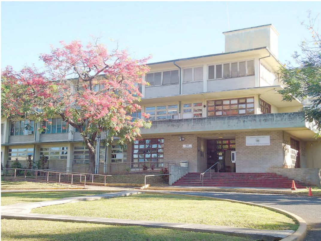
Hale Ola is eligible for listing on the National Register of Historic Places under Criteria “A” and “C” and possess the integrity required for eligibility.
