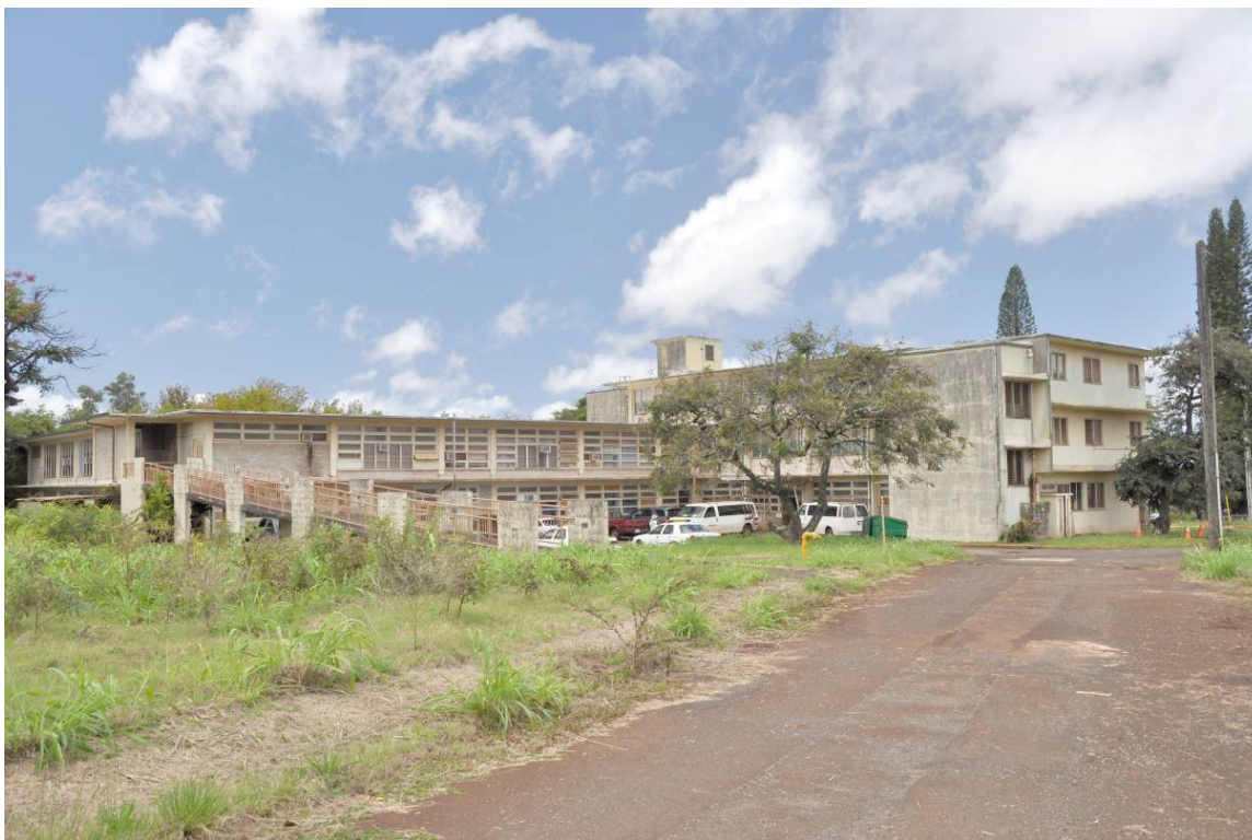
A two-story wing, as seen from the rear of the building
