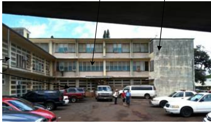
Back-side of Doctors Wing with 2-Story Addition (ca 2013)
