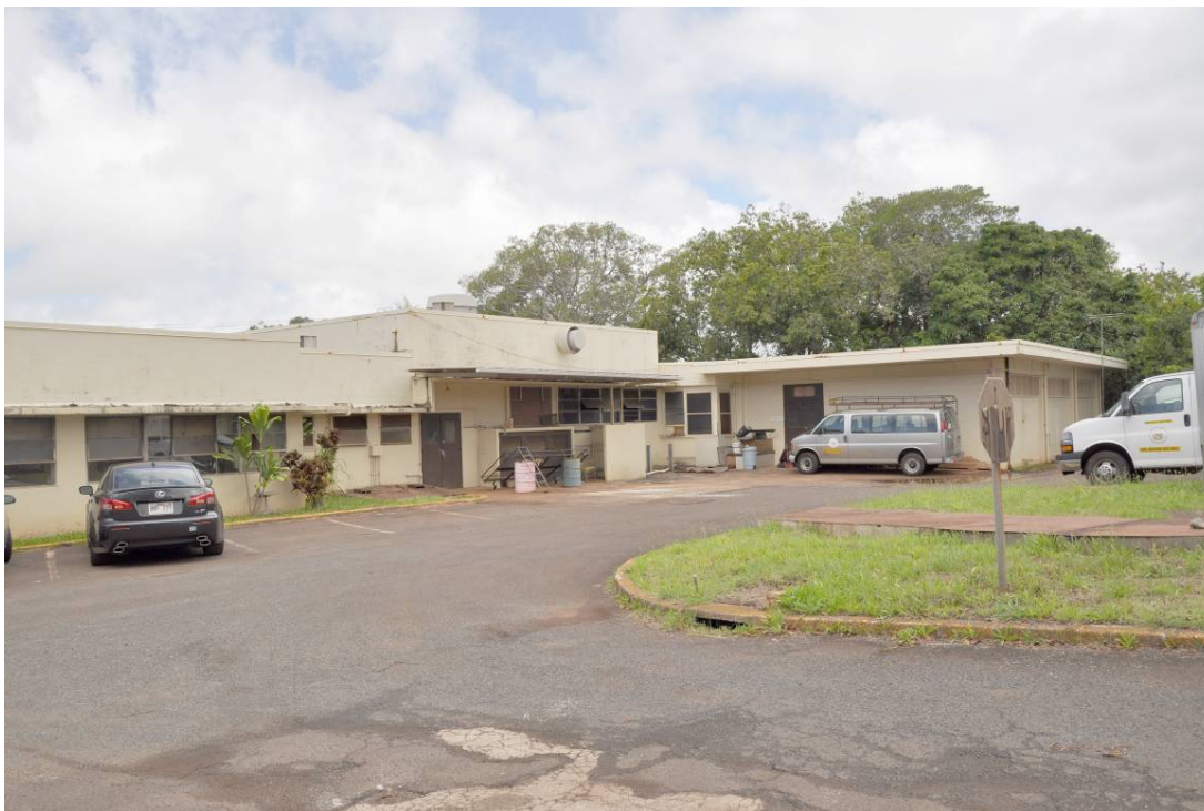
The former kitchen and dining building will provide conference rooms and offices for the DOH Clean Water Branch.
