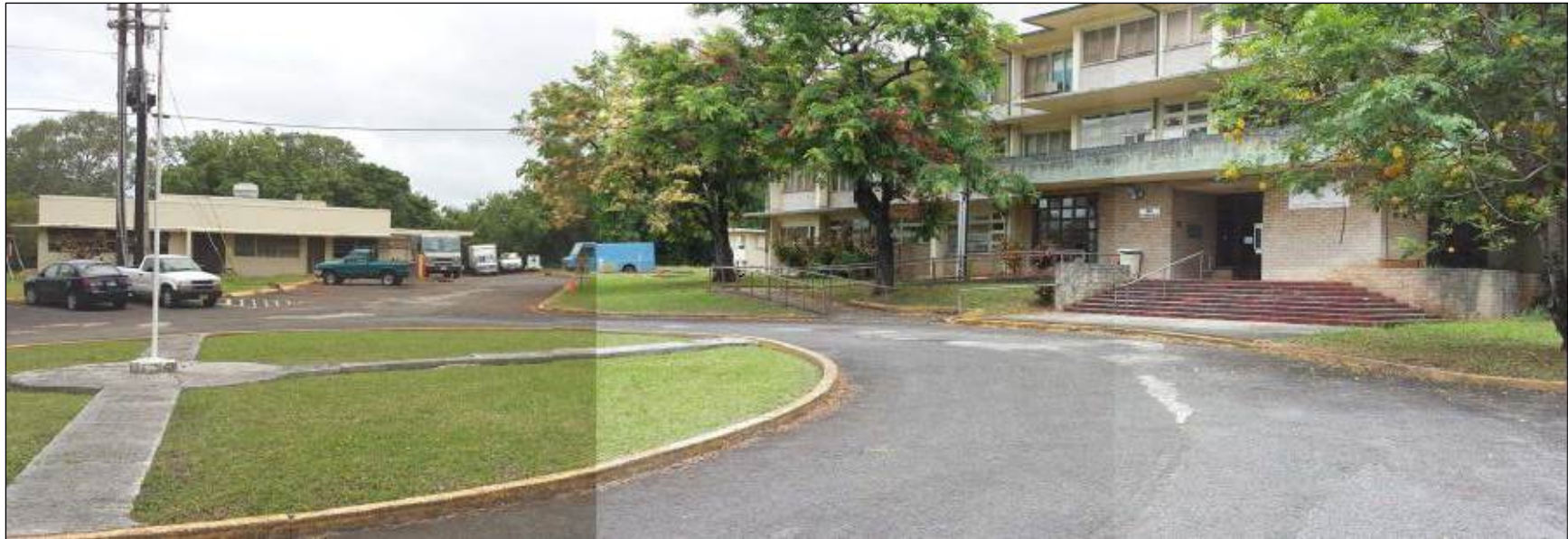
Figure 19. Stitched photos showing the Hospital Building at right and the Kitchen and Dining Building at left; view to the north
