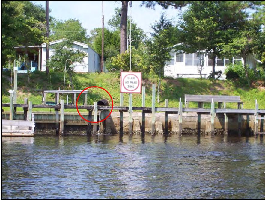
Photograph 3-7: Stormwater pipe discharging into the Lockwoods Folly River.
