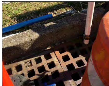
Photo of the bypass pumping of storm drain receiving sanitary waste
