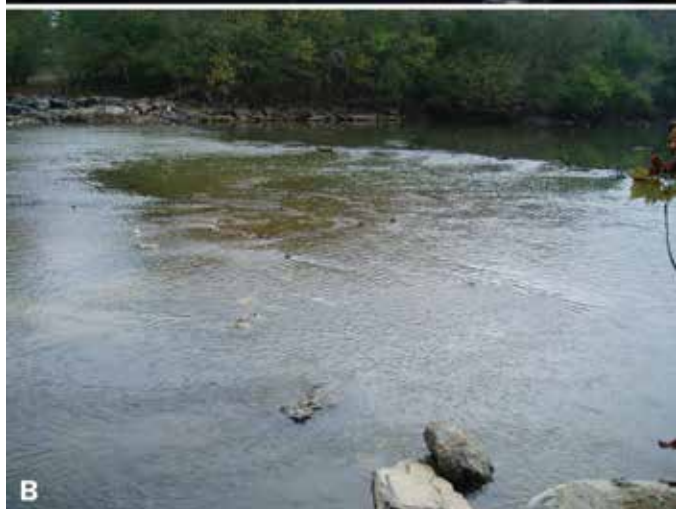
Figure 6. (A) Former Marvel Bridge located in the Cahaba River north of the Cahaba National Wildlife Refuge. The bridge (slab) was constructed by a mining company in the 1970s to move coal across the river and remained after the mine closed. (B) Efforts by the Nature Conservancy of Alabama culminated in its removal in late 2004, which improved habitat conditions over a kilometer of river and eliminated a barrier to fish passage. Photo Credit: Paul Freeman, the Nature Conservancy of Alabama.
