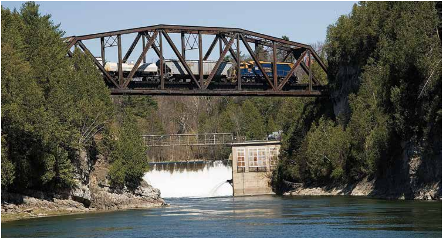
Winooski hydro station
