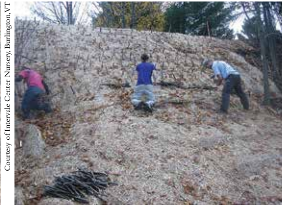
These two photographs show a bank restoration in Isle LaMotte on Lake Champlain in the fall of 2010 with about 500 live stakes. The live stakes were collected a day or two before planting to ensure the viability of the plant material and offer a natural way to combat erosion. Many sites need preparation involving excavation or earth removal to shape the bank before plantings are introduced.
