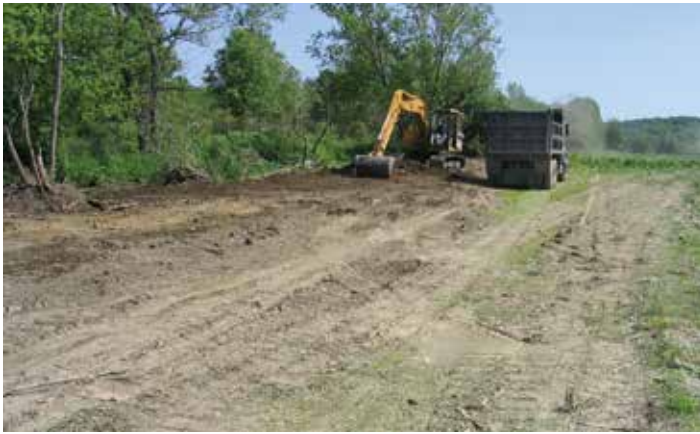
Removal of a berm or embankment along a river.
