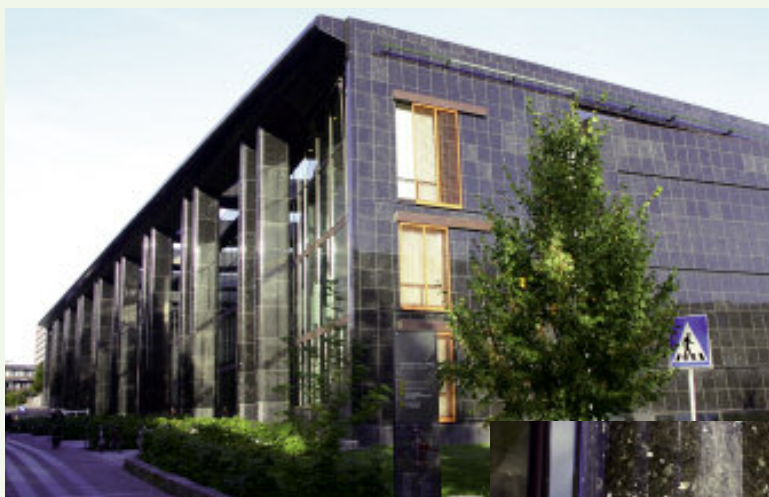
University of Oslo (UiO) Library at Blindern, an impressive building faced with larvikite. (Photo: B. T. Larsen)
