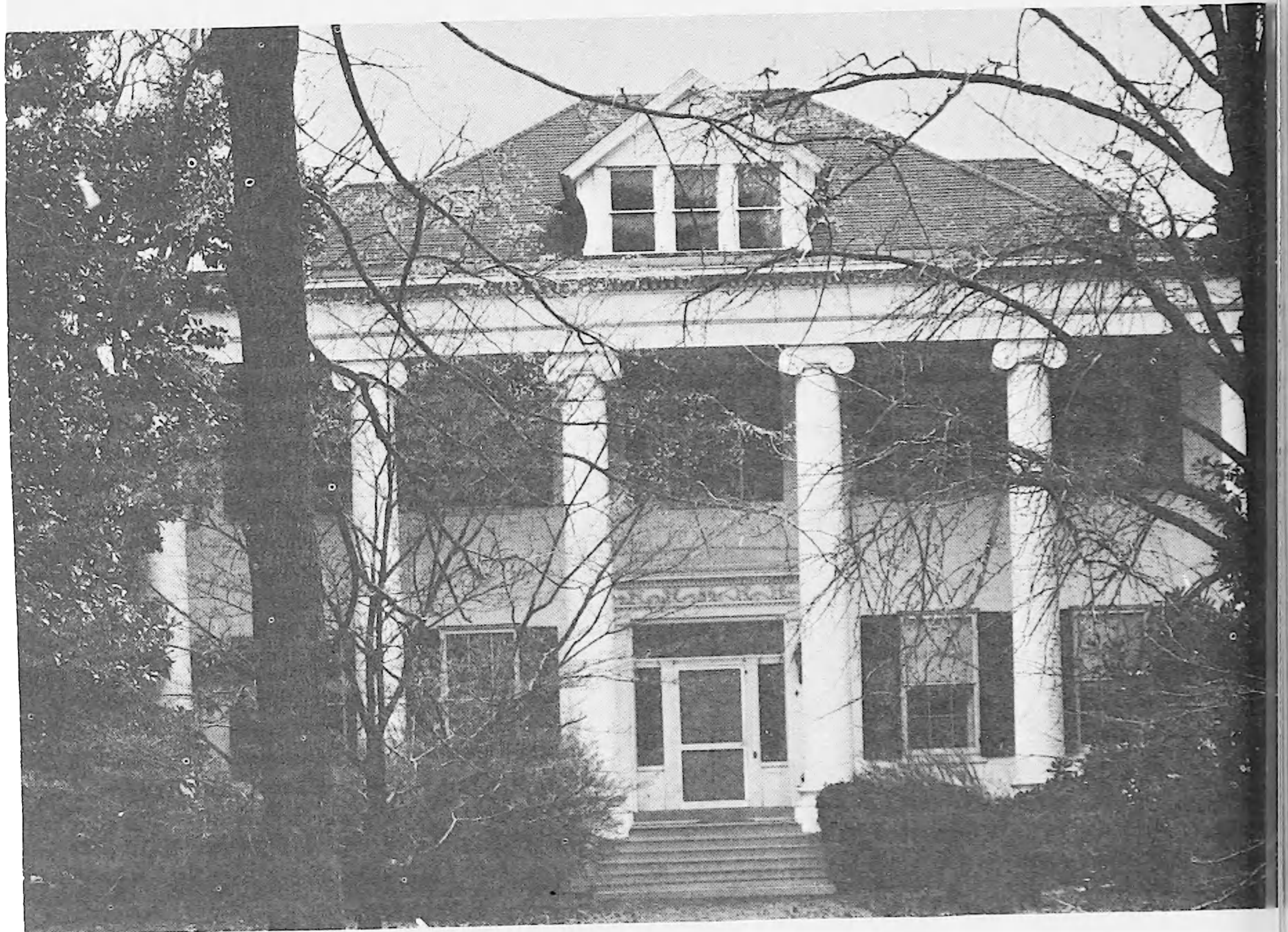
Pike-Fletcher-Terry House (Albert Pike House), Little Rock, Arkansas (Pulaski County). HABS. Arkansas Historic Preservation Program
