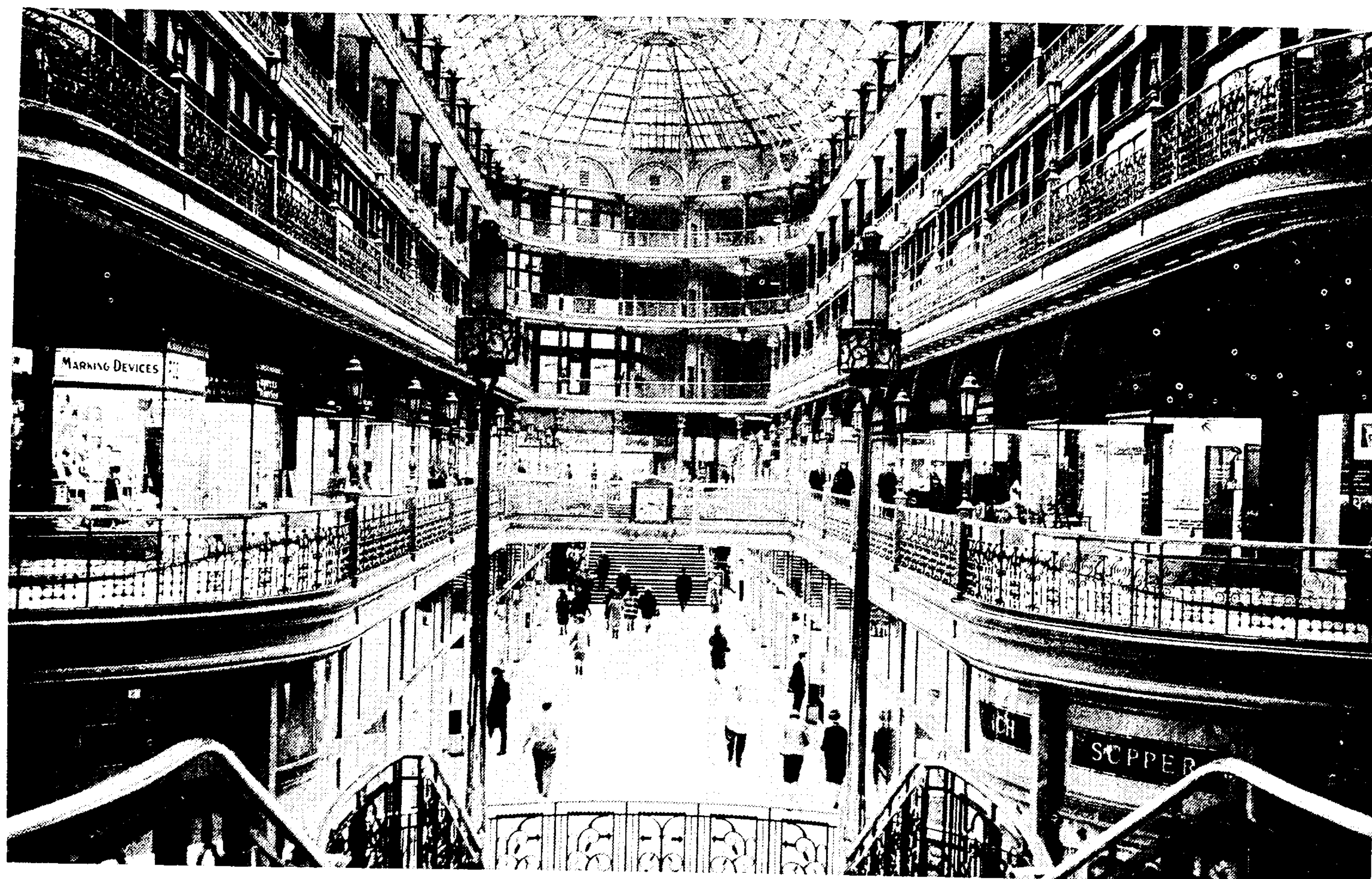
Cleveland Arcade, Cleveland, Ohio (Cuyahoga County). Martin Linsey for HABS
