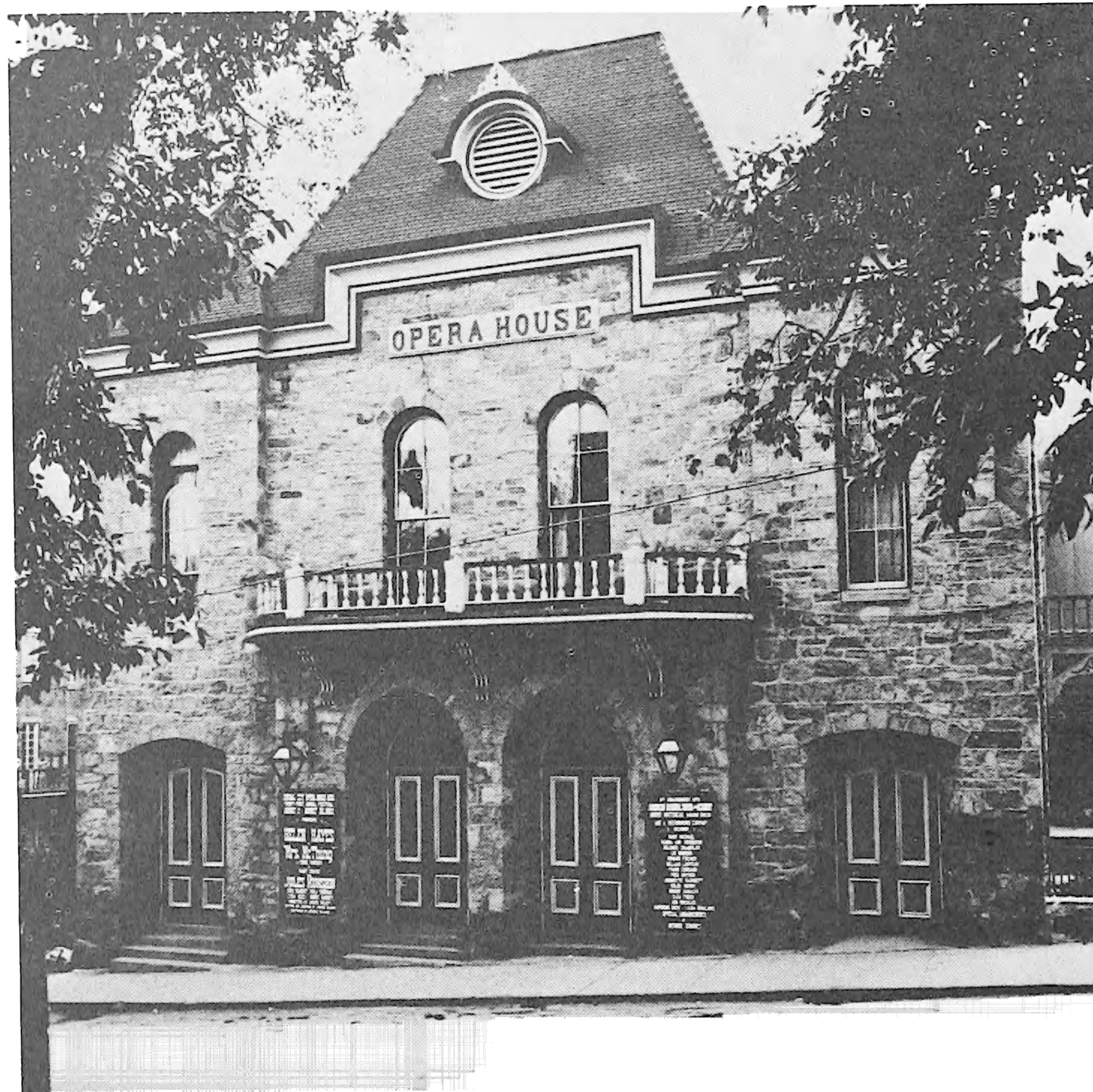
Central City Opera House, Central City, Colorado (Gilpin County). HABS. Central City Opera House Association
