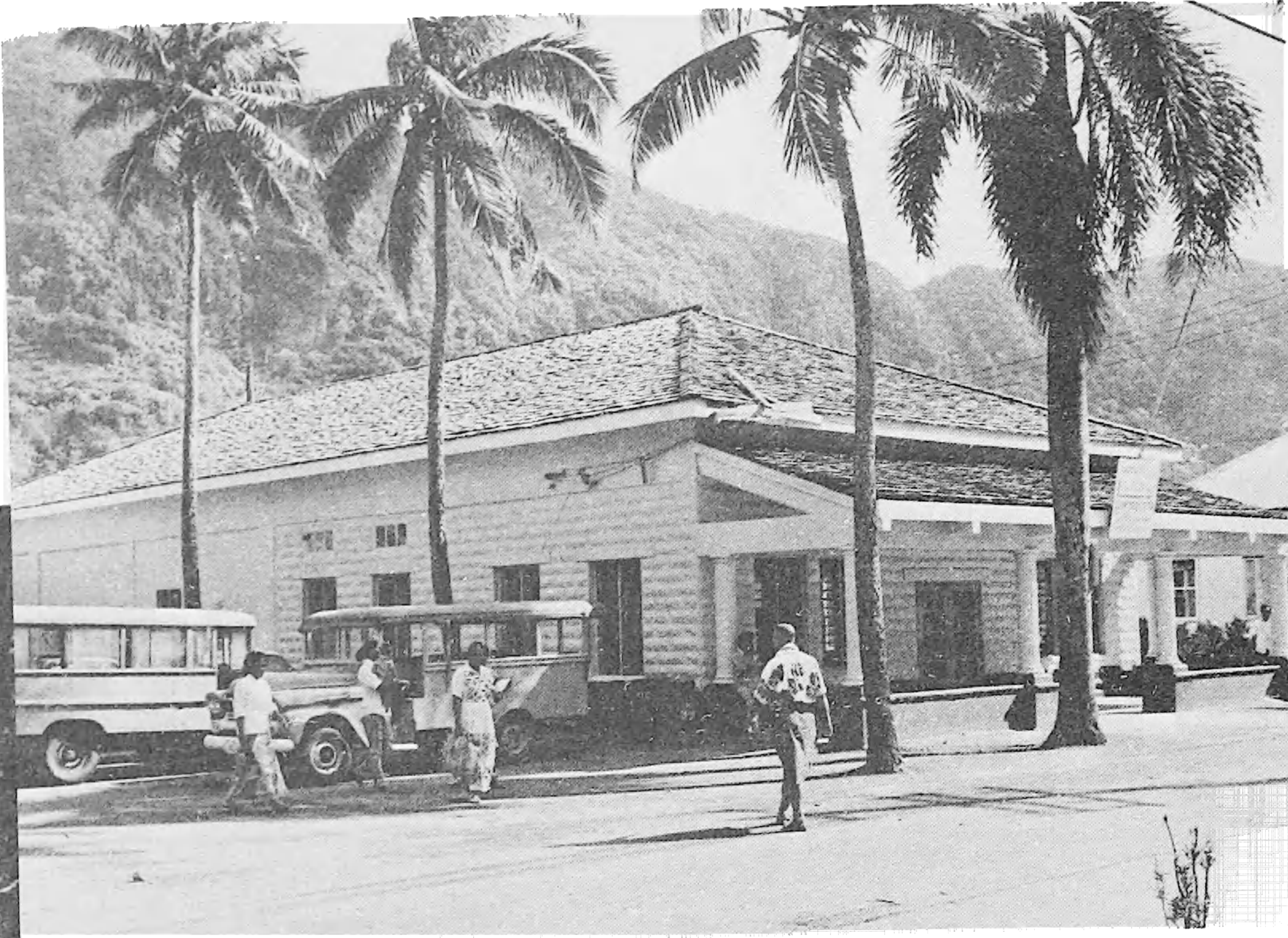
Navy Building 43 (Post Office and Commissary), Fagatogo, American Samoa (Eastern District). Dave Savé
