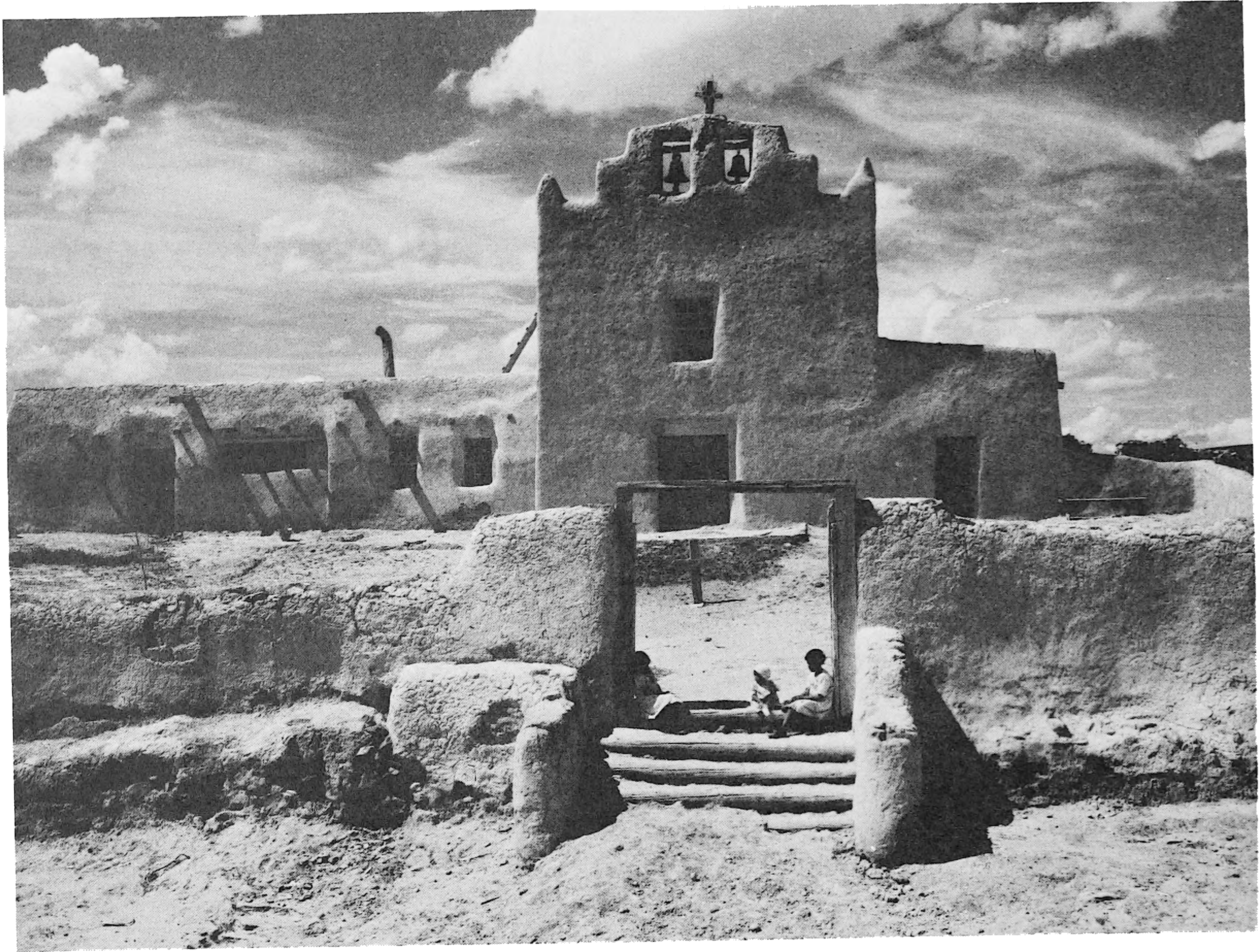
San Jose de la Laguna Mission and Convento (Old) Laguna Pueblo, New Mexico (Valencia County). HABS. Museum of New Mexico
