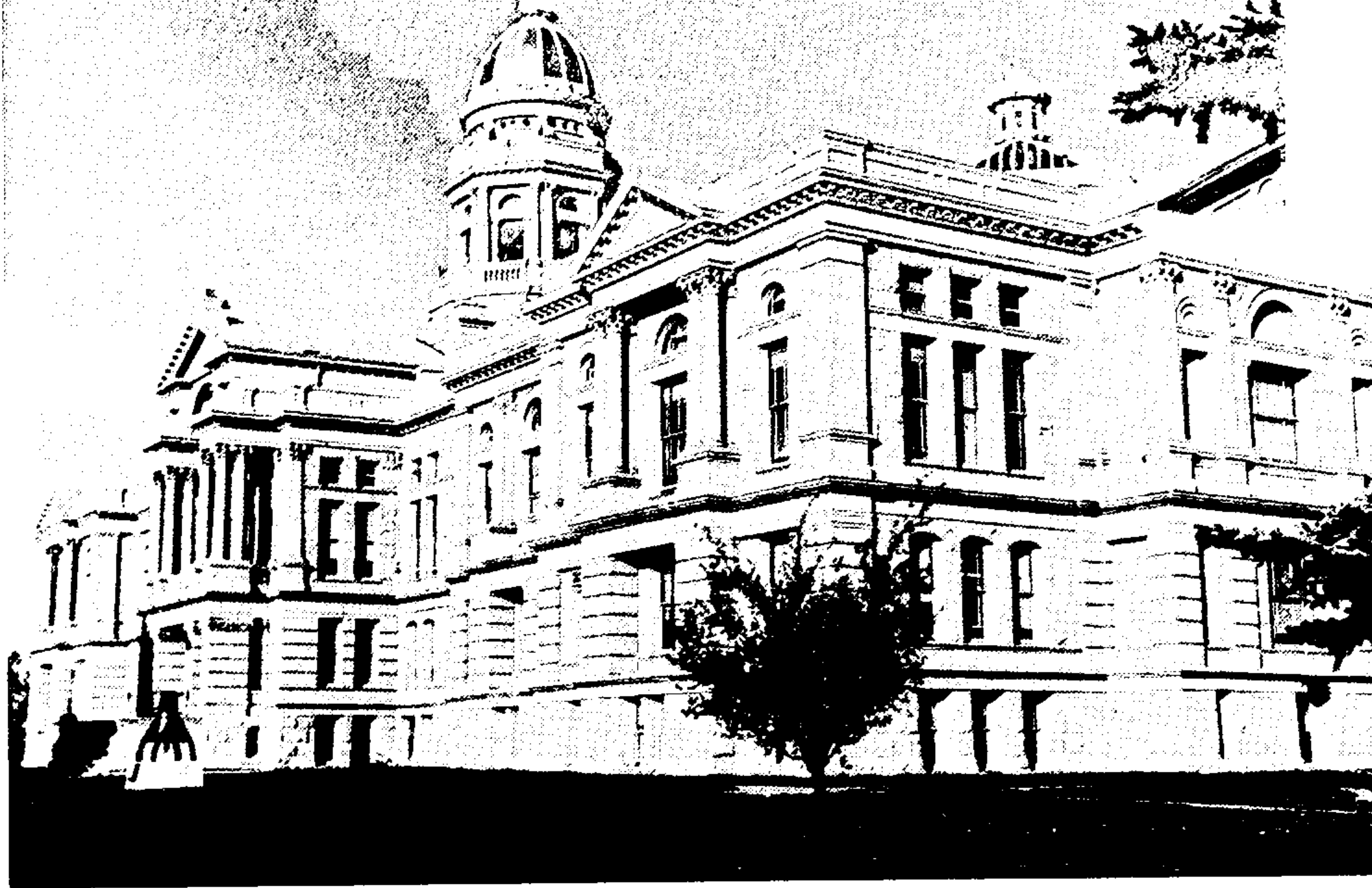
Wyoming State Capitol Building and Grounds, Cheyenne, Wyoming (Laramie County). Mark Junge
