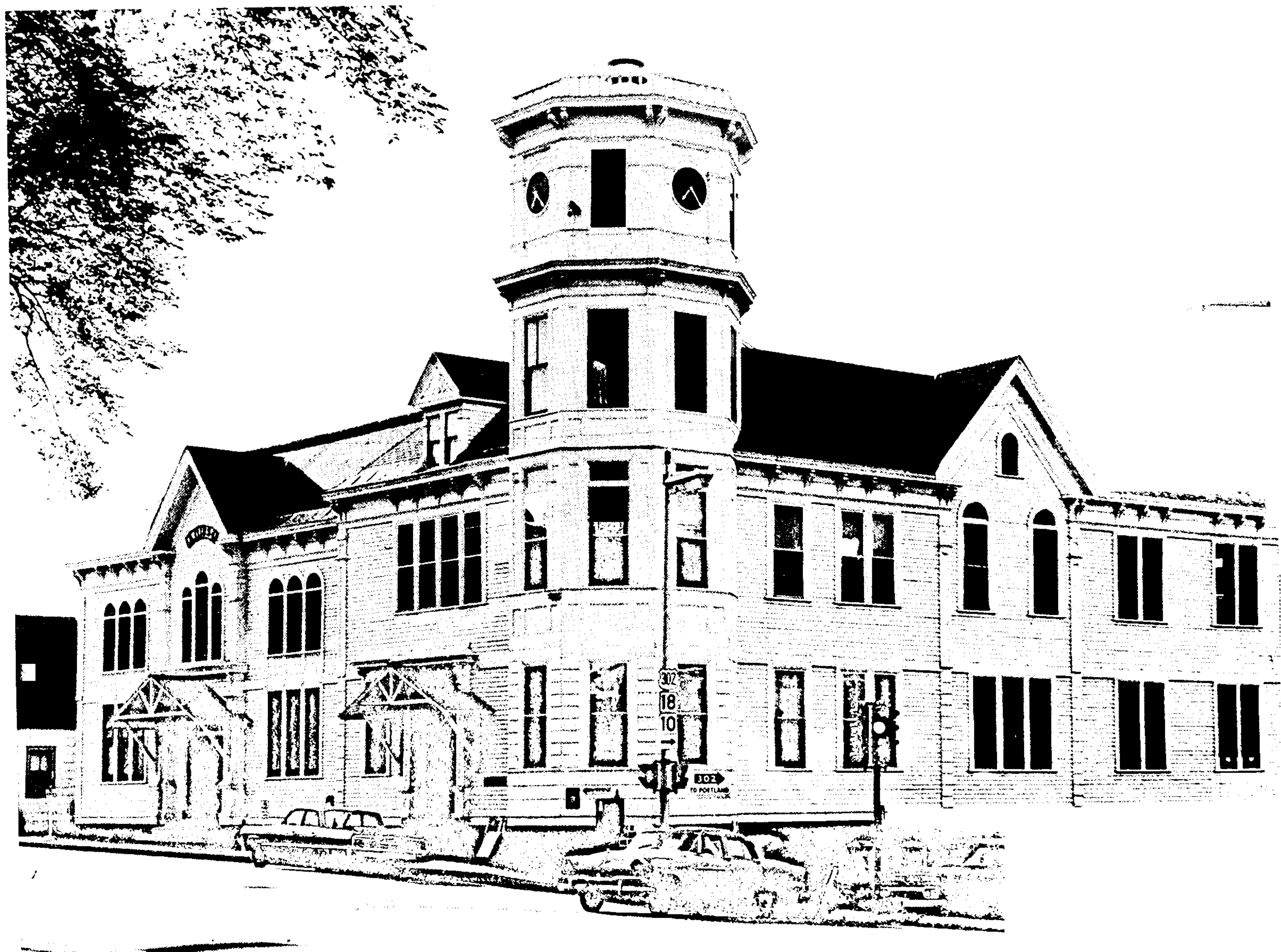
Littleton Town Building (Littleton Opera House), Littleton, New Hampshire (Grafton County). Lawrence H. Presby
