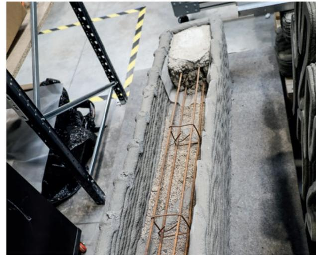
These days, you can print more than just buildings with concrete; segments of interior architecture are also possible (left), and rebar can be incorporated for additional stability (right)
