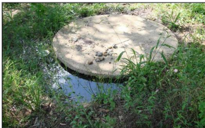
Figure 68 - Sewage from a failed septic tank 101
